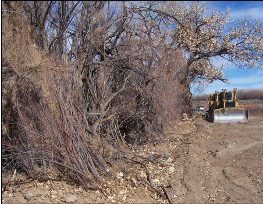
Figure 3. Dozing operations taking place in Socorro, New Mexico, in an area occupied by the invasive species saltcedar (Bureau of Reclamation photo).
