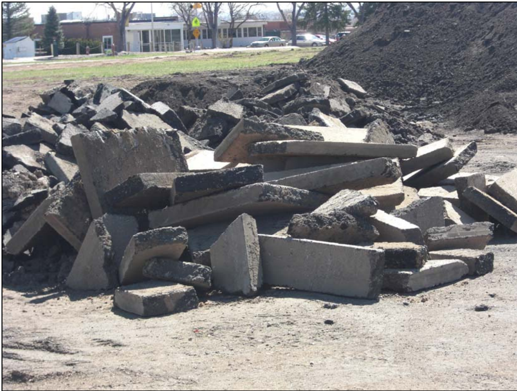
Figure A-3. Stockpiled broken concrete – note contact surfaces with adhering residue soils. These surfaces can harbor foreign species from the site of previous use (photo courtesy of Joe DiVittorio, 2010).
