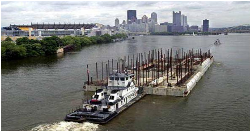
Transportation of Braddock Dam Module
