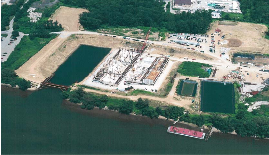
Graving Site for Braddock Dam
