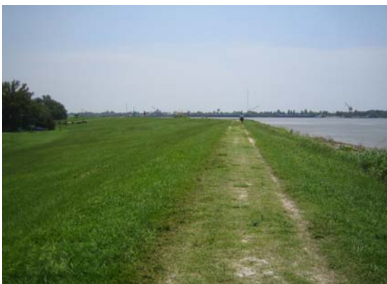
Photograph 5-8. Holy Cross levee with recreational trail.
