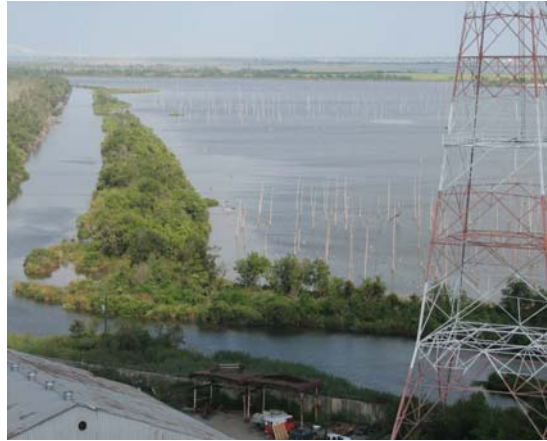
Photograph 5-5. Triangular-shaped wetland area located east of the IHNC and south of Bayou Bienvenue
