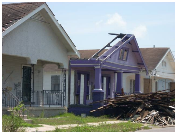
Photograph 5-3. Damaged houses in the study area.
