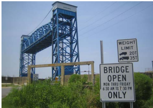
Photograph 4-2. Florida Avenue Bridge as viewed from the Lower Ninth Ward
