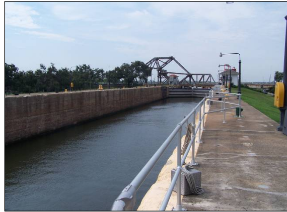
Photograph 3-1. Existing IHNC Lock
