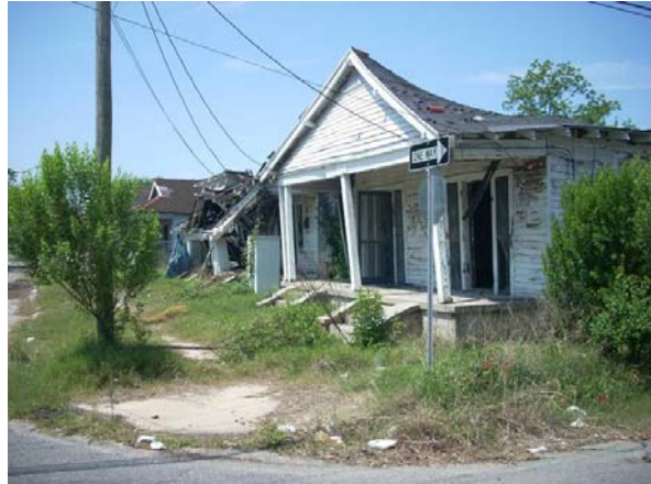
Photograph 5-1. Example of damaged residences located in the study area.
