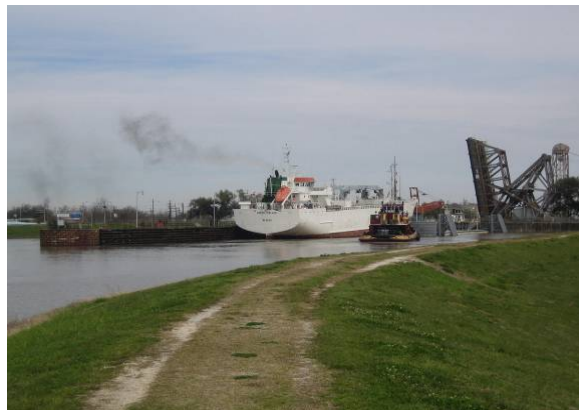
Photograph 4-5. Existing St. Claude Avenue Bridge; view of the bridge is from the south near the IHNC – Mississippi River confluence
