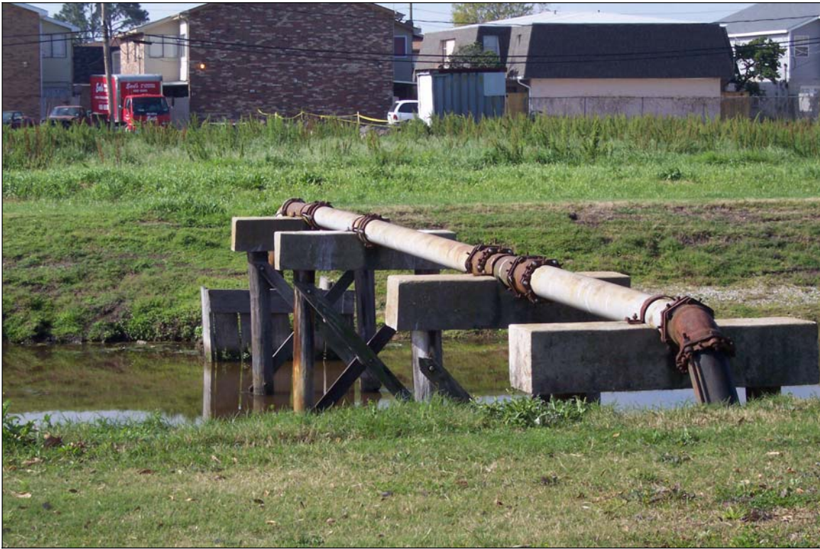
Photograph 5. Pipeline crossing project corridor
