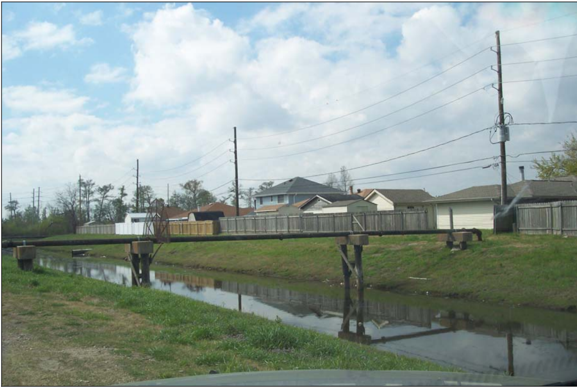
Photograph 11. Pipeline crossing project corridor
