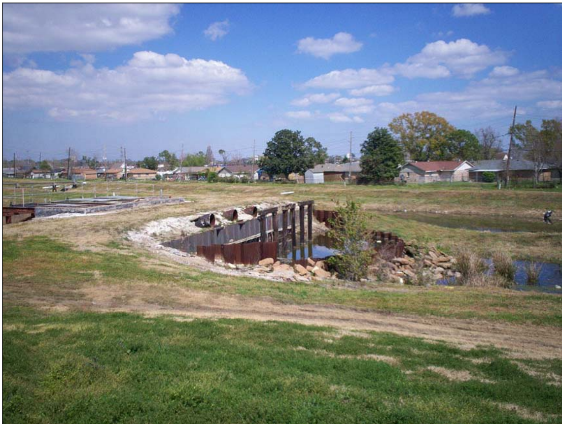
Photograph 3. Bridge and structure foundation adjacent to project corridor
