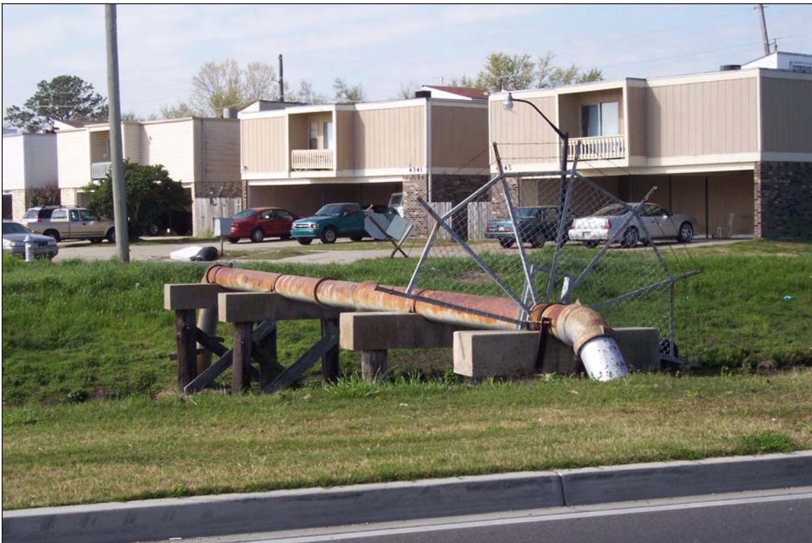
Photograph 6. Pipeline crossing project corridor
