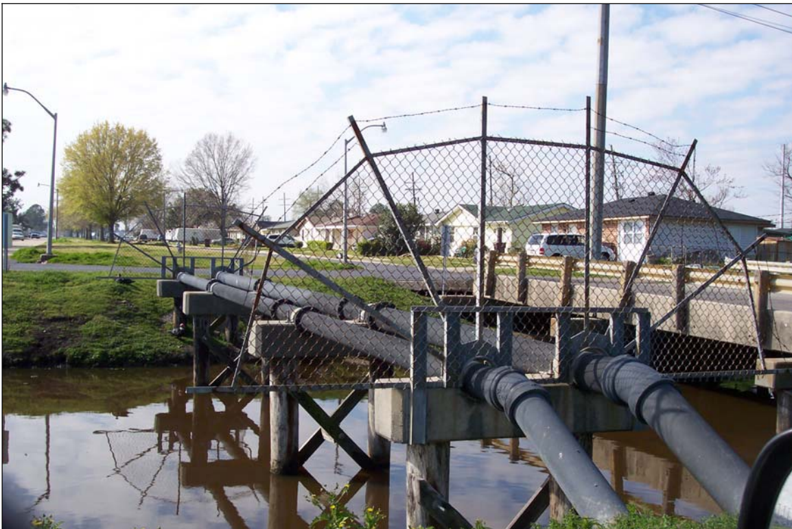
Photograph 8. Pipeline crossing project corridor
