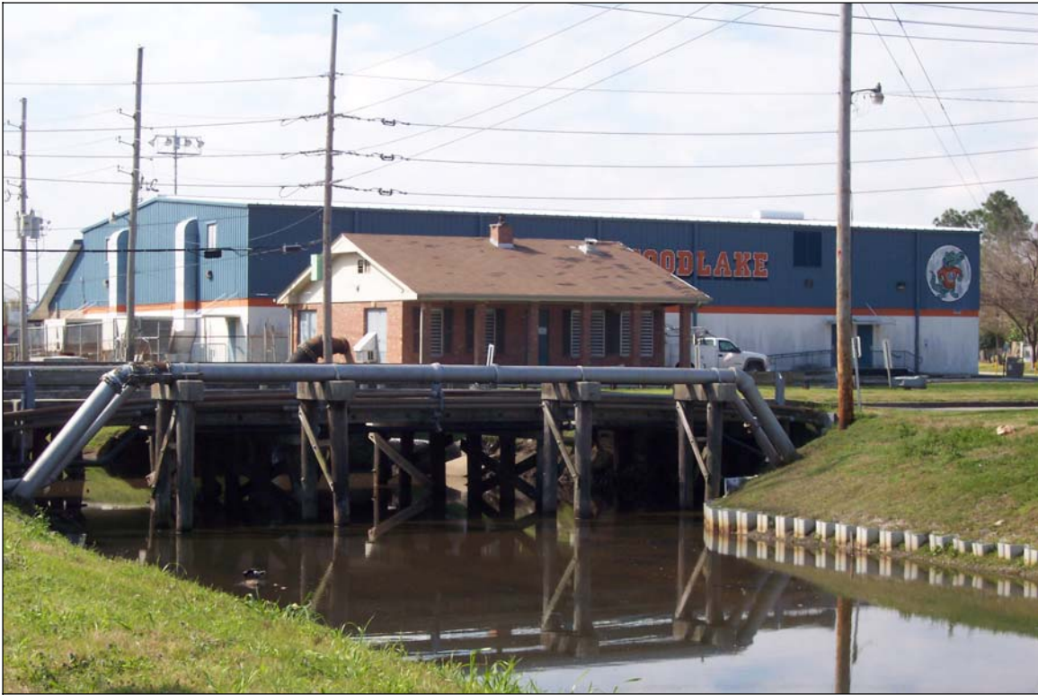
Photograph 12. Pipeline crossing project corridor
