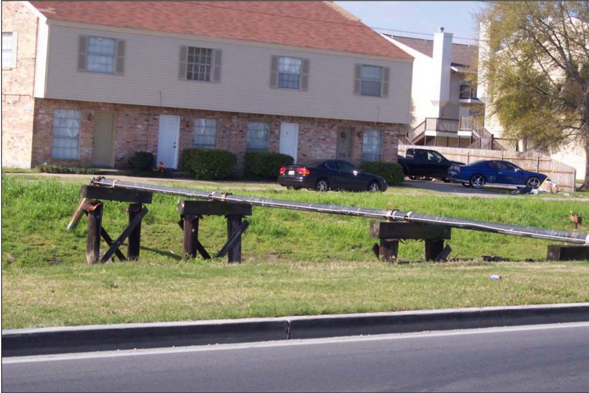
Photograph 1. Pipeline crossing project corridor
