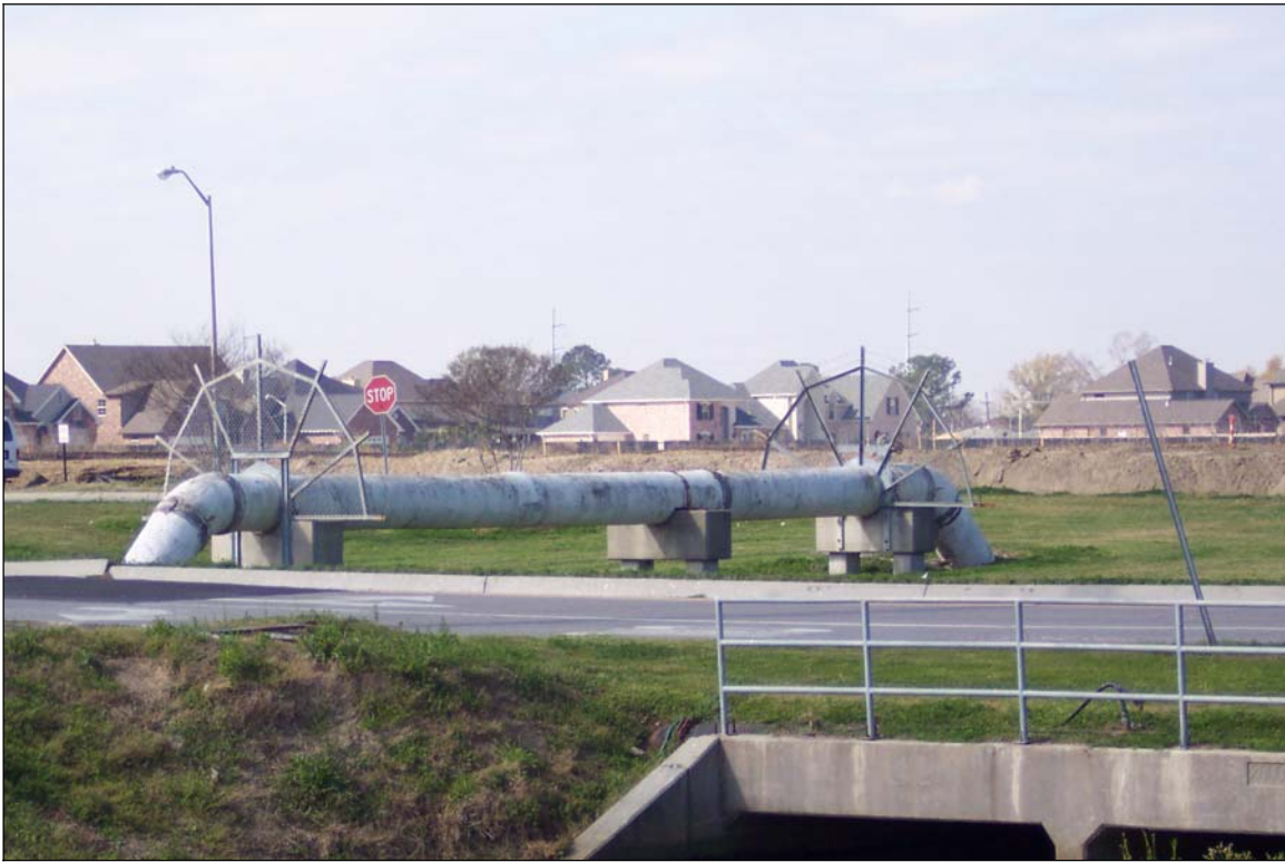
Photograph 7. Pipeline crossing project corridor
