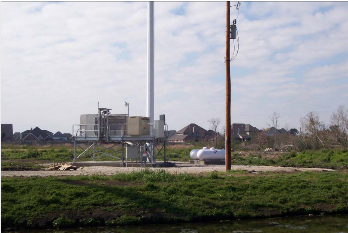
Photograph 17. Cell tower and generator adjacent to project corridor
