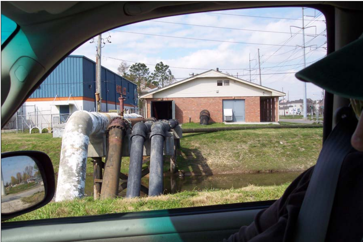
Photograph 13. Wastewater pump station and pipelines adjacent to project corridor
