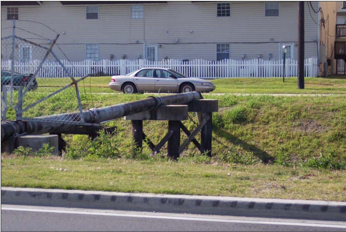
Photograph 3. Pipeline crossing project corridor
