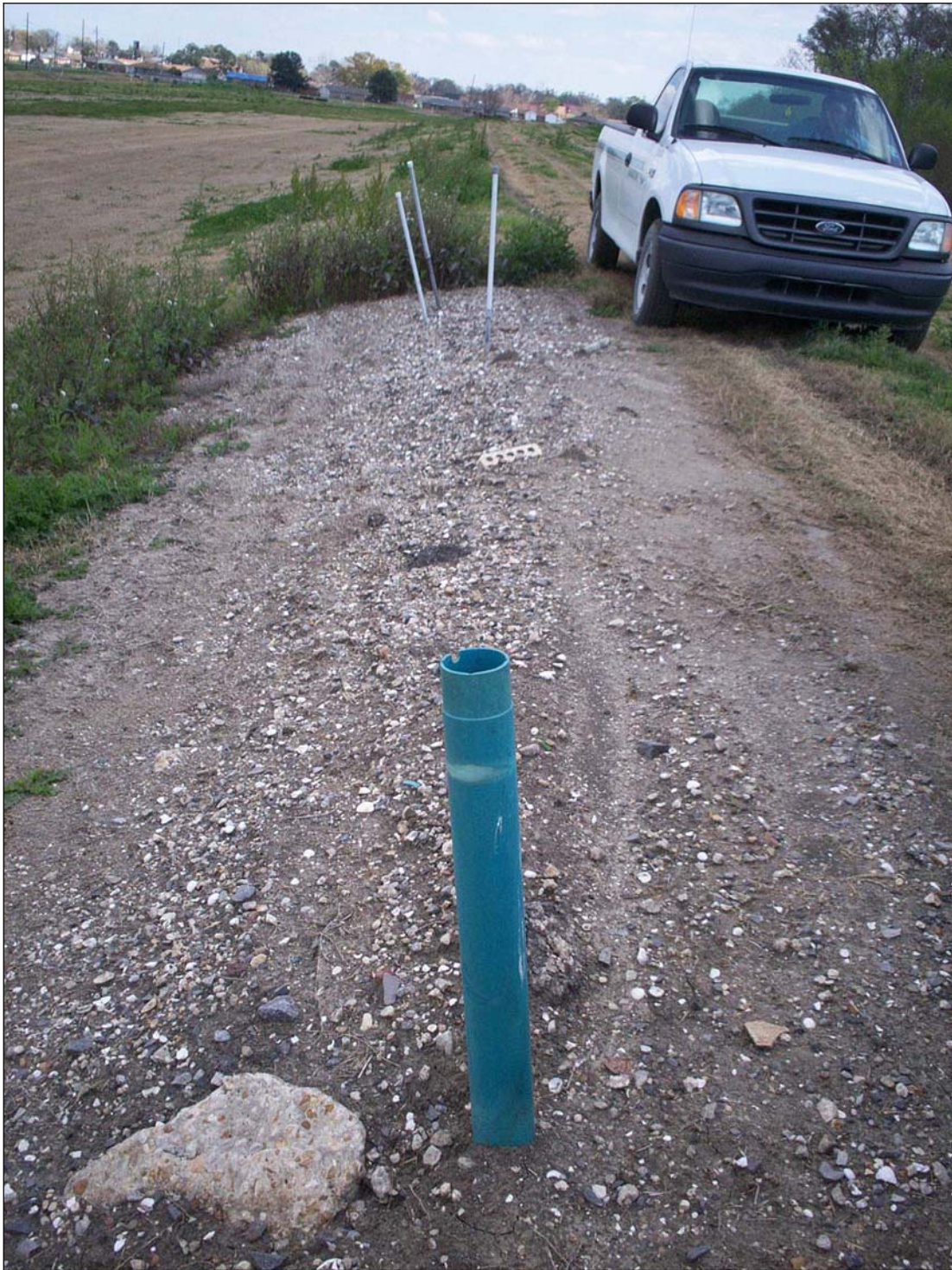
Photograph 8. Recent monitor well on levee in project corridor
