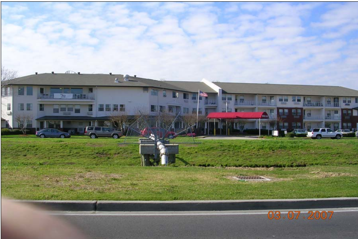
Photograph 2. Pipeline crossing project corridor
