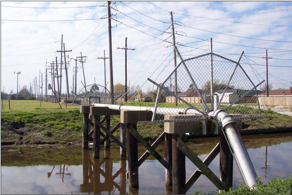
Photograph 9. Pipeline crossing project corridor
