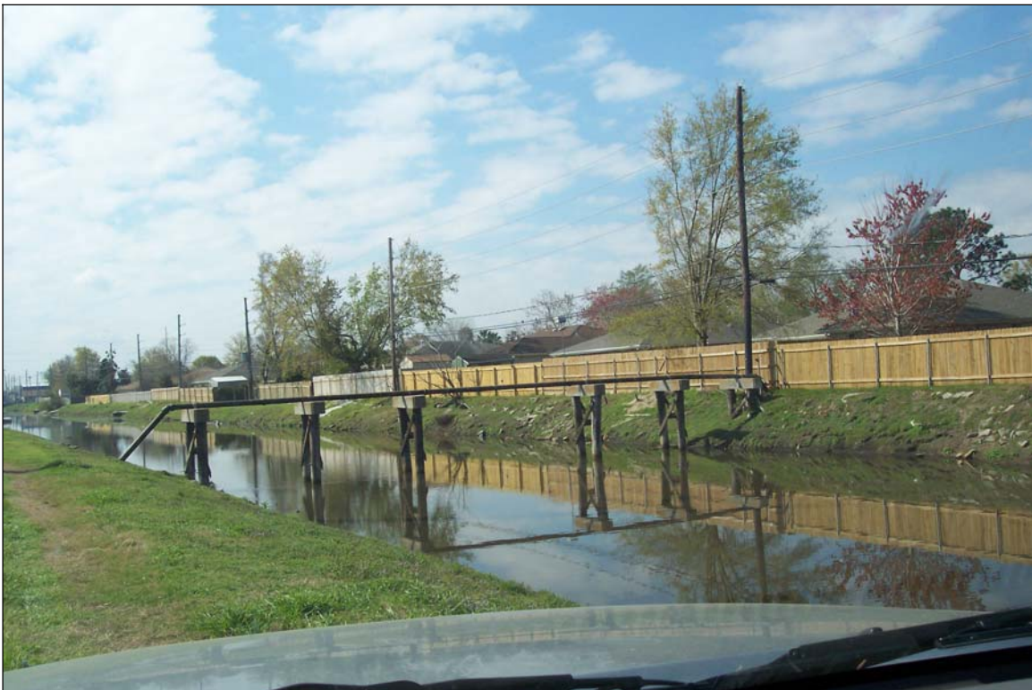
Photograph 10. Pipeline crossing project corridor
