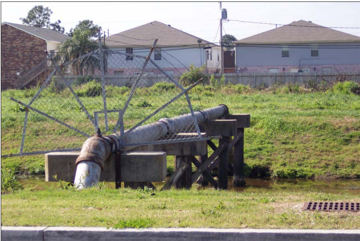
Photograph 4. Pipeline crossing project corridor
