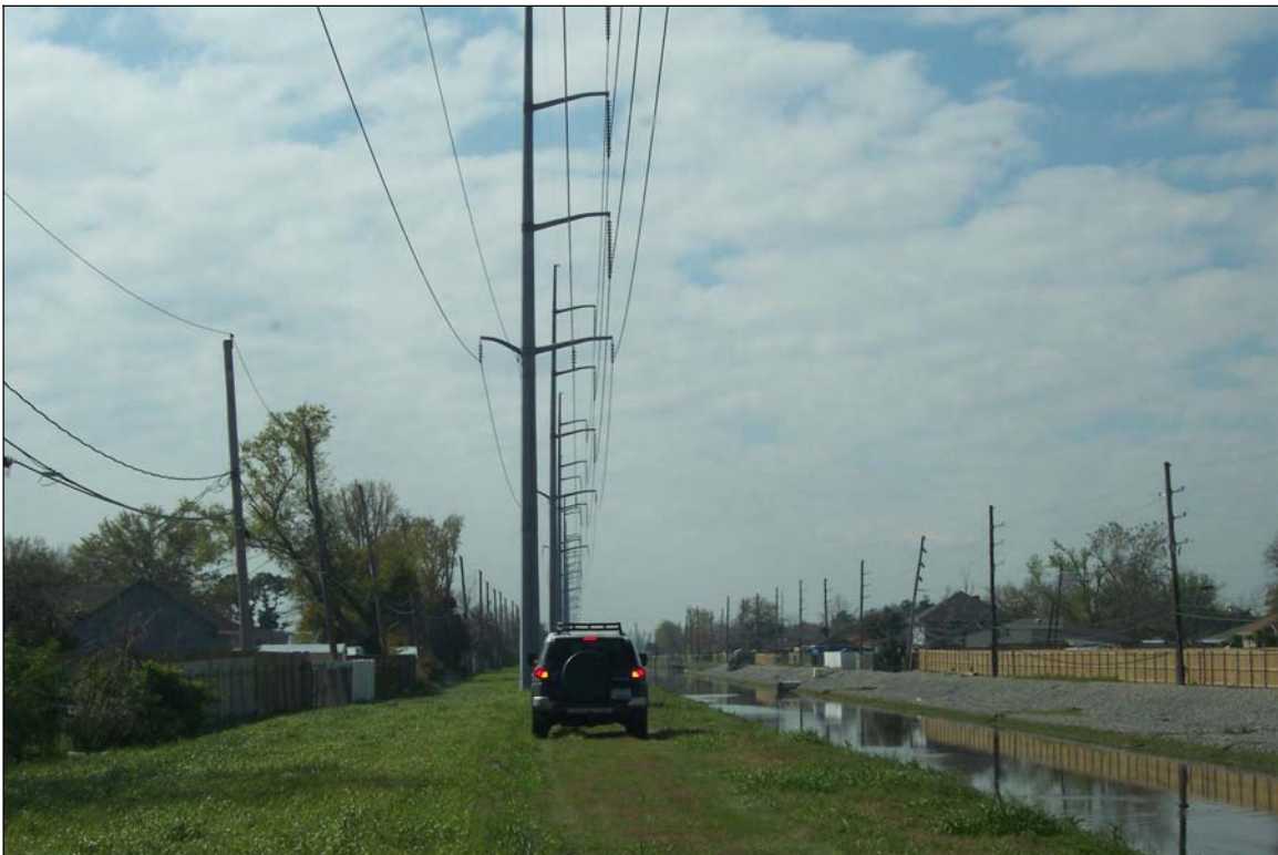
Photograph 20. Typical view to the south from Parish Line P.S. canal turn
