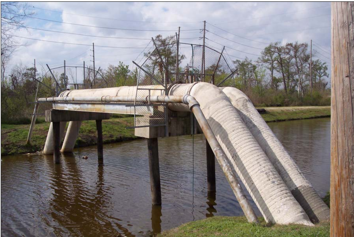
Photograph 14. Pipeline crossing project corridor
