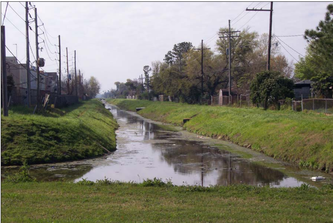
Photograph 24. Canal entering project corridor from the south
