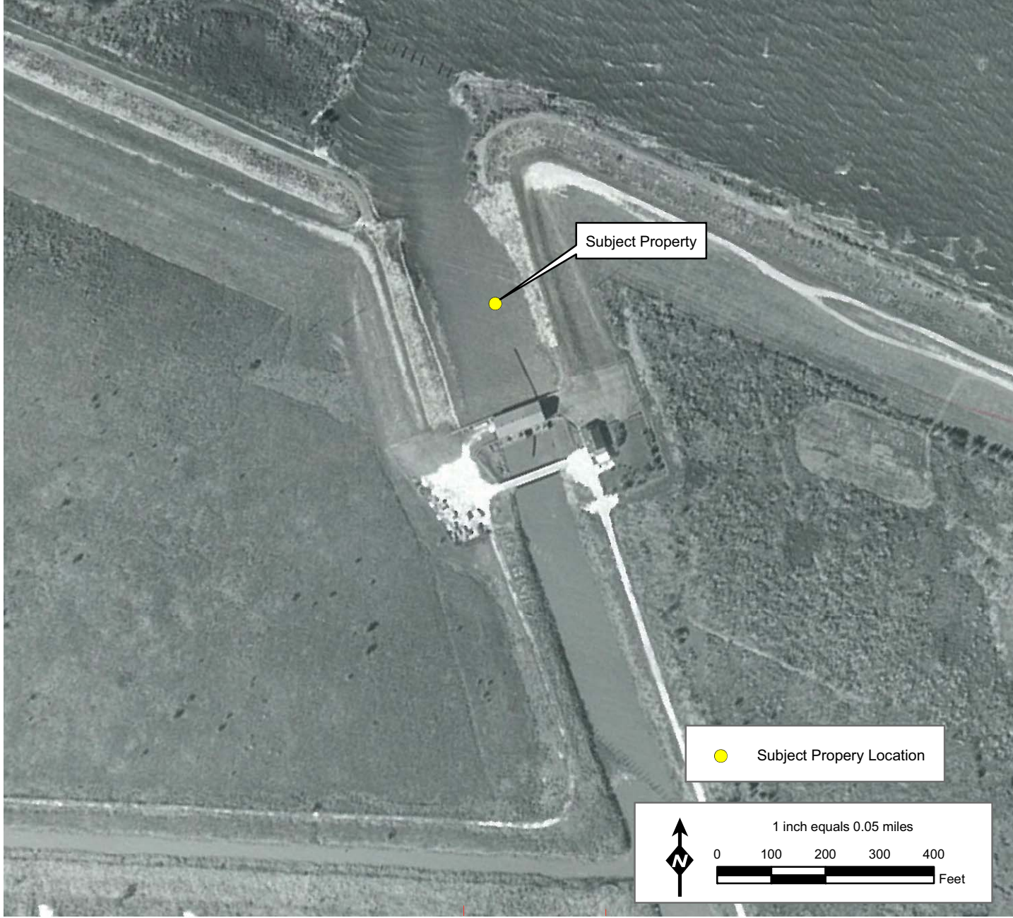
Elmwood Pump Station 1964 Aerial Photography
