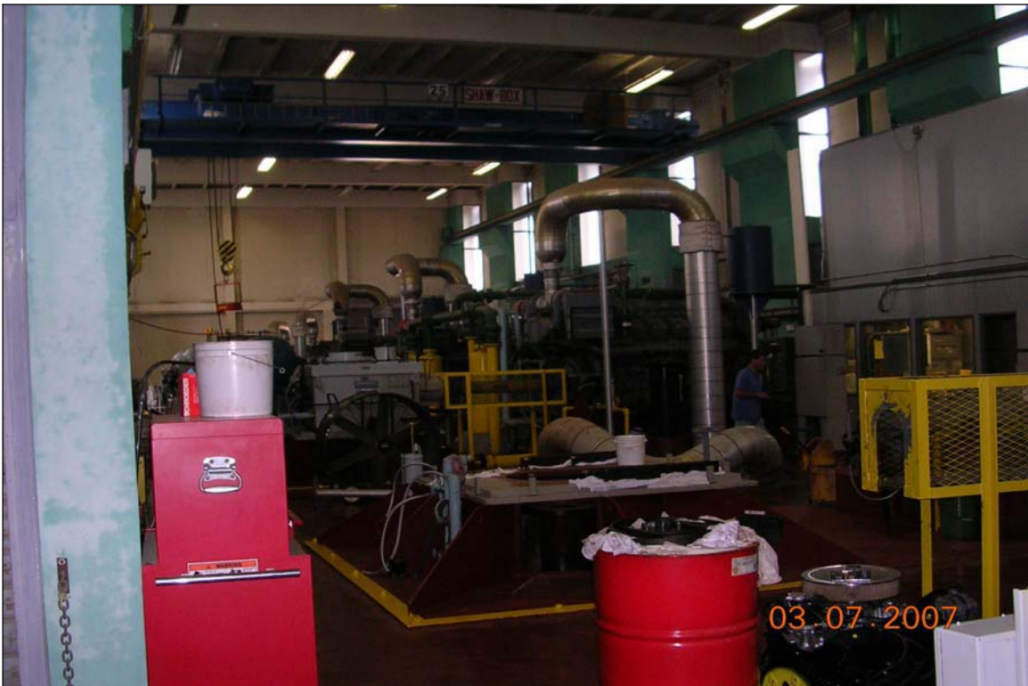
Photograph 12. Interior view of pump station building
