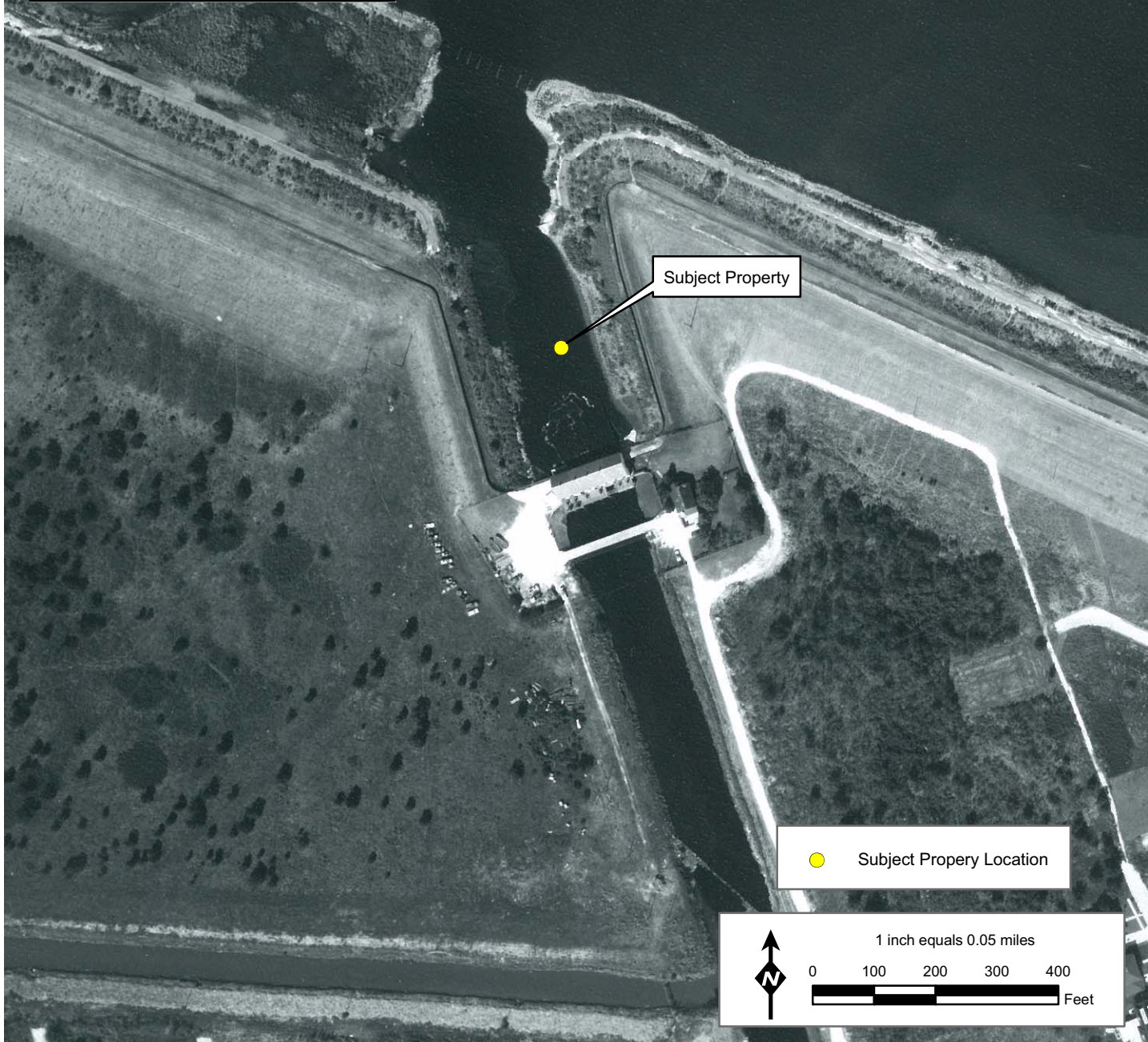
Elmwood Pump Station 1970 Aerial Photography
