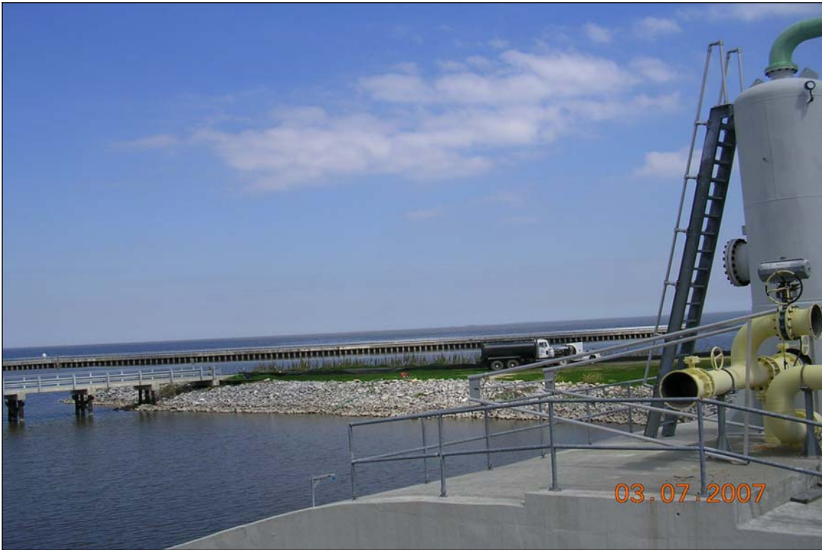
Photograph 9. View to the northeast of outfall basin and Lake Ponchartrain
