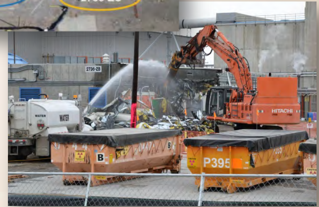
Demolition of PFP Vault Building
