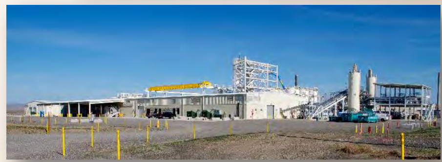
200 West Groundwater Treatment LEED Facility
