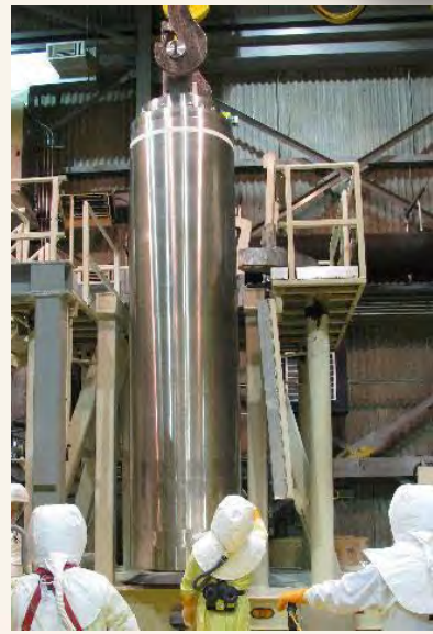
MCO #389 movement to trailer inside 105KW Transfer Annex
