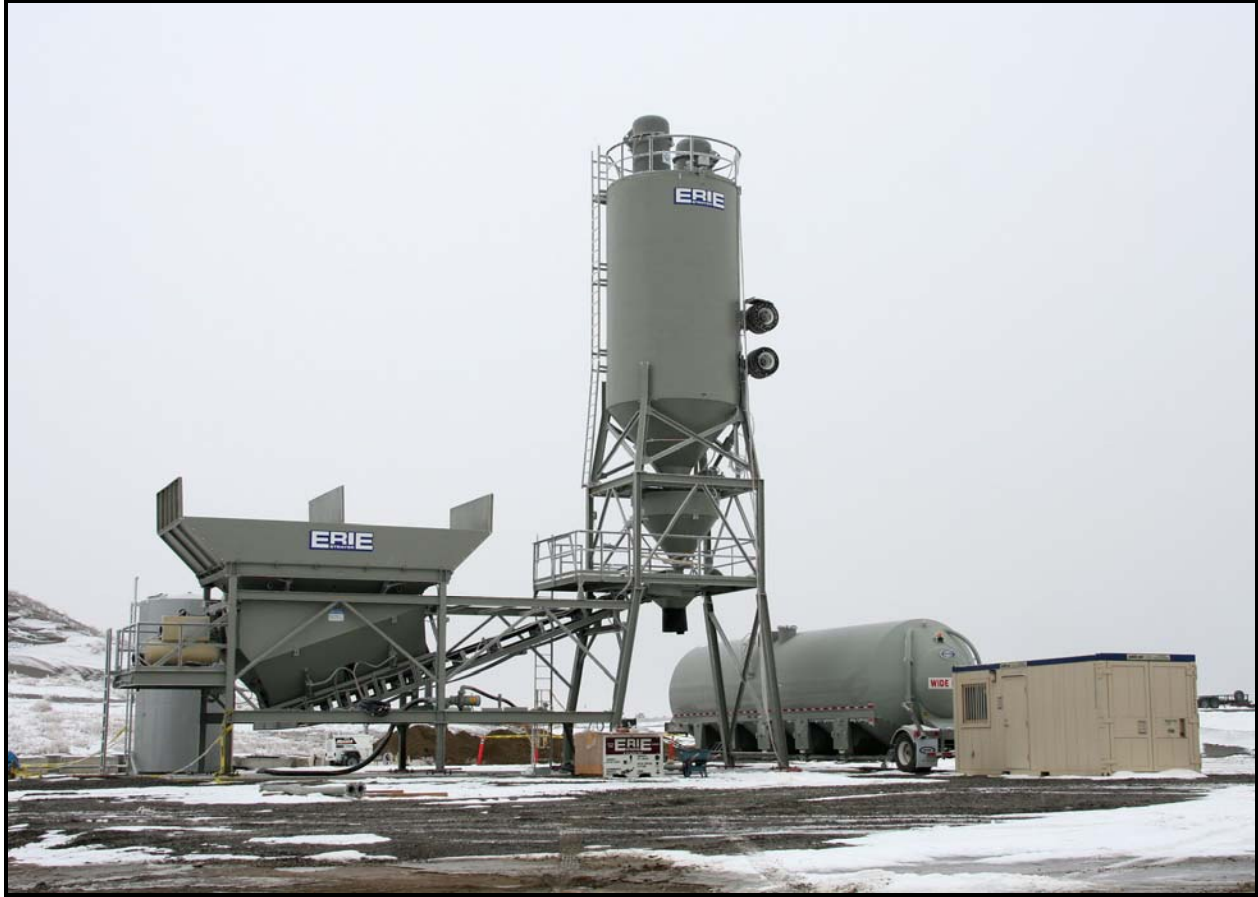
Assembly of the Environmental Restoration Disposal Facility's onsite batch plant is complete. The batch plant will be used to produce "flow fill." (Photo 4)
