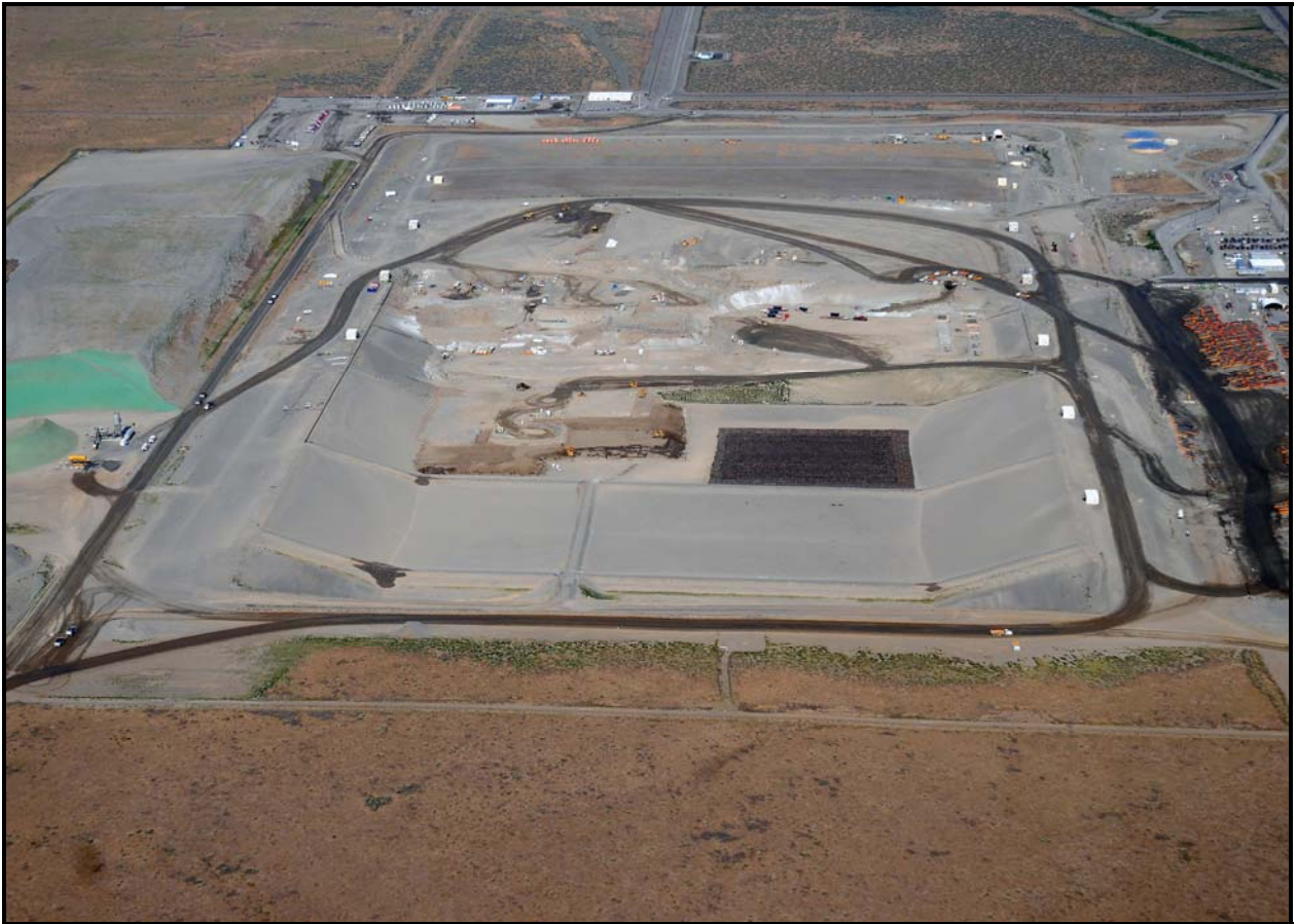
More than 11.5 million tons of waste has been disposed in the Environmental Restoration Disposal Facility. With the additions of super cells 9 and 10, the facility has a capacity of 16.4 million tons. (Photo 1)
