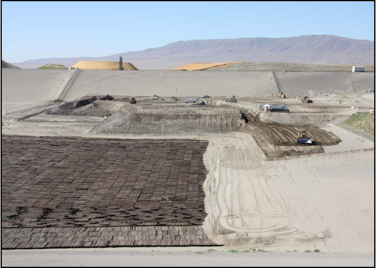
The Waste Operations team begins to spread contaminated soil over 58,500 railroad ties that were delivered to the facility this spring. (Photo 2)
