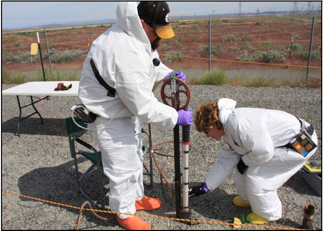
North Wind employees retrieve a multi-detector probe from a cone penetrometer of a vertical pipe unit during noninvasive characterization at the 618-11 Burial Ground. (Photo 7)
