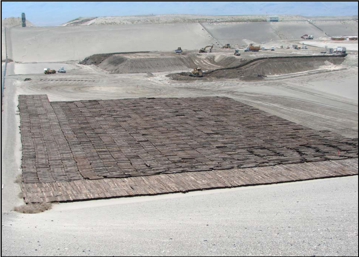
The Waste Operations team continues to dispose Hanford Site railroad ties in the north end of super cell 9 at ERDF. The facility is expected to receive more than 58,000 ties. (Photo 2)
