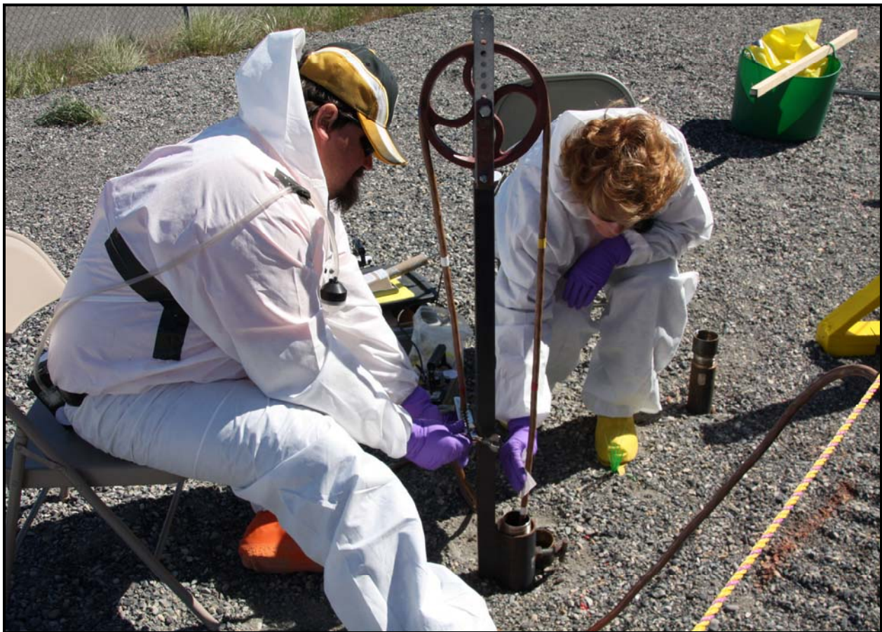
Employees with Washington Closure Hanford and subcontractor North Wind Inc. retrieve a multi-detector probe from a cone penetrometer during nonintrusive characterization of the 618-11 Burial Ground. (Photo 7)
