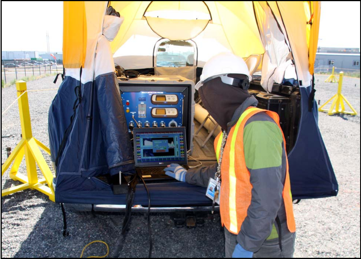
A North Wind employee takes readings during nonintrusive characterization of the vertical pipe units at the 618-11 Burial Ground. (Photo 9)
