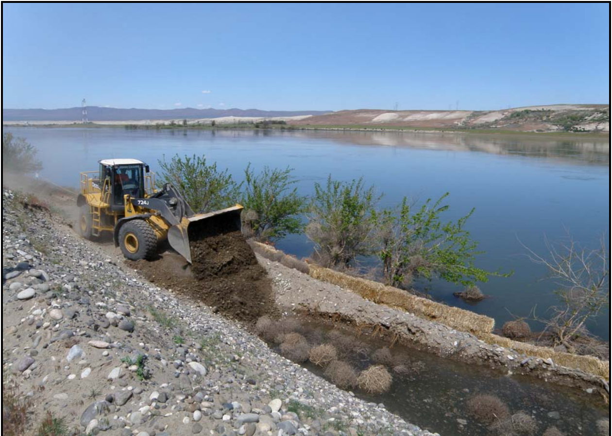
Washington Closure Hanford subcontractor Ojeda Business Ventures backfills site 100-F-45. (Photo 10)
