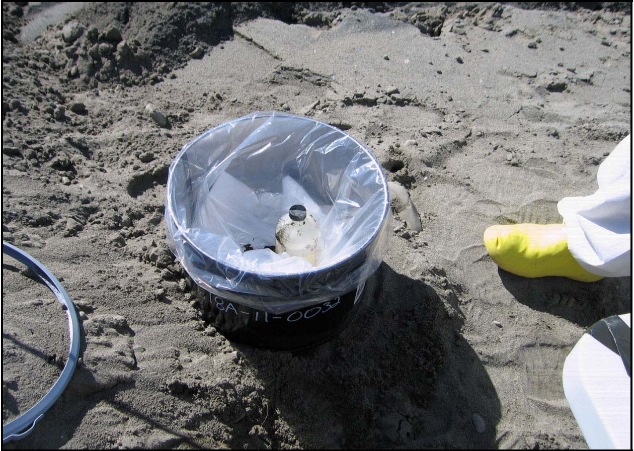
One of numerous bottles found during trench excavation on the north side of the 618-10 Burial Ground. (Photo 6)
