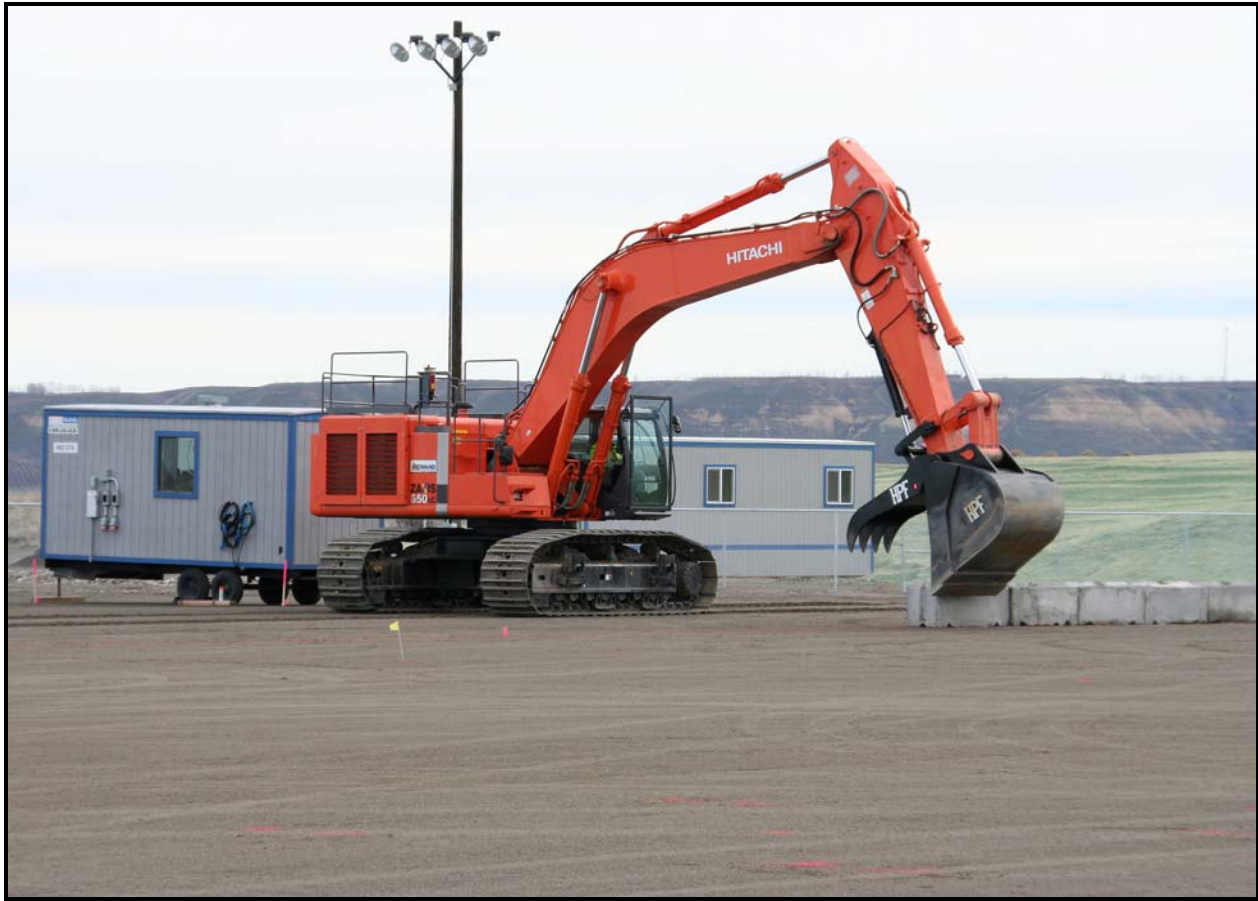
White Shield/Apollo places ecology blocks in the drum-punch area at the 618-10 Burial Ground. (Photo 8)
