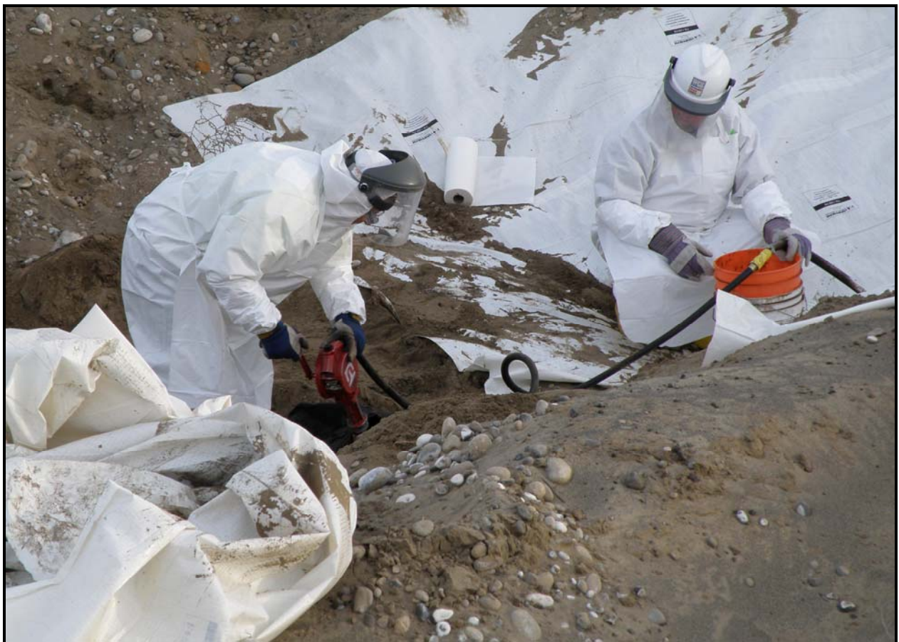
Washington Closure Hanford subcontractors drain waste oil from a drum discovered at 100-F-49. (Photo 12)
