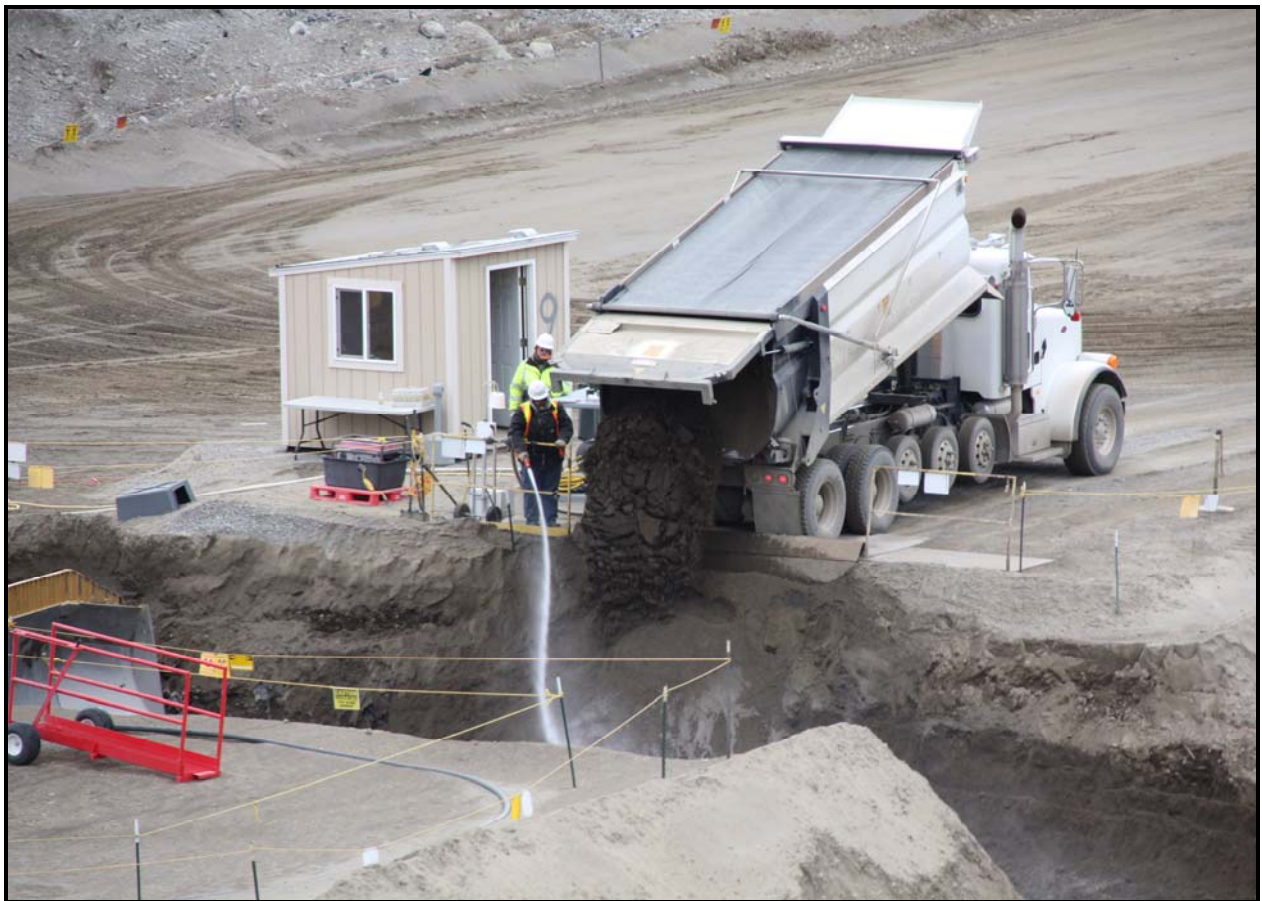
The Waste Operations team dumps waste that was introduced into super cell 9 at the Environmental Restoration Disposal Facility. (Photo 1)
