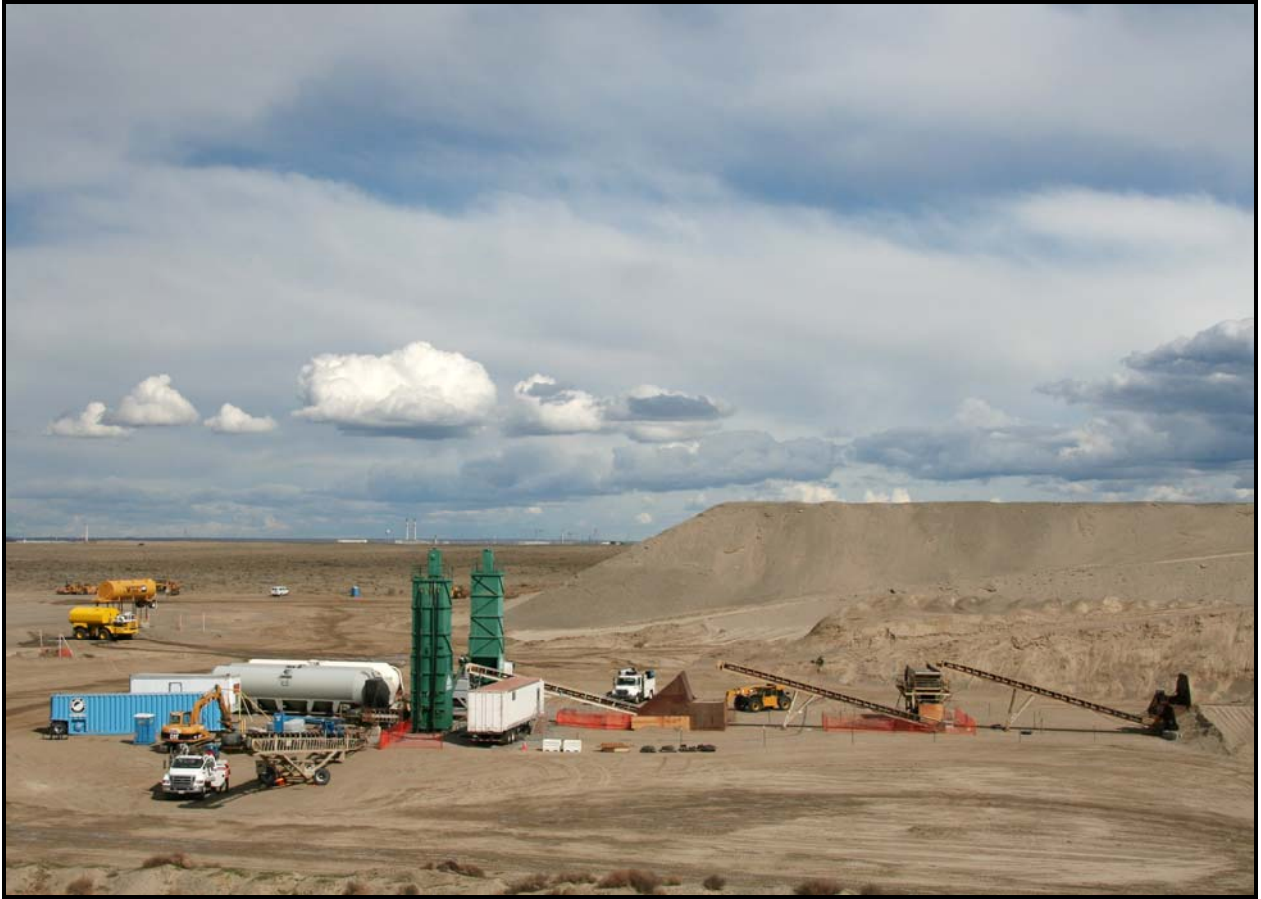
DelHur Industries has completed setup of the pug mill at the Environmental Restoration Disposal Facility.
