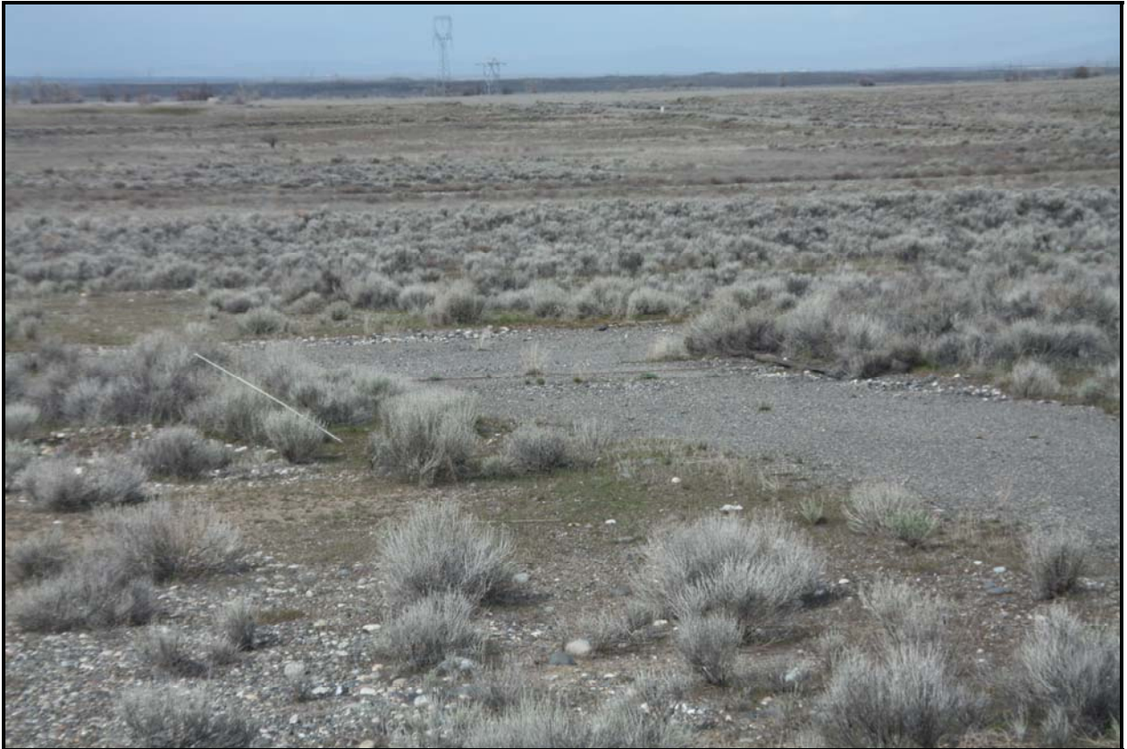
Waste site 100-F-47 is the foundation for a former electrical substation.
