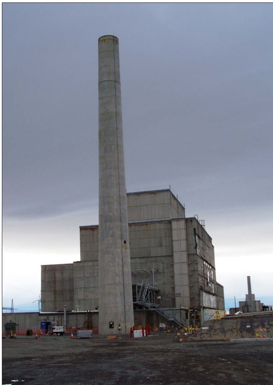
The 116KE Reactor Exhaust Stack as it exists today. Planning is under way for demolishing the 175-foot-tall stack later this fiscal year.
