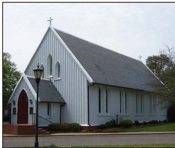
Carpenter Gothic chapel (1858) with board-and-batten siding at Fort Monroe, Virginia.
