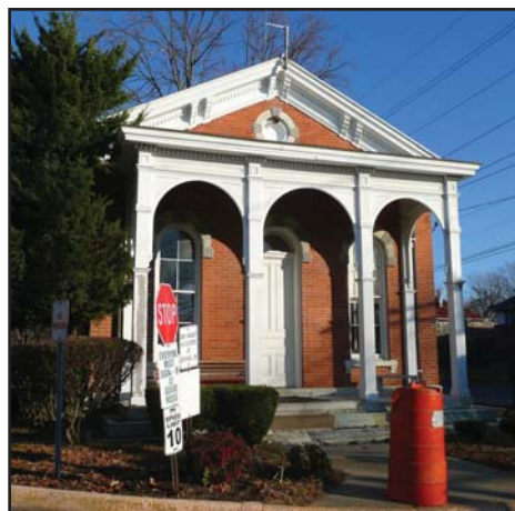
The Gate House (ca. 1864) at the Indianapolis Arsenal is characterized by a round-arched door, round-arched windows, and round-arched porch bays.
