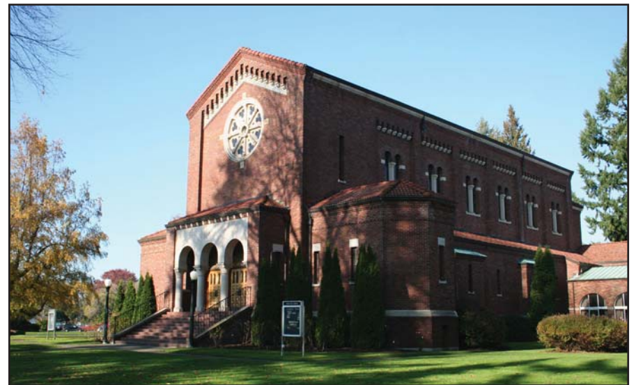
The Main Post Chapel (1934) at Fort Lewis, Washington, exhibits features from the Romanesque Revival style, including the prominent gable front, round-arched arcade, and round-arched cornice.
