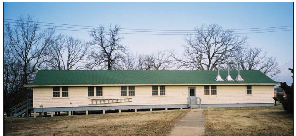
Top: 700-series barracks (1941) at Fort Leonard Wood, Missouri, has the unique aqua media between the two floors and a canopy over the second-floor windows.
