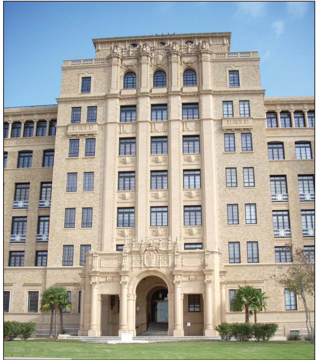
The old Brooks Army Medical Center (1937) at Fort Sam Houston, Texas, features a Churrigueresque interpretation of the Beaux Arts, illustrated by masonry materials, arcades, pilasters, balustrade windows, cartouches, and roof balustrades.
