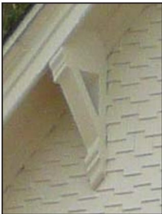
Left: Elbow bracket under eave at a Stick-style officer's quarters at the Presidio of San Francisco.
