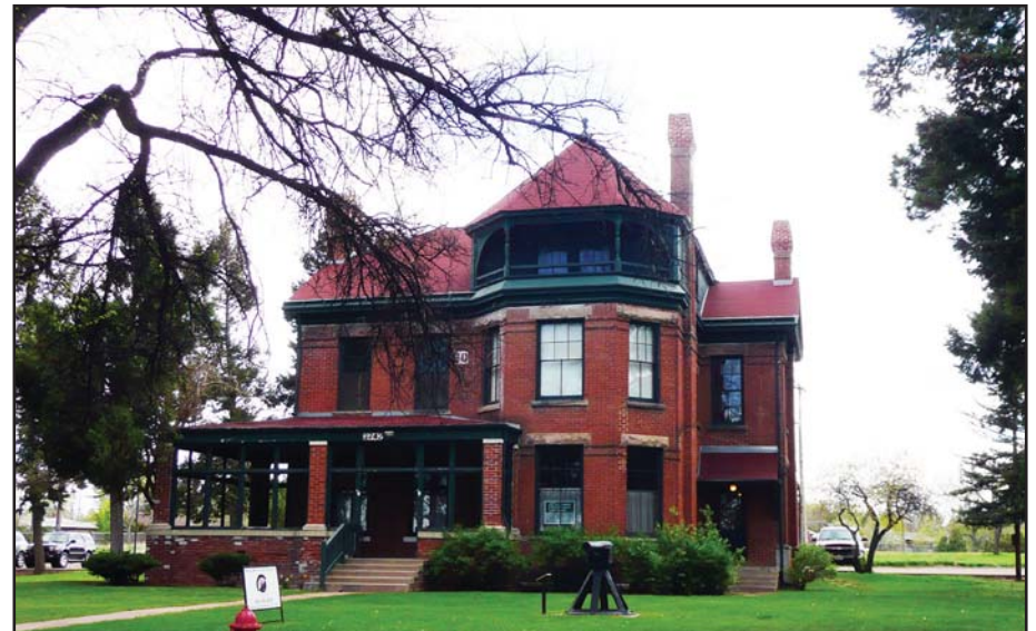
Top: This officer's quarters (1886) at Vancouver Barracks, Washington, displays many defining features of the Queen Anne style including asymmetrical massing, elaborate wraparound porch, turret, multi-light windows, and varying types of woodwork.
