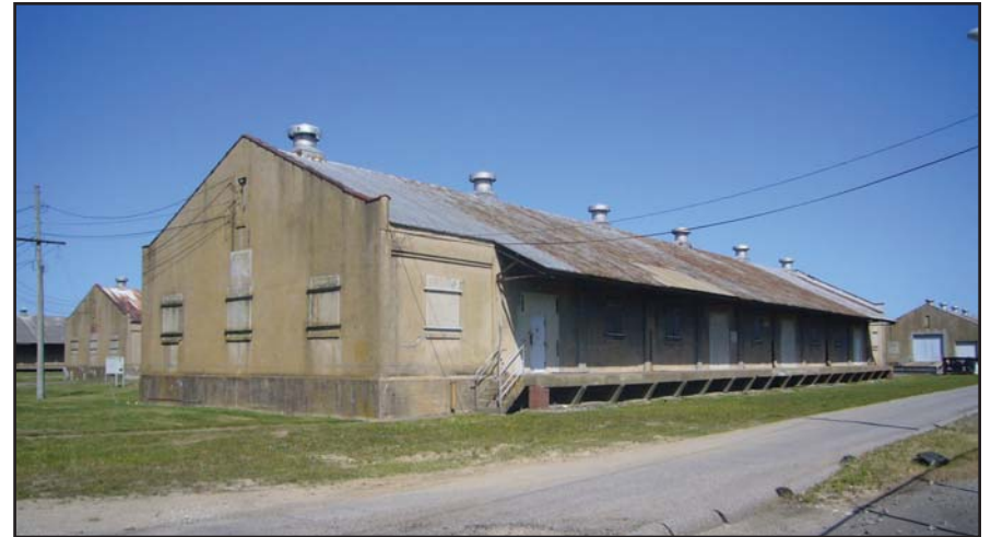
Gabled ends, covered loading docks, horizontal massing, and roof ventilators are characteristic of storage and warehouse buildings, as shown at this concrete storehouse building (ca. 1918) at St. Julien's Creek Annex (NSA Norfolk Naval Shipyard), Virginia.
