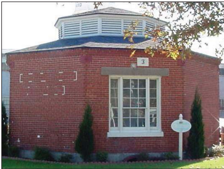
Building 3 (1835) at Naval Support Activity Norfolk Naval Shipyard, Virginia, has the character-defining features of the geometrical shape, pyramidal roof, and cupola of the style.
