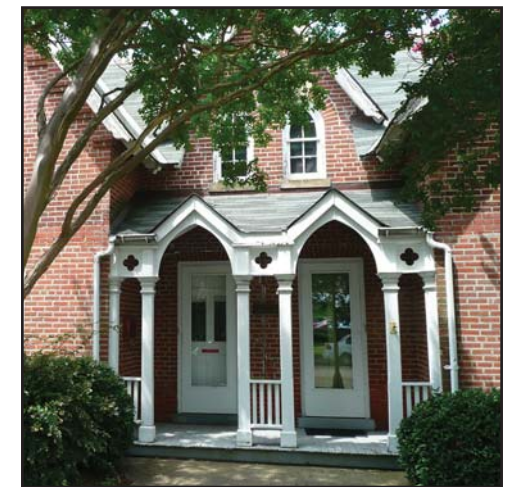
Gothic Revival officers' quarters (ca. 1889) at Fort Monroe with pointed arches and quatrefoils.
