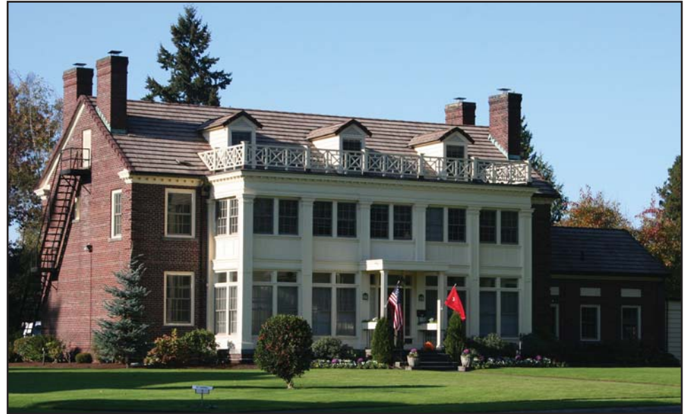
The Post Commander's Quarters (ca. 1930) at Fort Lewis, Washington, maintains the gable roof, gable dormers, rooftop balustrade, and double-hung windows of the Colonial Revival style.
