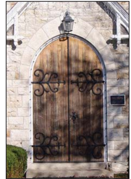
Both of these doors have pointed arch forms and vertical board construction. The one on the right also has the decorative iron strap hinges.
