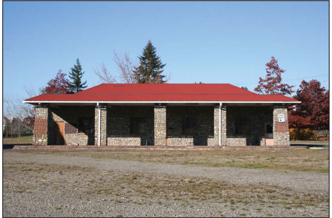
The Federal Prison inmates (Fort Lewis) built this service station (1938) at Fort Lewis out of stone in the Rustic style.
