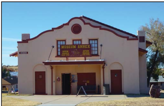
Above: The old Post Theater (1934) at Fort Huachuca, Arizona, with a curvilinear and decorated roofline.
