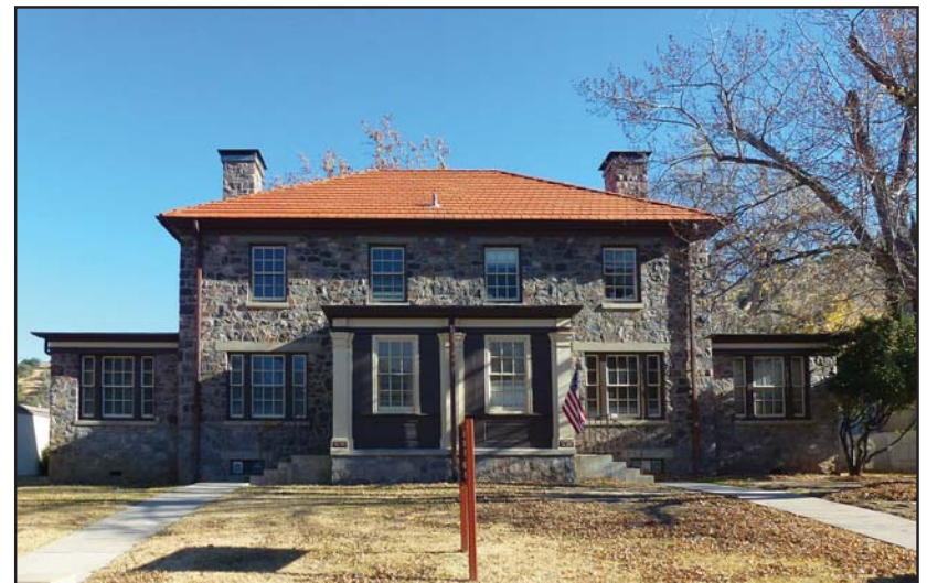
The duplex (top, 1932) is a French Revival adaptation at Barksdale Air Force Base, Louisiana, but the standardized plan is the same as the duplex (bottom, 1939) in the Colonial Revival style in stone at Fort Huachuca, Arizona. This plan was also executed in wood, red brick, yellow brick, and stucco at other installations.
