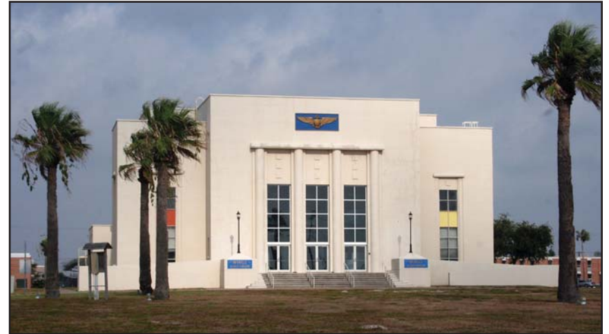
The theater (1941) at Naval Air Station Corpus Christi, Texas, is a restrained example of the style. It has a flat roof, smooth wall surface, and vertical emphasis at the entrance consistent with the style.
