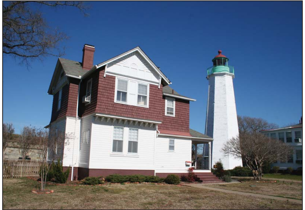
The Old Point Comfort Light Keeper's House (1891) at Fort Monroe, Virginia, built by the Light House Service, displays shingle siding, a prominent front gable, half-timbering in the gable, and exposed brackets of the Stick style.
