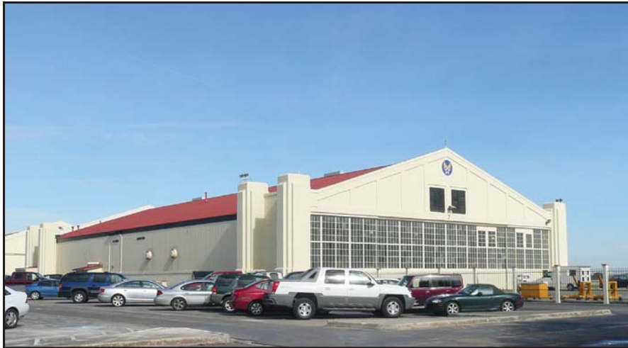
The old hospital (top, ca. 1905) at Fort Sam Houston, Texas, with an entrance porch and double-story porch allowing access from the former wards and a hangar (bottom, ca. 1930) at Randolph Air Force Base, Texas, with form, corner towers, and full-width doors as defining features.
