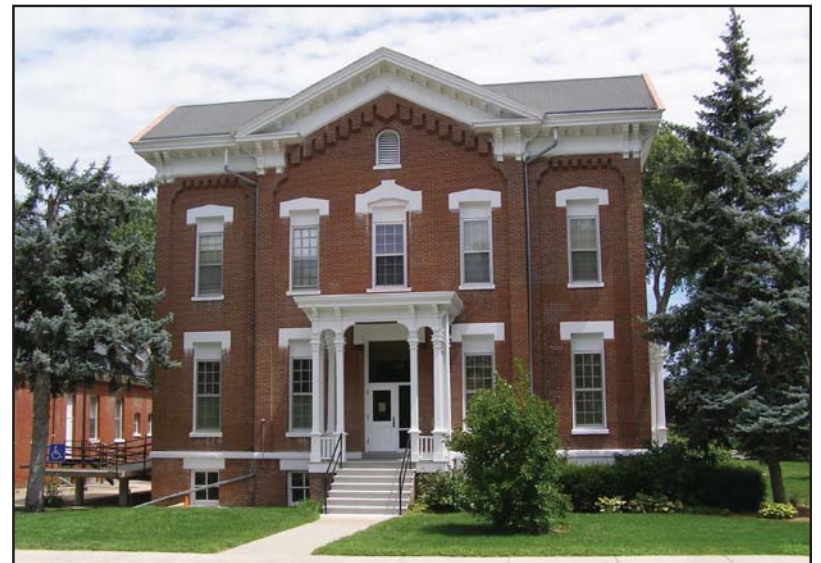
The Headquarters Building (1879) at Omaha Barracks has a bracketed cornice and an elaborate porch.
