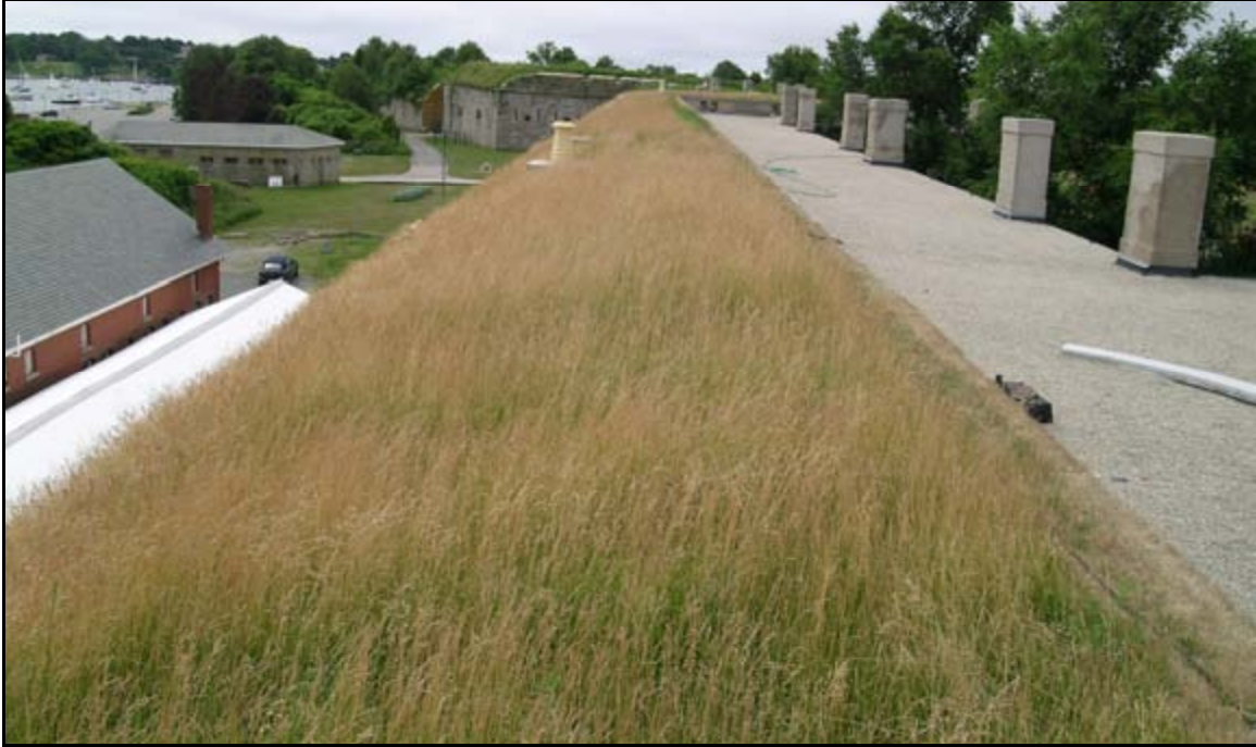
Photograph 50: View looking at earthen rampart at Fort Adams, Newport, Rhode Island. The sea grass planted on the rampart is left uncut to provide greater erosion protection to the soil underneath. The sea grass was specifically chosen for the coastal conditions of Rhode Island. (Photograph by T. Beckwith, July 2005).
