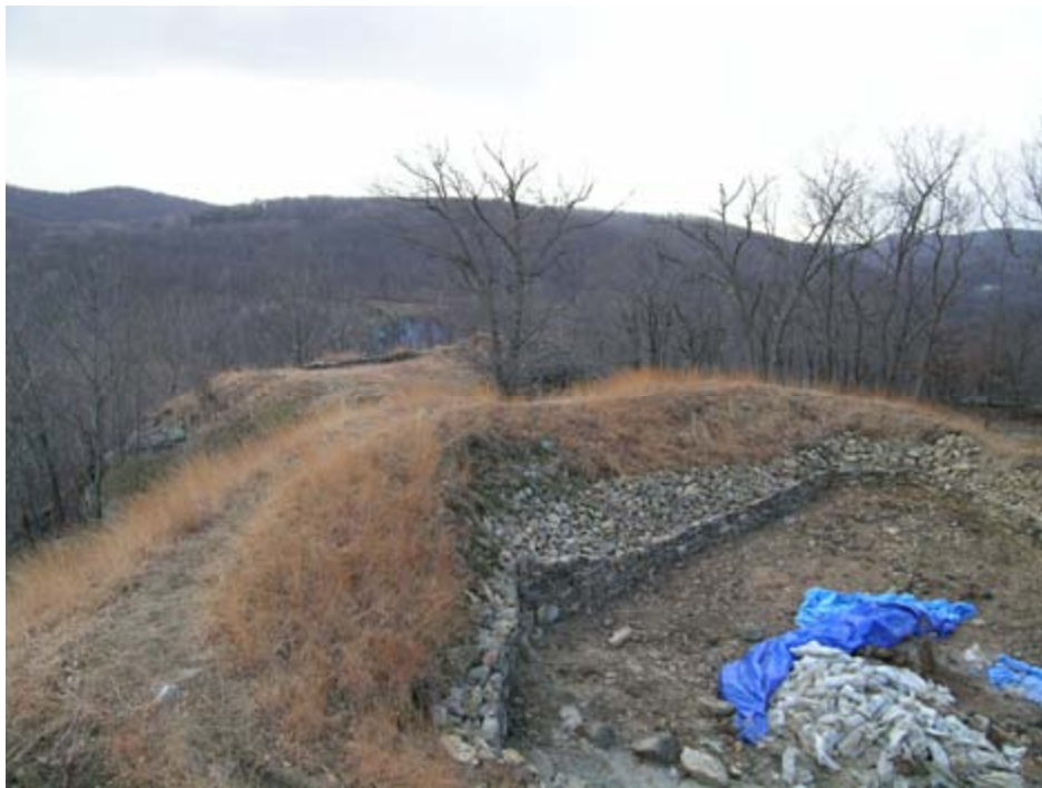
Detail, Interior of Redoubt No. 2, following demonstration project. [D. Cubbison, January 2006]
