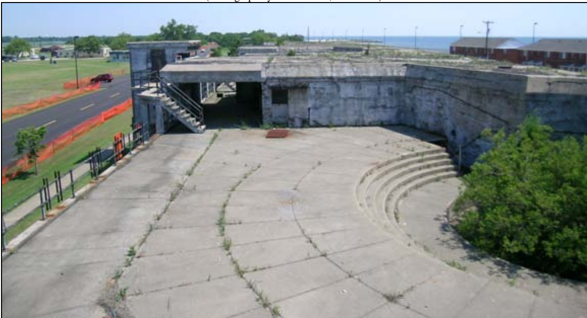
Photograph 16: View looking at Battery DeRussy, Fort Monroe, Virginia. The horizontal surfaces surrounding the gun emplacements appear to be in remarkable shape. Although there is some biological growth in the seams, there is very little cracking or erosion of the surfaces. What little vegetation there is in the seams should be removed to facilitate drainage and natural drying.
