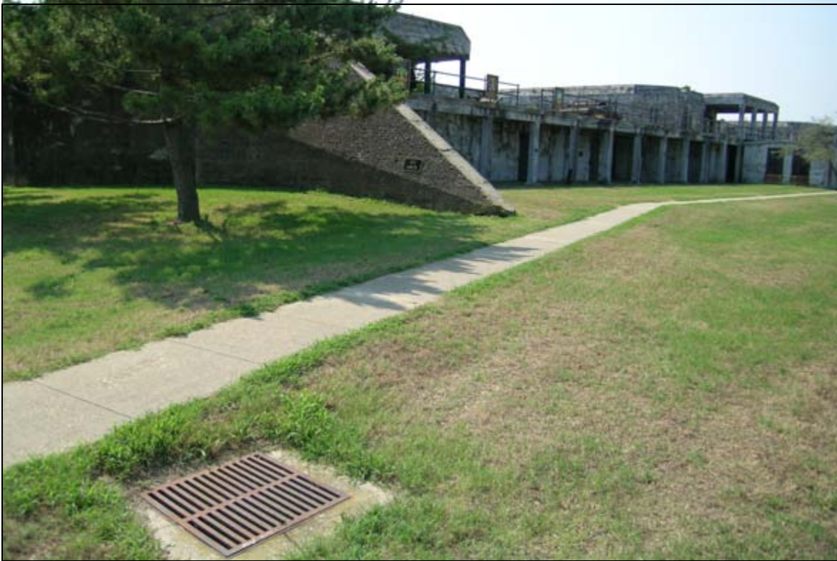
Photograph 54: Installation of a new sidewalk in the rear of Battery DeRussy at Fort Monroe altered drainage patterns, and separated the battery from the storm water drain in the foreground. The result is water pooling and failing to drain from this Endicott Series Battery.
