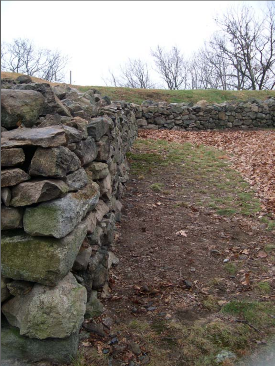
Photograph 18: Redoubt Four (1779-1783), Fortress West Point, Dry-Laid Stone Walls at West Reentrant Angle. (Photograph by D.R. Cubbison)
