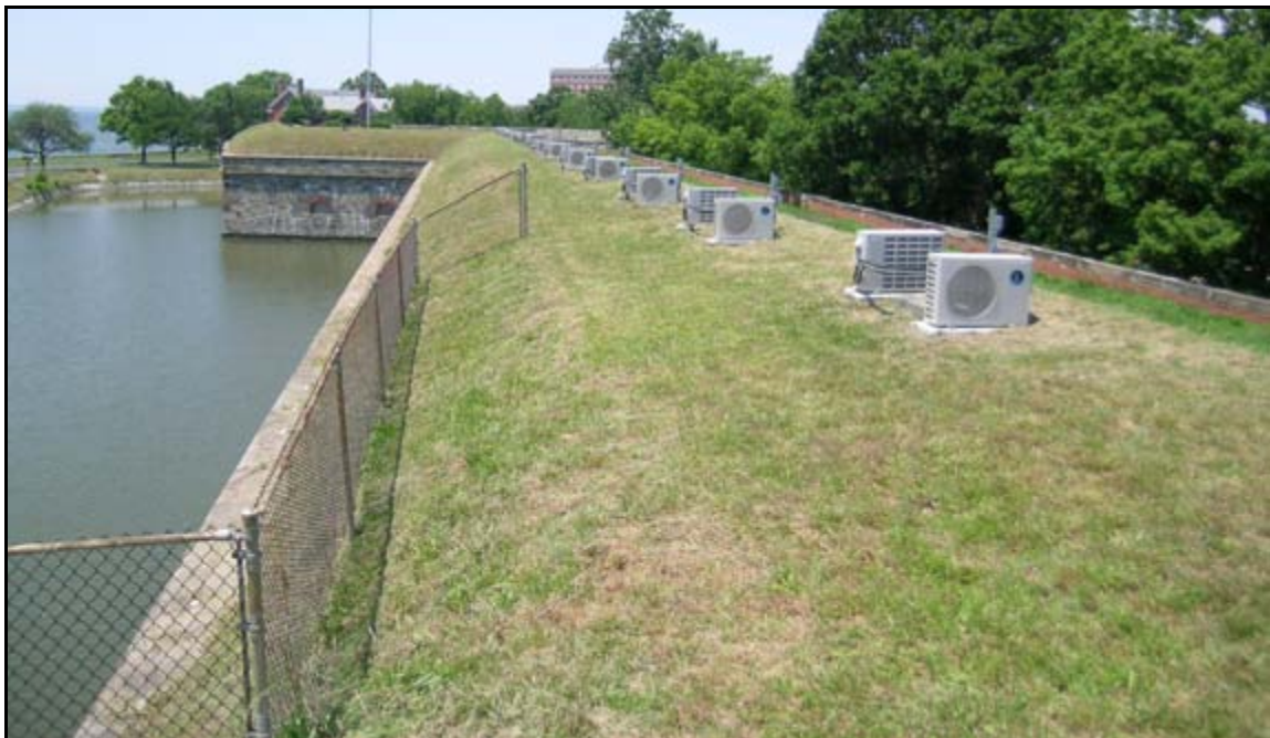
Photograph 44: View looking at the top of the Casemate 21, Fort Monroe. The parapet placed on top of the casemates makes it difficult to inspect the condition of the drainage system and to make repairs. The units located along the ridge are air conditioning units, installed within the original smoke vents through the parapet. (Photograph by T. Beckwith, June 2005)
