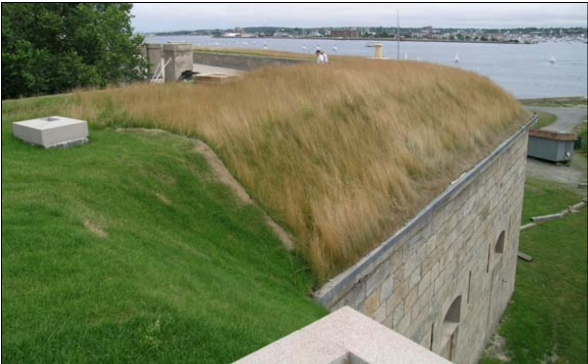
Photograph 51: Another view looking at the earthen rampart at Fort Adams, Rhode Island. Note the flashing located between the earth and the cordon stone. (Photograph by T. Beckwith, July 2005).
