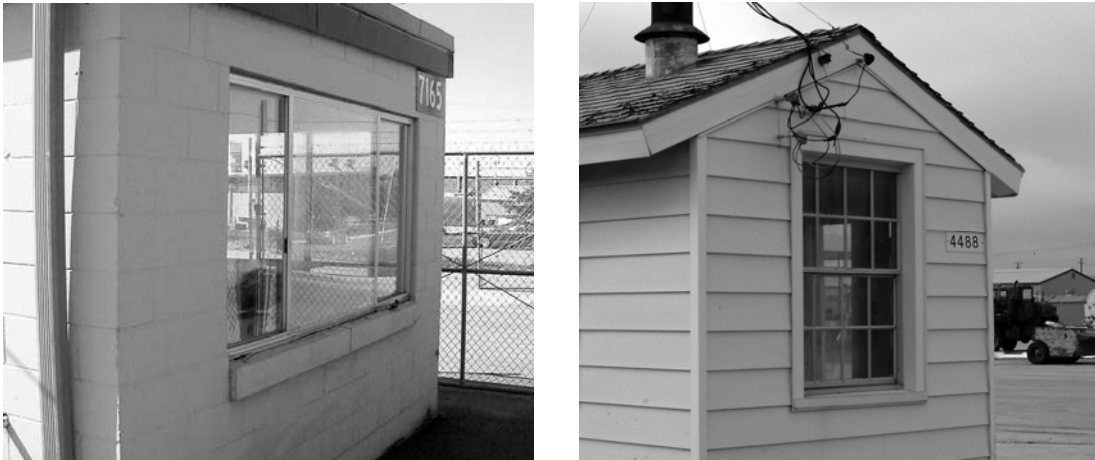
Figure 4.1. Sliding (left) and hung (right) windows (ERDC-CERL 2007, 2004).
