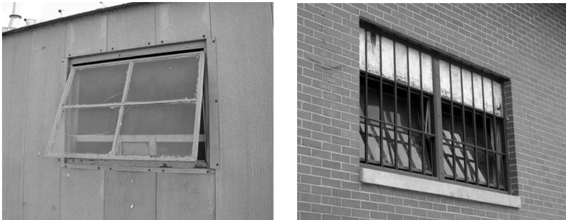
Figure 4.2. Awning (left) and hopper (right) windows (ERDC-CERL 2007).
