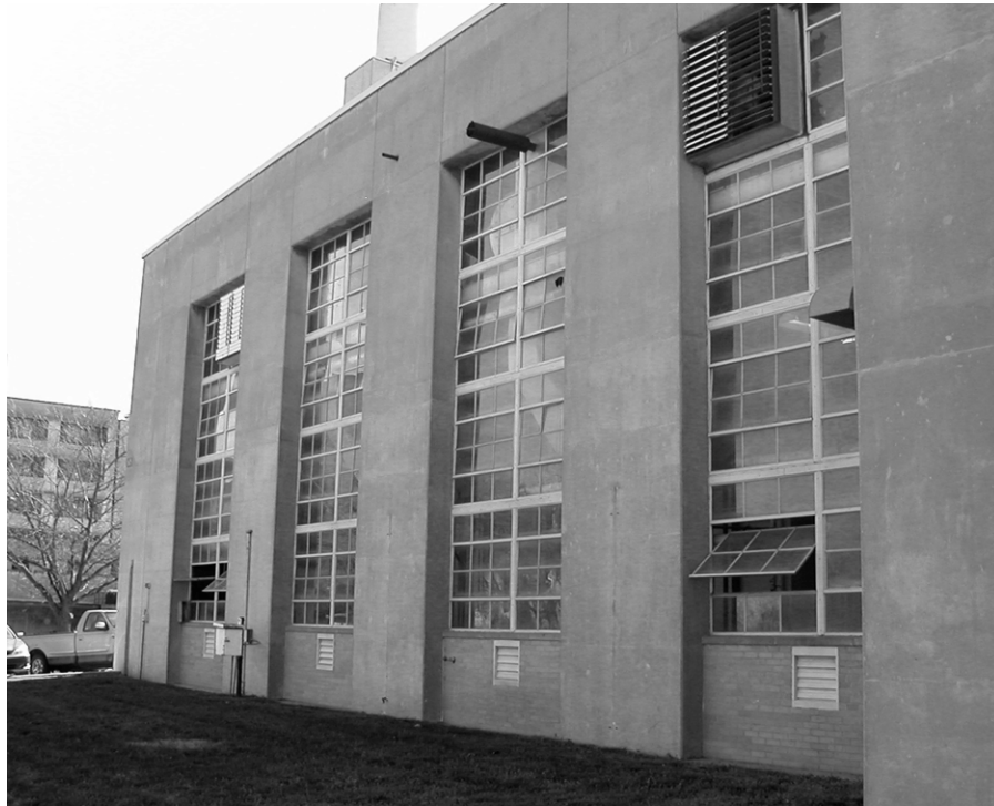
Figure 4.3. Factory-style muntins and mullions (ERDC-CERL 2007).
