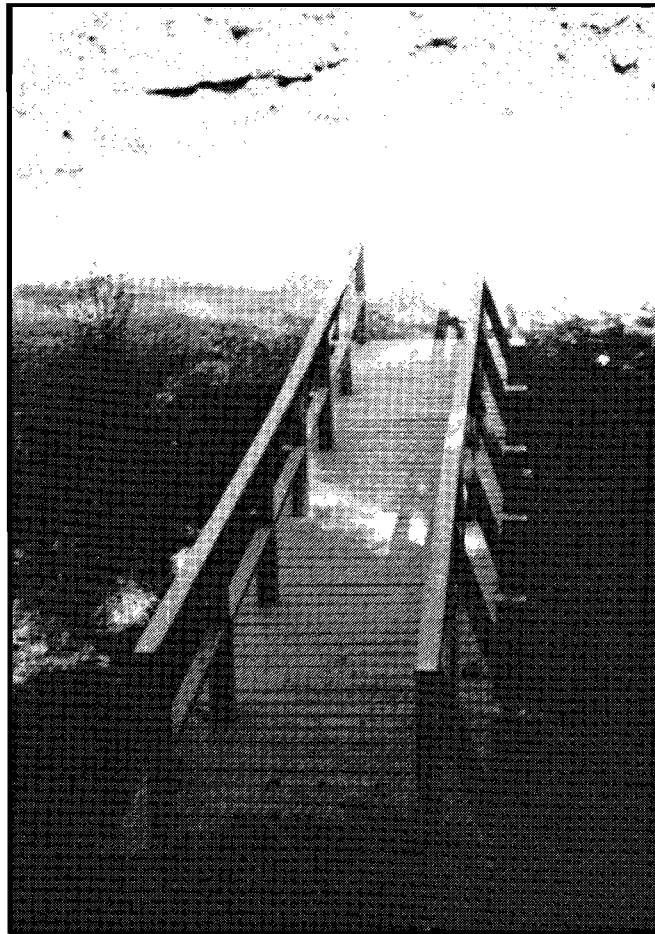
Figure P.9. Bridge constructed at Rappell Cliffs Rockshelter to facilitate access.
