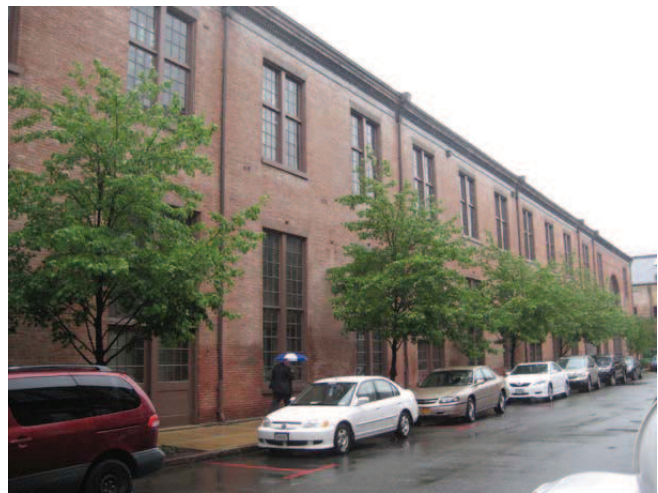
Figure 85: The exterior shell of Building 33 was retained
