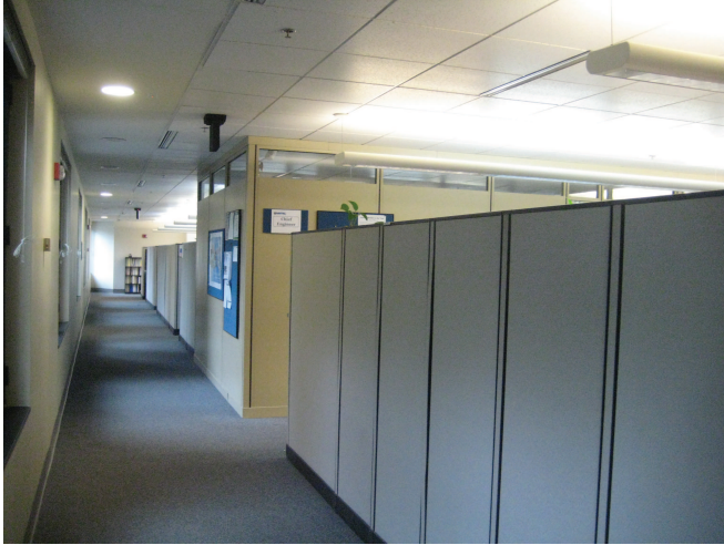
Figure 98: Lighting Building 33 Photo shows indirect and direct ambient lighting
