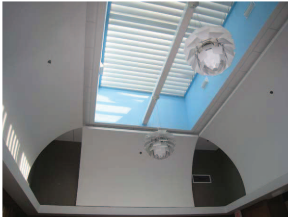
Figure 109: New conference room skylight
