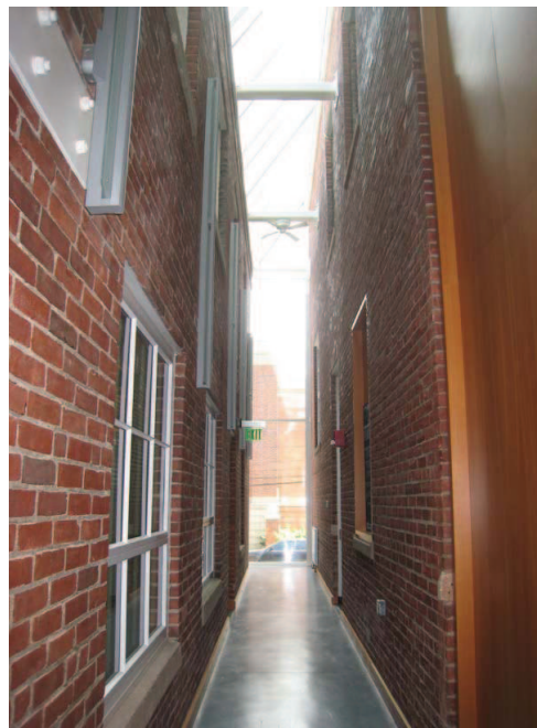
Figure 75: Glass enclosure connecting the buildings
