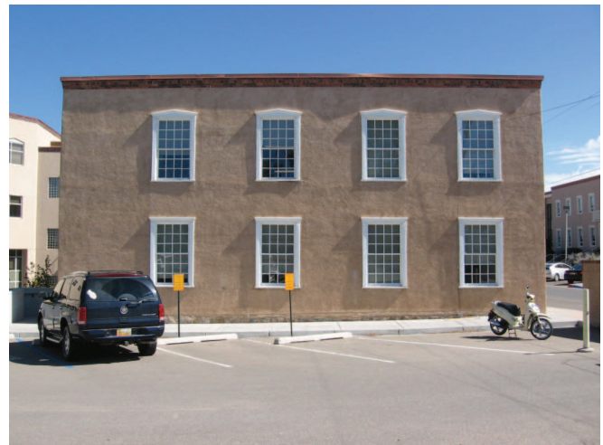
Figure 73: Historic windows with ceramic film on glazing
