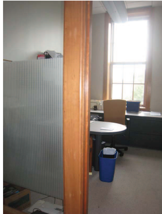
Figure 107: View into a private office showing the transparent and translucent separation wall to the corridor
