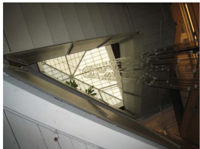
Figure 101: View of skylight from lower level
