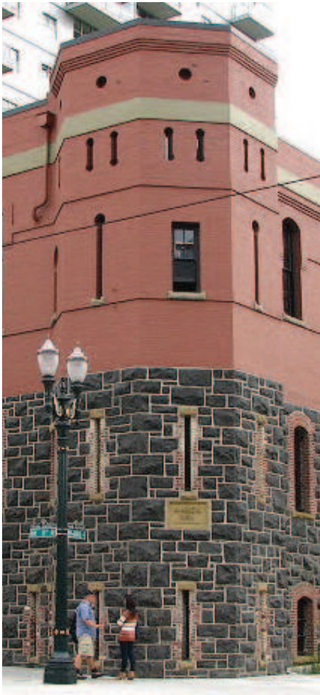
Figure 125: Exterior view of rebuilt corner turret
