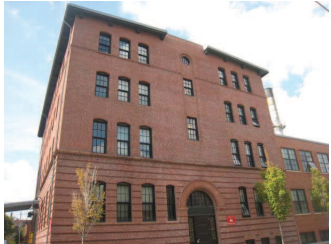
Figure 74: Diary building façade - note historically appropriate replacement windows
