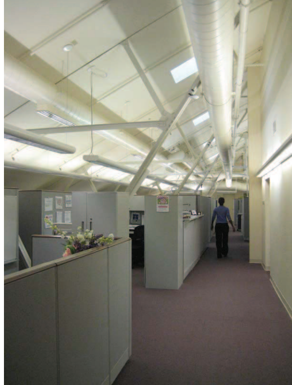
Figure 64: Photovoltaic sensors such as these help control lighting based on the amount of ambient light
