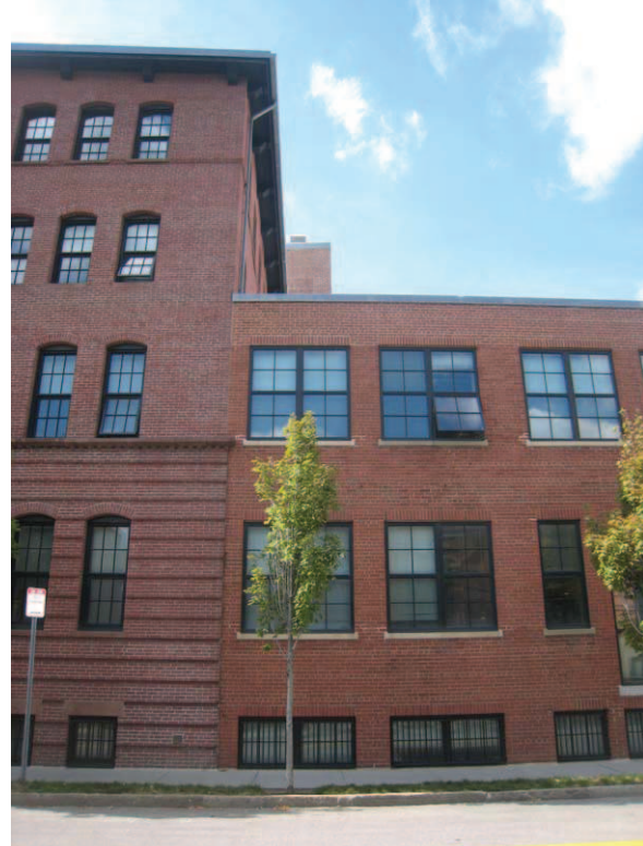
Figure 112: Exterior view where several open windows are visible
