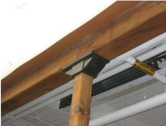
Figure 120: Re-used original beam and column
