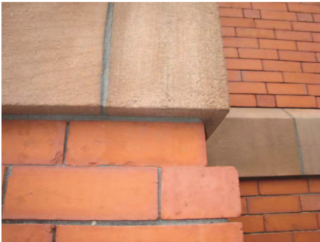
Figure 76: Close up of repointing at The Annex.
