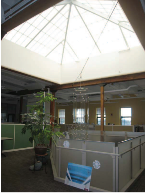
Figure 102: View of skylight
