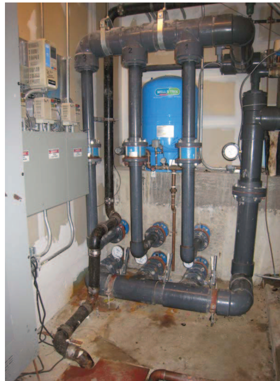
Figure 81: Connection to ground source heat pump
