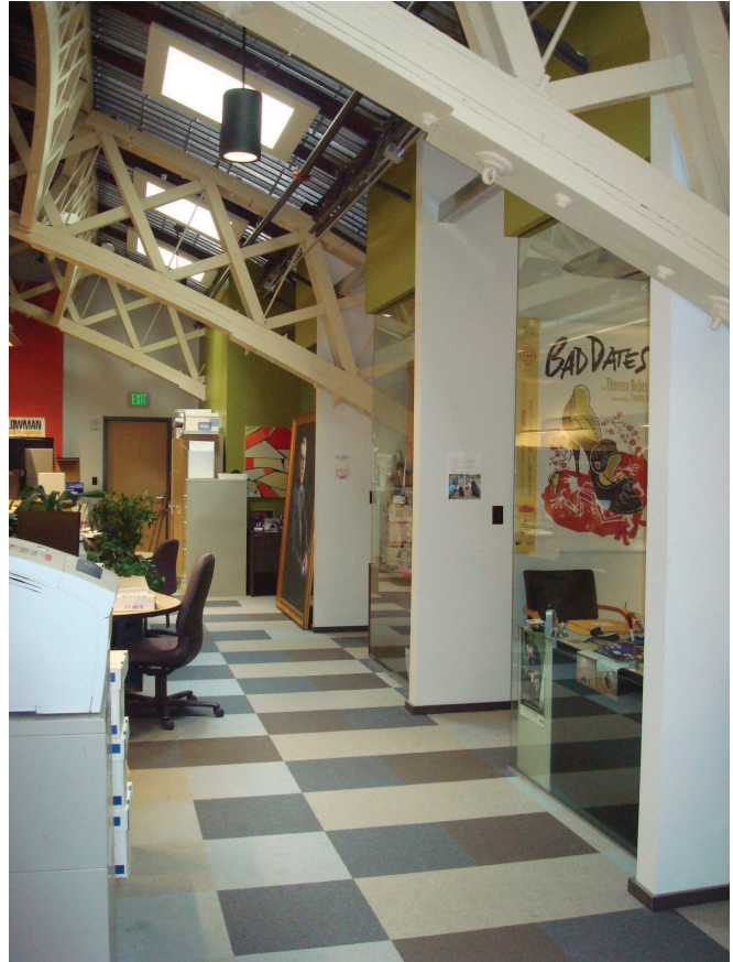
Figure 104: Upper office space showing existing historic roof structure and new skylights for daylighting
