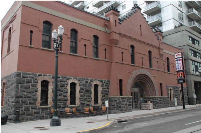
Figure 124: Exterior view of front entry to armory showing restored facade
