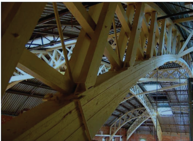
Figure 103: Note operable skylights between historic trusses
