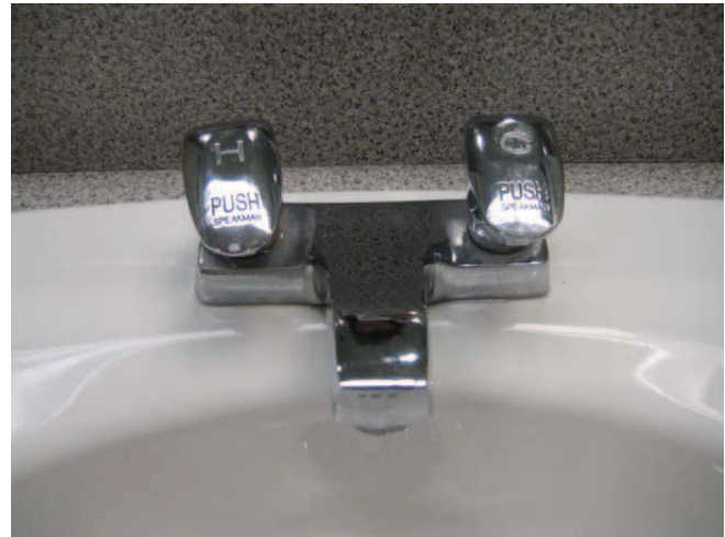
Figure 91: Low flow fixtures such as this faucet in a bathroom in Building 33 help reduce water use significantly
