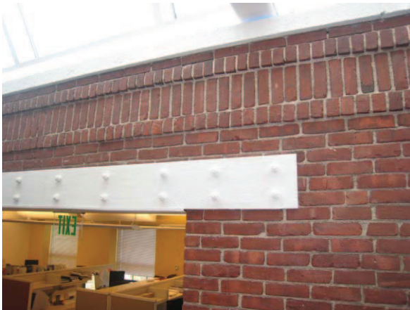
Figure 122: Original brick and steel lintel
