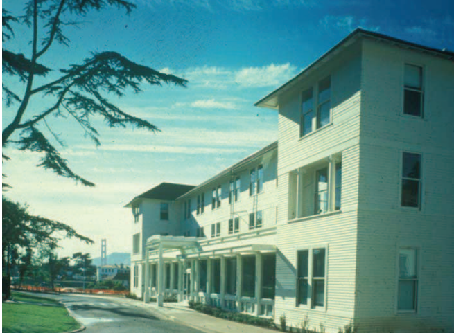
Figure 111: Tall, operable windows such as these at the Thoreau Center allow occupants to take advantage of available natural daylighting and ventilation
