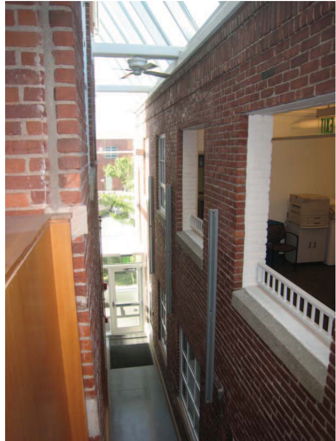
Figure 100: View from one of the removed windows into the glass enclosure
