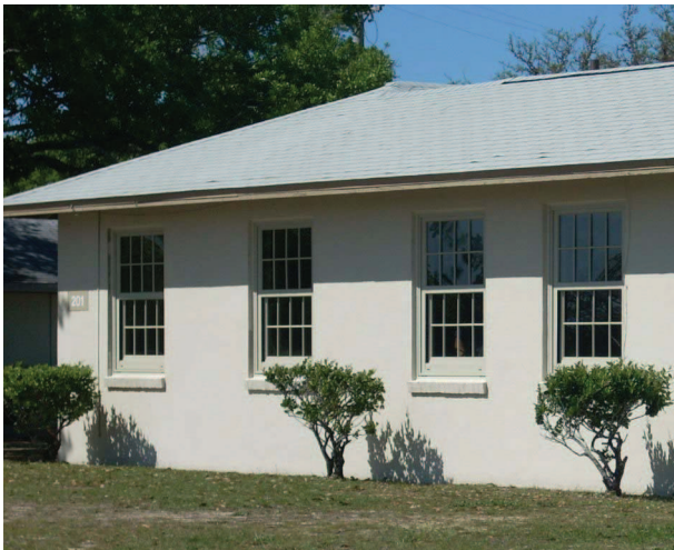
Figure 6: Historically sensitive double-hung replacement windows
