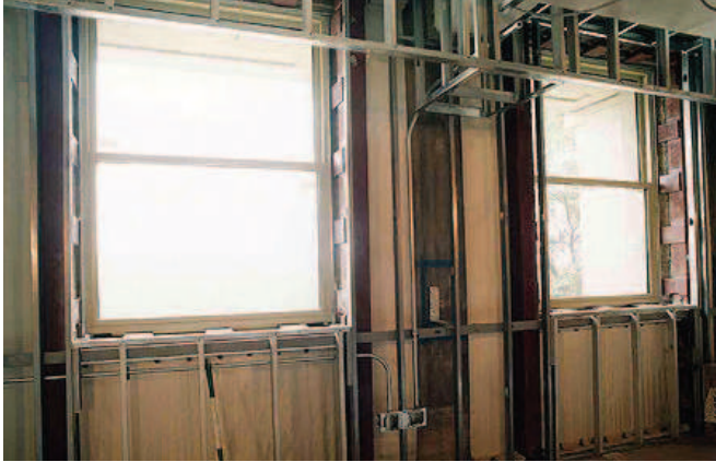
Figure 72: Pentagon, new windows in wall prior to adding insulation
