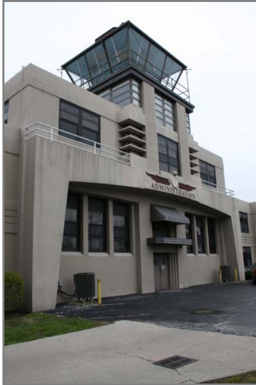
FIGURE 4-2. FRONT FAÇADE, WEST ELEVATION OF BUILDING 5
