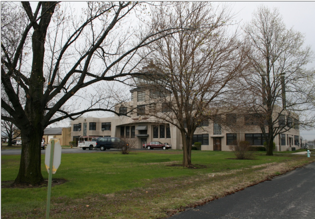
FIGURE 4-1. VIEW OF BUILDING 5, WEST ELEVATION
