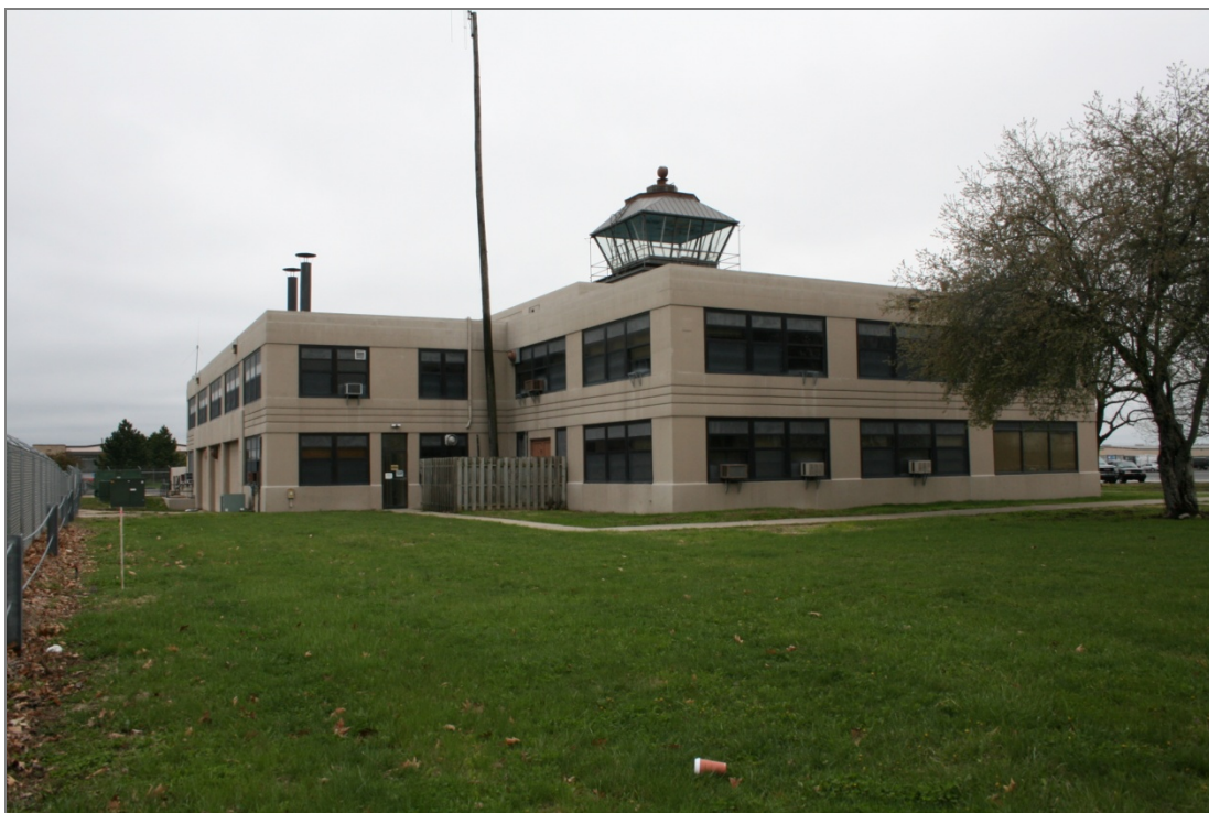
FIGURE 4-3. VIEW OF EAST AND NORTH ELEVATIONS OF BUILDING 5
