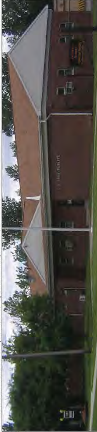
Plattsburg, NY USARC. Built in 1956 using the 1952 standard plan for a 400-3Mm USARC. Note the pitched roof added over the original flat roof in 2000.
