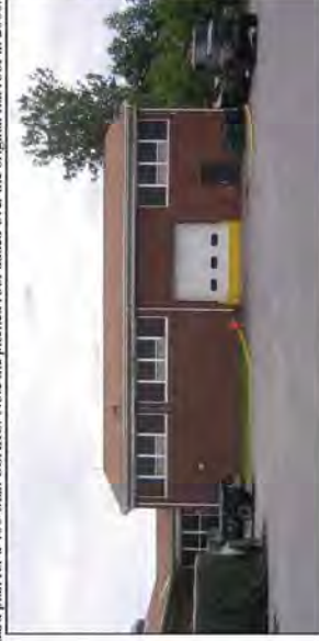
Plattsburg, NY USARC. Built in 1956 using the 1952 standard plan for a 400-3Mm USARC. Note the pitched roof added over the original flat roof in 2000.
