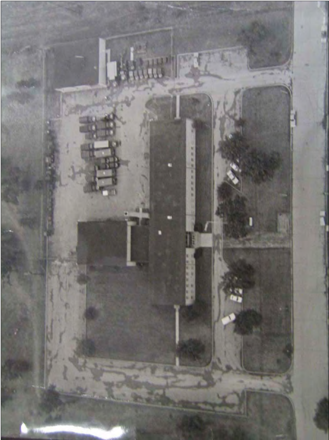
Figure 4.3.6. Aerial photo showing the Tonawanda, NY USARC (courtesy of Ravi Ajodah, 77 th RRC).
