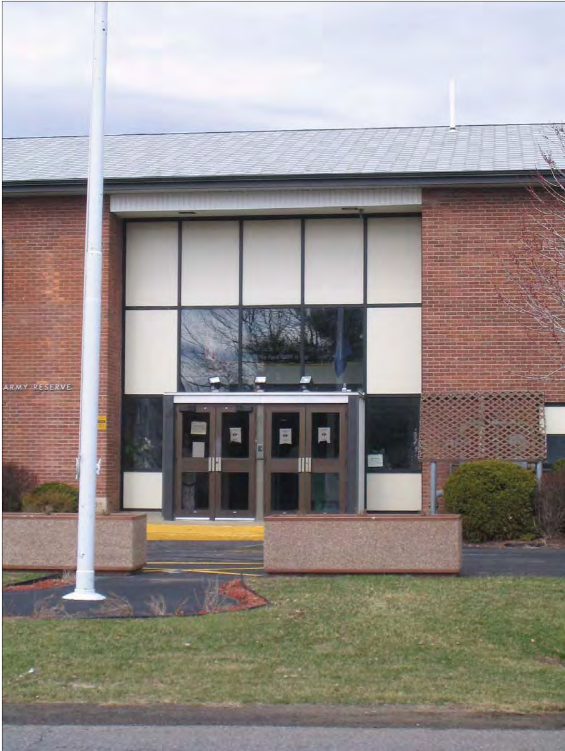
Figure 4.3.14. Photograph of entrance assembly at the Schenectady, NY USARC, circa 2005 (courtesy of Ravi Ajodah, 77 th RRC).
