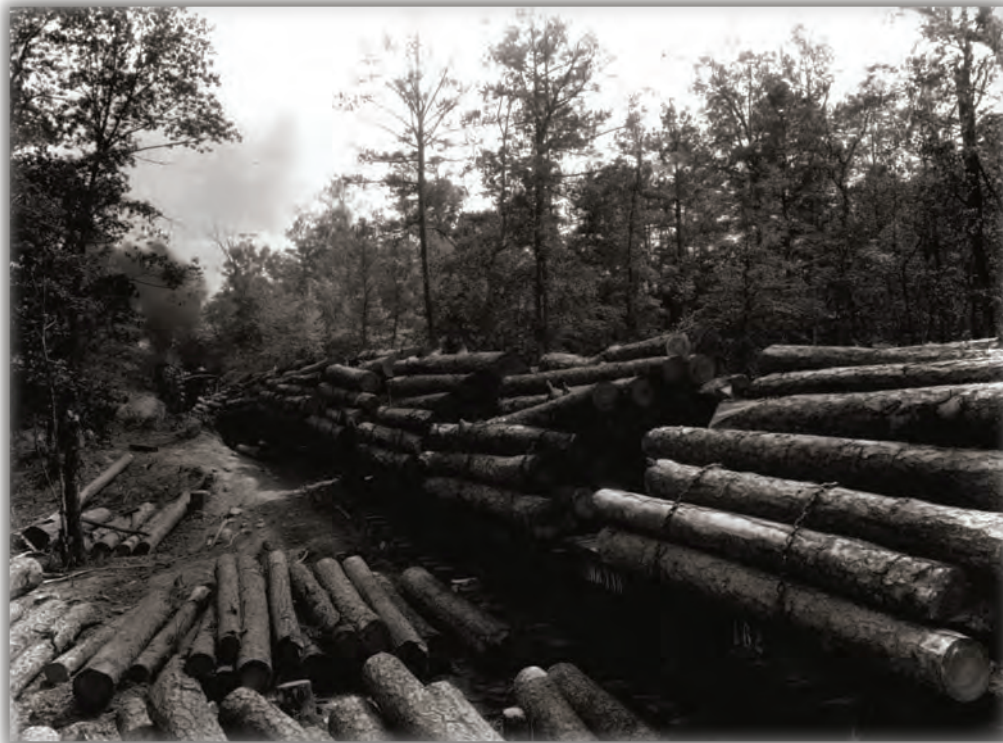
Skidway Associated with a Logging Railroad. Logs are arranged in rows parallel to the track for loading. Arkansas, Unknown Date (U.S. Forest Service).
