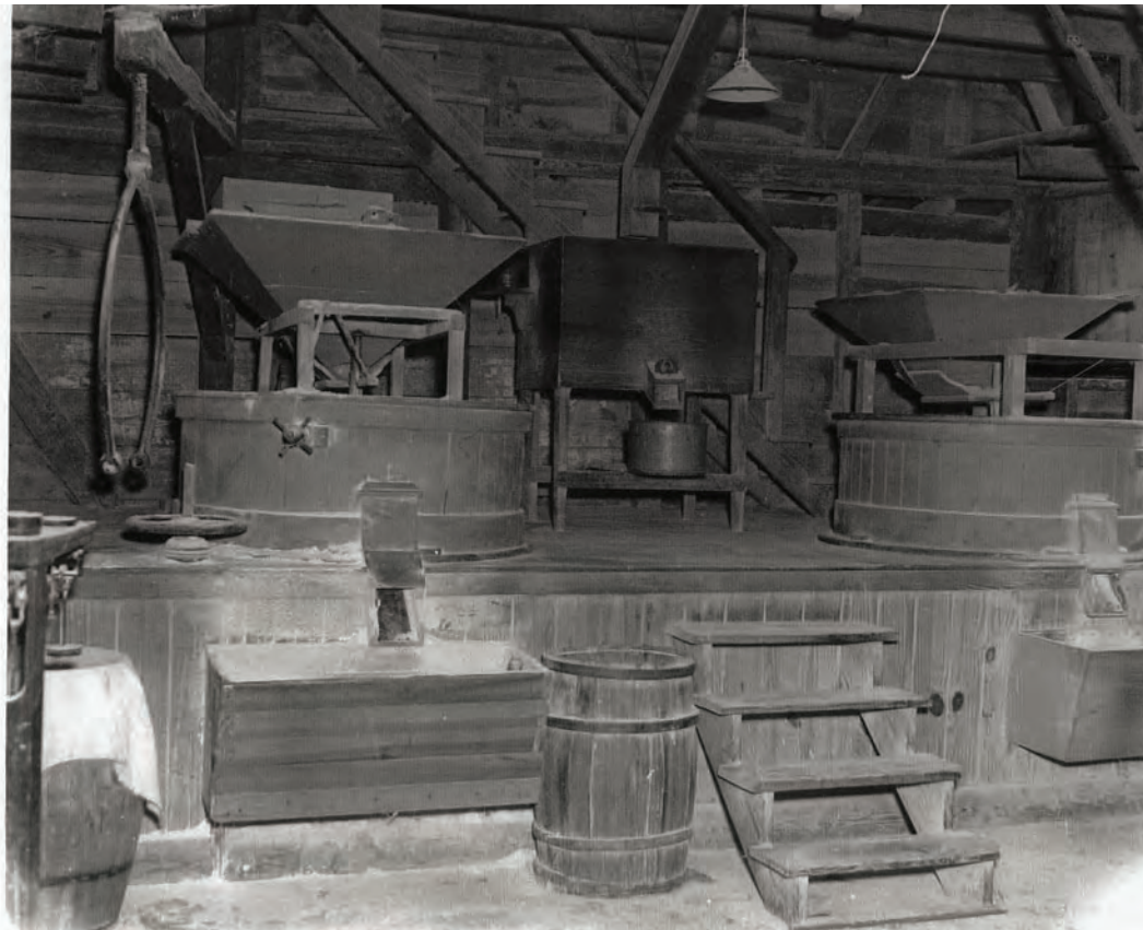
Interior of Leitner Mill Showing the Stone and Meal Floors. Fort Gordon, Richmond County, Georgia, circa 1940 (courtesy of Fort Gordon).
