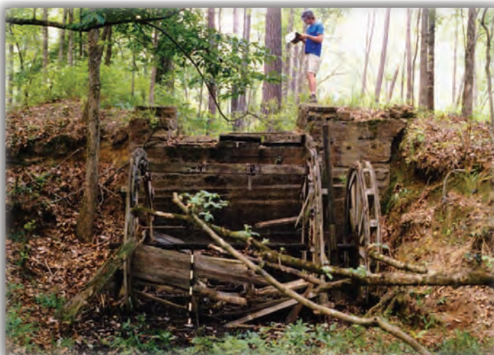
Overshot Wheel, Woodruff Mill (Site 9CE1735), Fort Benning, Chattahoochee County, Georgia (Cowie 2000).
