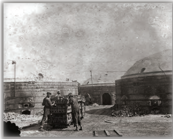
Round "Beehive" Kilns at a Large Brick Plant, Florida, Unknown Date. The same construction would be used at smaller rural brickyards. (Florida State Library).
