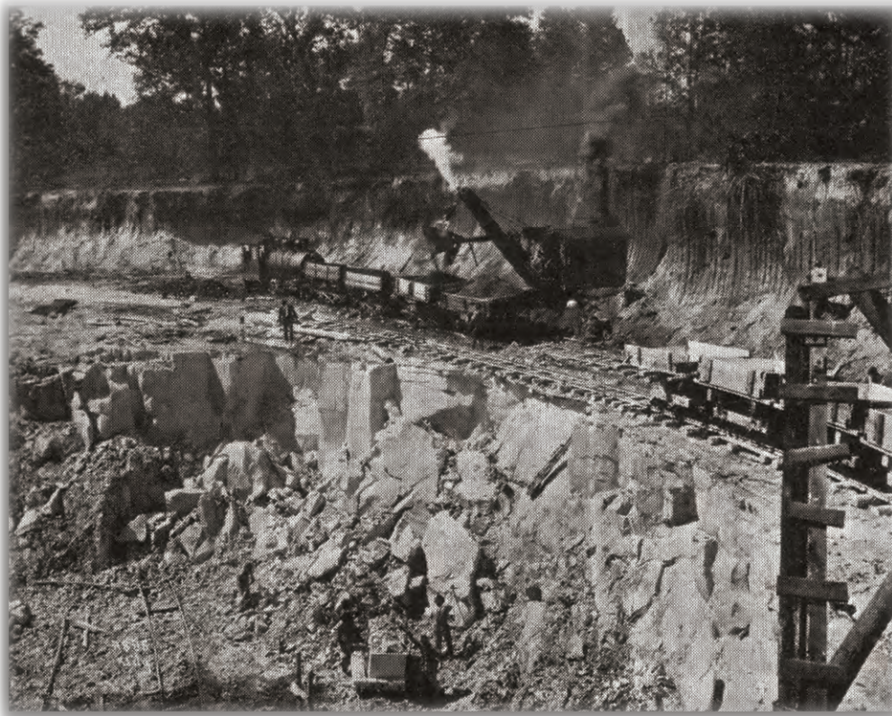
Machine-Excavation of Kaolin Mine Overburden. In the mine below, workers excavate by hand. Vicinity of McIntyre, Georgia, circa 1920s (Stull 1924).
