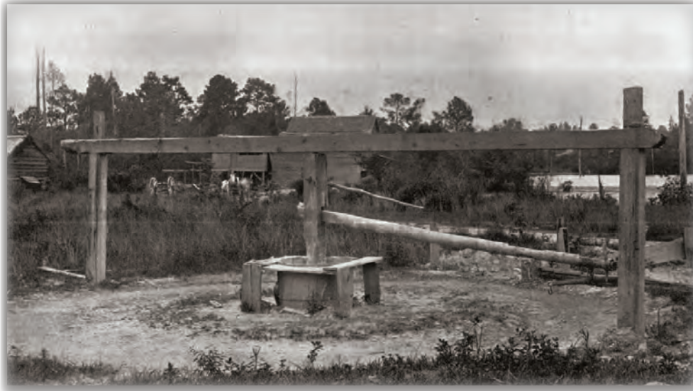
Pug Mill at a Small Country Pottery. Crawford County, Georgia, 1890s. (Ladd 1898).
