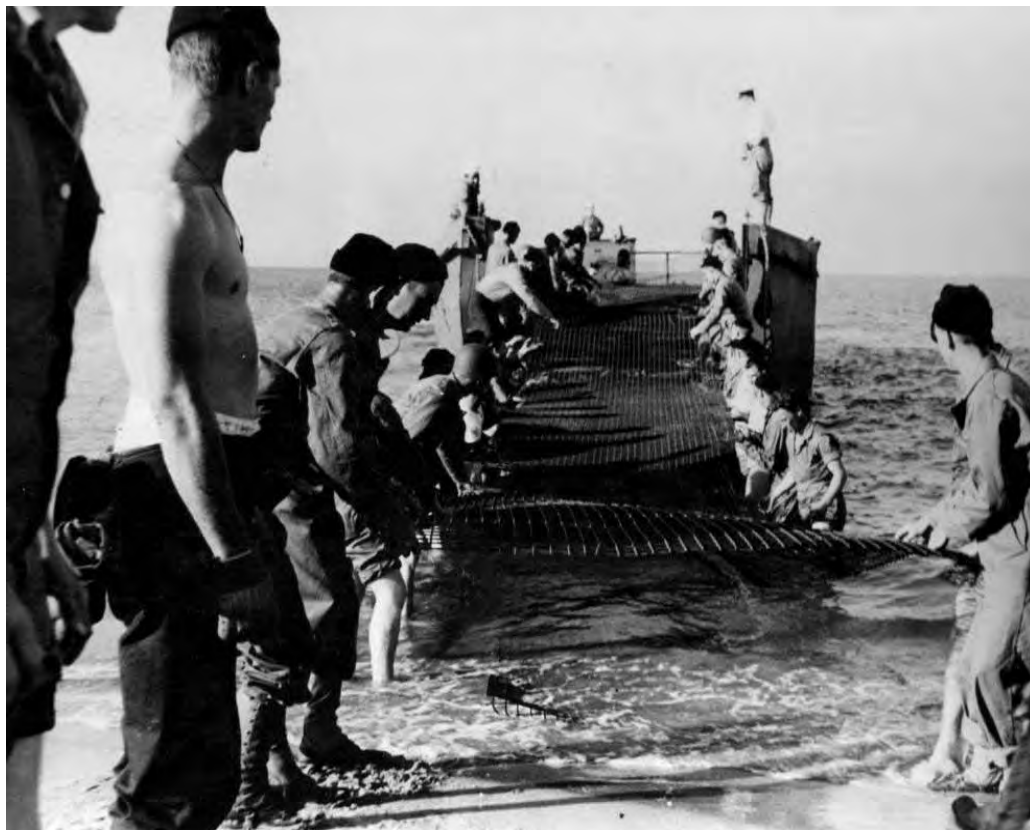
Figure 213. Seabees training with men laying a landing strip from boat to beach for unloading tanks at unknown location, 8 October 1943 (NARA College Park, RG 80-G, box 377, photo 82513).
