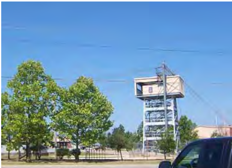
Figure 335. Parachute jump tower, Fort Bragg, NC, 18 May 2006.
