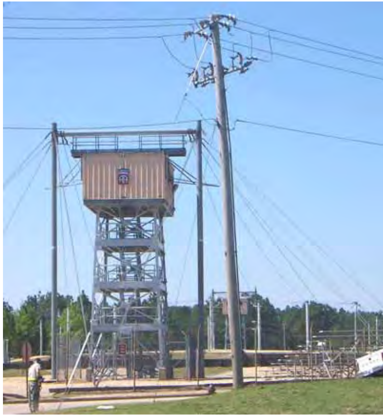
Figure 334. Parachute jump tower, Fort Bragg, NC, 18 May 2006.
