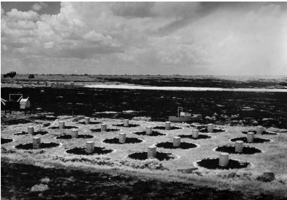
Figure 108. Oil tanks in the mock Tokyo bombing range at Midland Army Air Field, TX, 4 July 1942 (NARA College Park, RG 342-FH, box 2202, photo 4A-17188).
