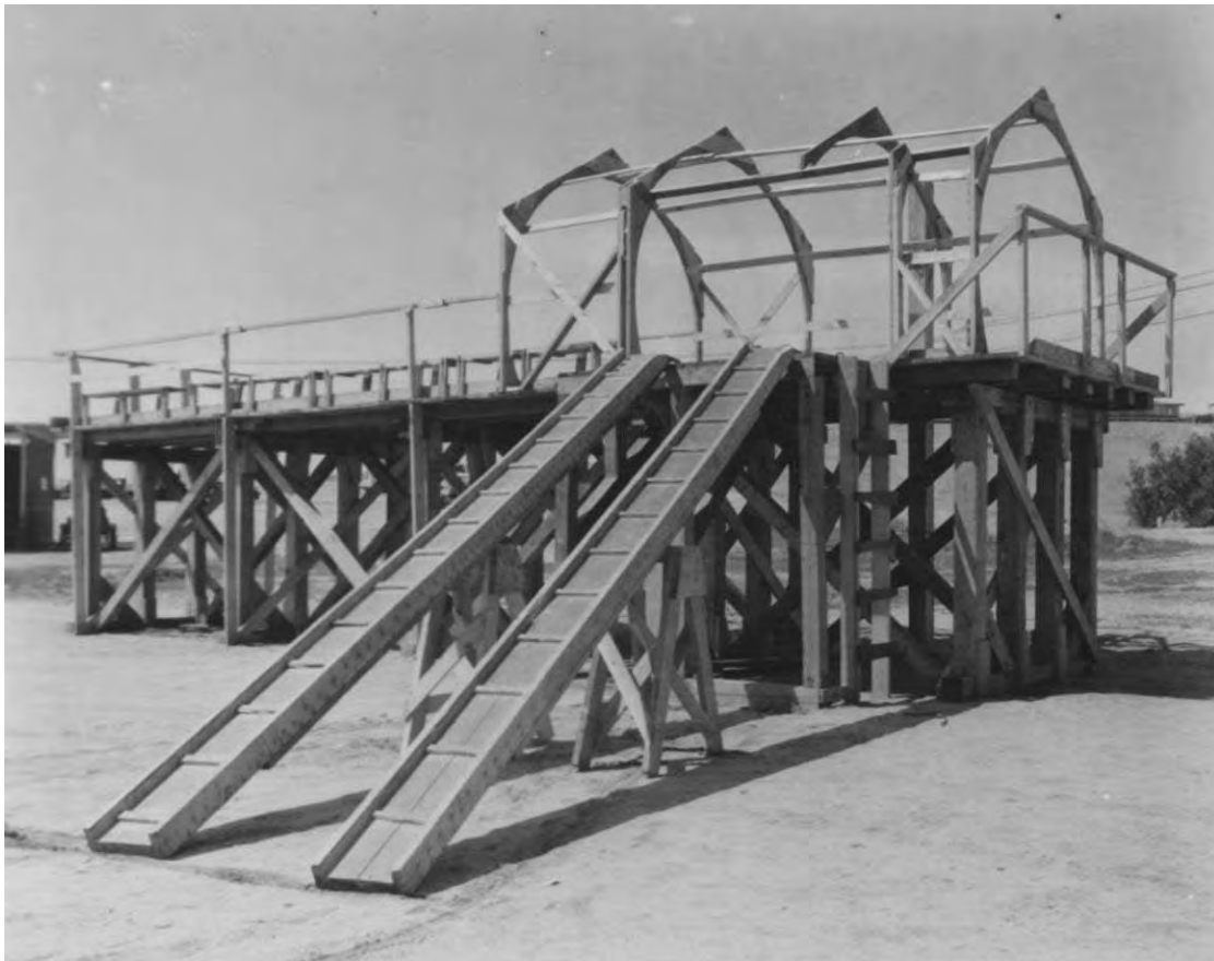
Figure 88. Mock up of cargo hatch and interior of R5D cargo plane at Camp Pendleton, CA, 23 March 1948 (NARA College Park, RG 127-GC, box 11, photo 407108).
