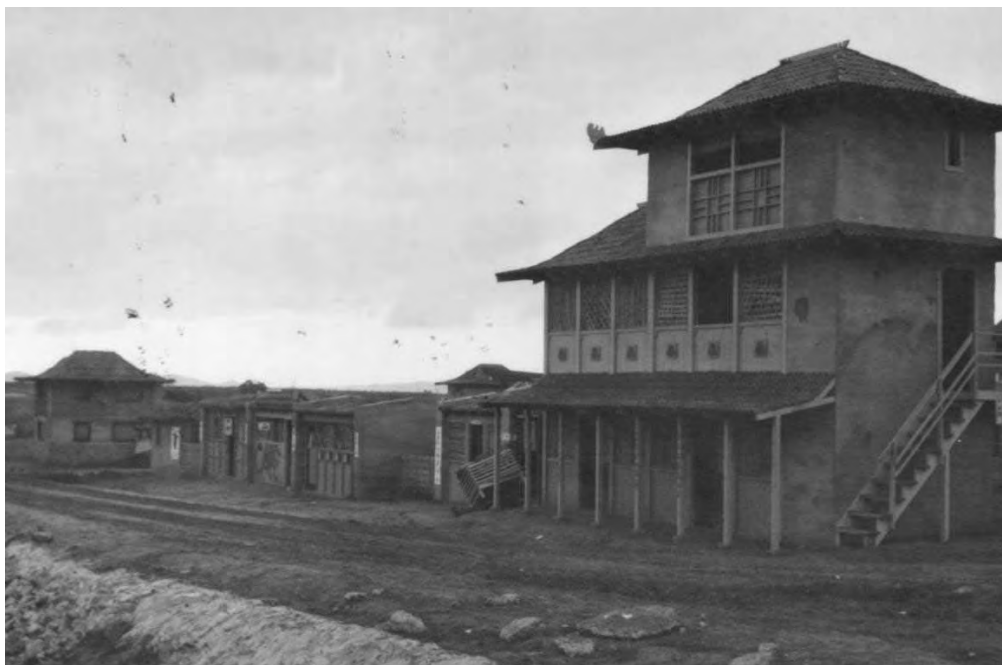
Figure 25. An Oriental combat town at Camp Pendleton, CA, 16 December 1952 (NARA College Park, RG 127-GC, box 11, photo A350100).
