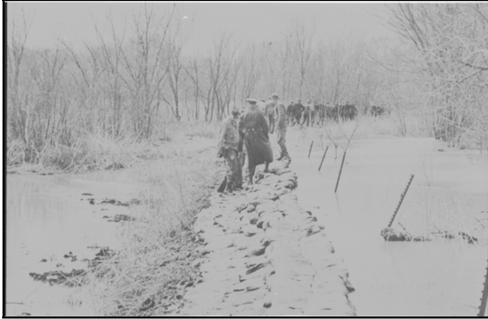
FIGURE 7-14. GERMAN POWS AFTER STACKING SANDBAGS TO FIGHT A FLOOD NEAR OMAHA, NEBRASKA, APRIL 1944 (NARA 308A-Q—UNOFFICIAL IMAGE FROM ARMY PICTURE SERVICE [ROLL #5-3])
