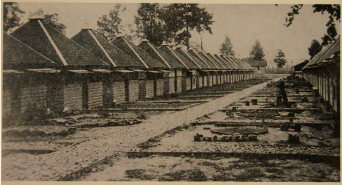
View of POW hutments showing graveled walkways and garden plots (Tulahoma Fine Arts Center)
