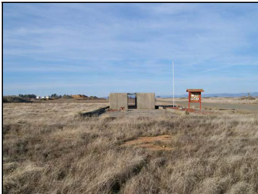
General Setting of Building #245, looking north (Cheever/Berryman 2007)
