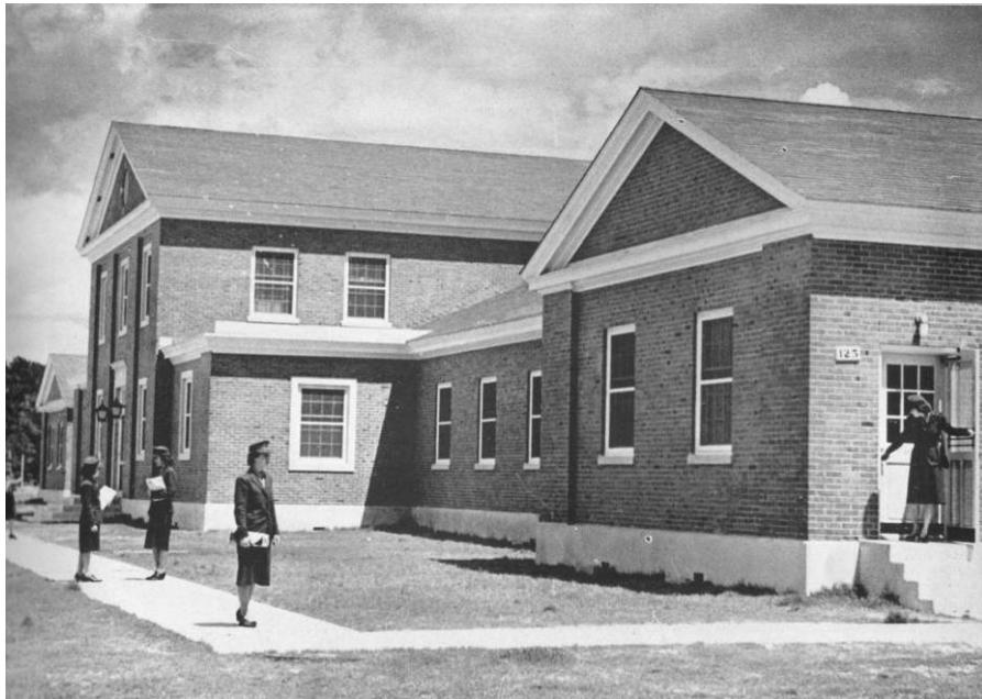
Figure 10. WAC area building, Camp Lejuene, 1943 (WIMSA, Document File, Collection of Lyla Spelbring).
