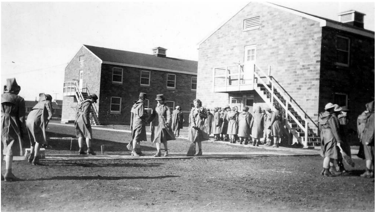
Figure 42. WAC barracks area showing fire escape stairs, Fort Des Moines, 1942 (WIMSA, Vertical Photo File, Collection of Ruth Sparacio).
