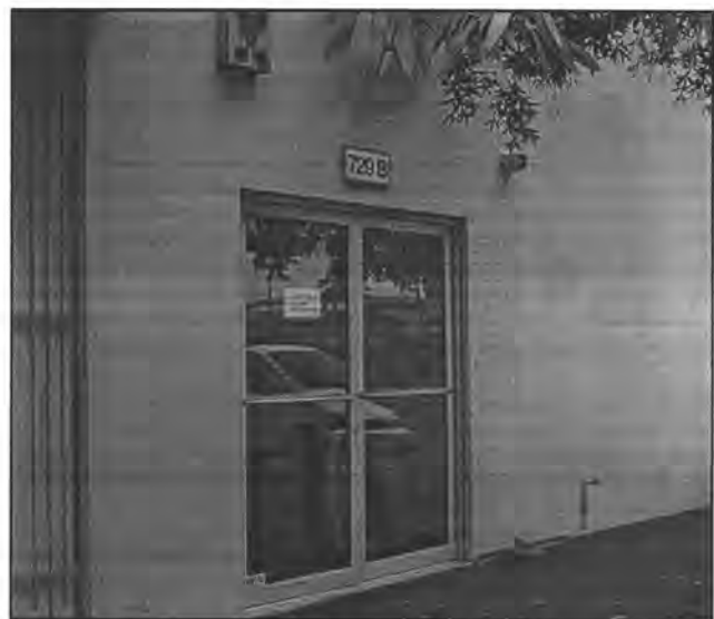
Figure 67. Exterior of the building where Garcia and Associates is located.
