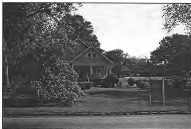
Figure 102. New South Associates offices are located in an 87 year old wooden structure.
