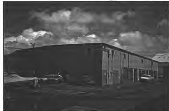
Figure 80. Exterior view of the commercial storage building, Building J, where International Archaeological Research Institute, Inc. rents space to house their collections.
