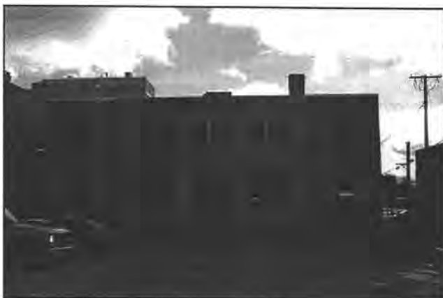
Figure 130. The offices of SWCA, Inc. are located in Flagstaff in a former federal building.
