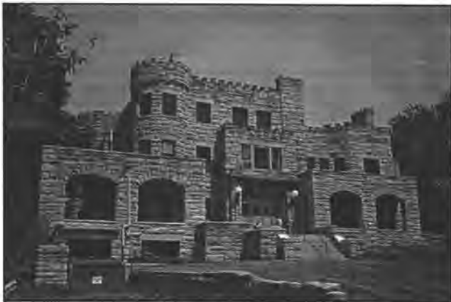
Figure 84. Exterior of the Kansas City Museum's Annex Administration building.
