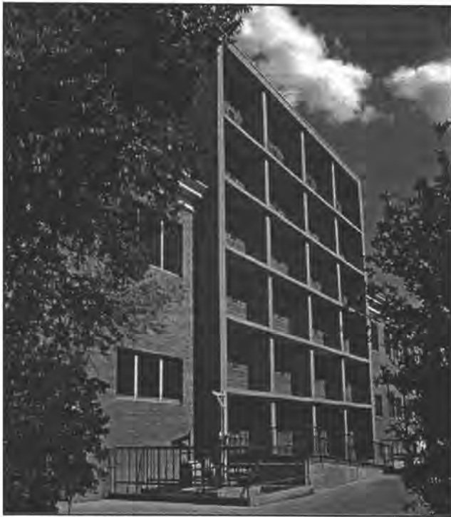
Figure 43. The Matthews Center on the campus of Arizona State University houses artifact collections from Williams Air Force Base.
