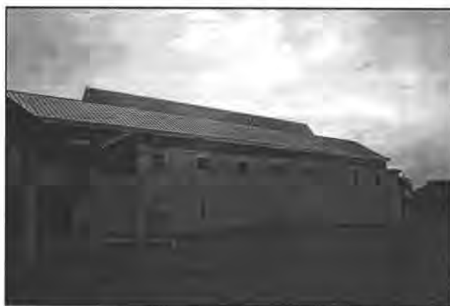
Figure 87. The Kansas Historical Museum Center for Archaeological Research building is cement with a standing seam roof.
