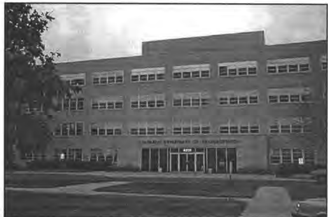
Figure 61. Exterior view of Colorado Department of Transportation.
