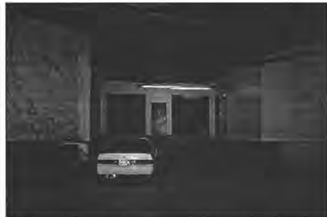
Figure 85. Interior entrance to the storage space within the Downtown Underground Dock "cave" system.
