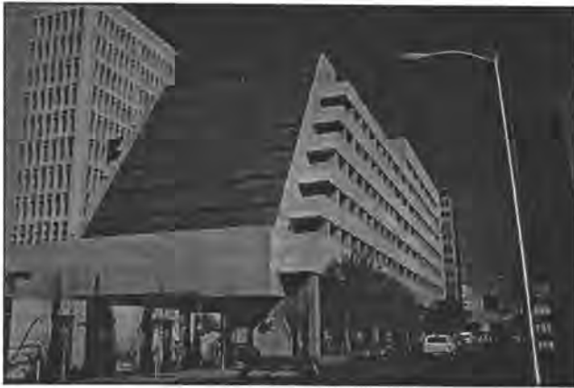
Figure 120. Public Service Company of New Mexico headquarters building is located in downtown Albuquerque.
