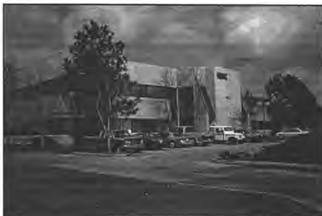
Figure 71. The offices of Gulf South Research Corporation, a private engineering firm.
