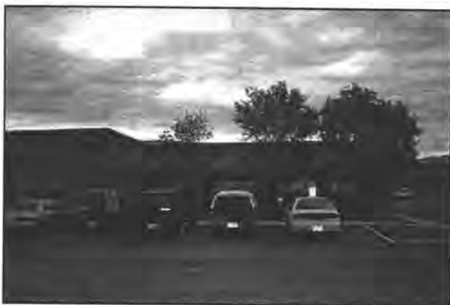
Figure 136. The offices of TRC-Mariah Associates are located in an industrial park on the northeast side of Albuquerque.
