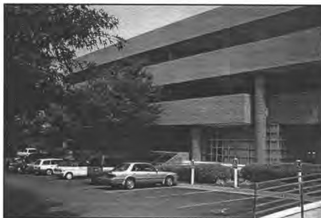
Figure 114. Parsons Engineering Science is a private contract engineering firm that conducts work for various Department of Defense installations.
