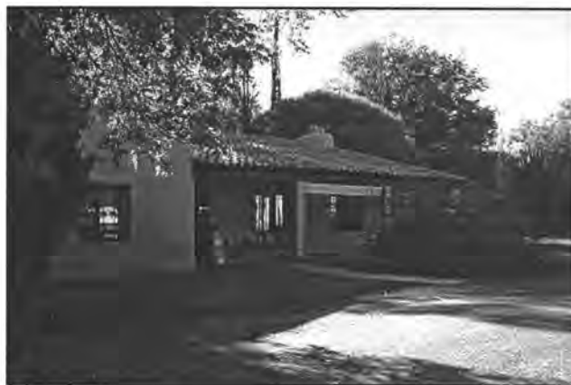
Figure 77. The Human Systems Research office in Tularosa is located in an adobe and stucco building with a clay tile roof constructed around 1900.
