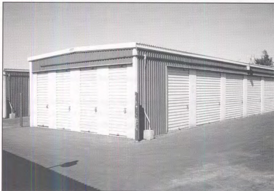
Figure 12. Exterior view of FWARG repository 2.
