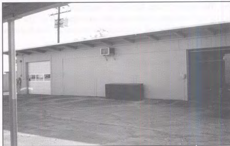
Figure 14. Exterior view of the Joshua Tree National Monument curation repository.
