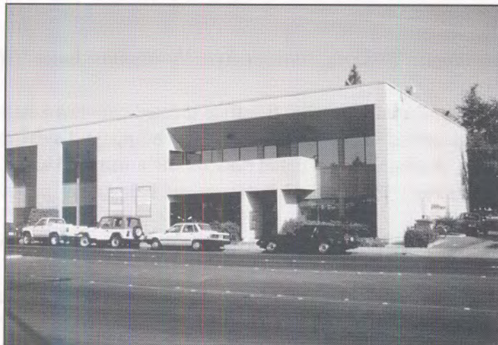
Figure 11. Exterior view of FWARG repository 1.
