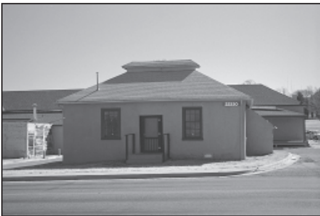
Figure 2. Building 22330 is a 900 square foot adobe building constructed in 1884; it originally served as a magazine.
