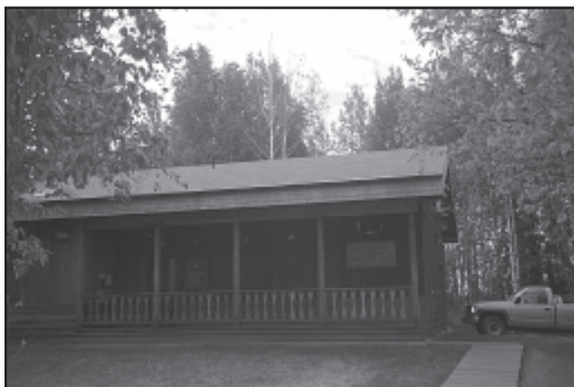
Figure 1. View of the exterior of the Natural Resources building at Eielson Air Force Base.
