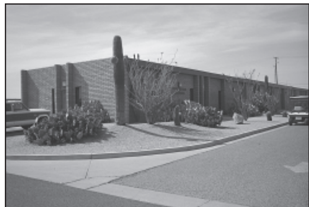
Figure 6. Building 302 on Luke Air Force Base houses the Environmental Impact Analysis Section.
