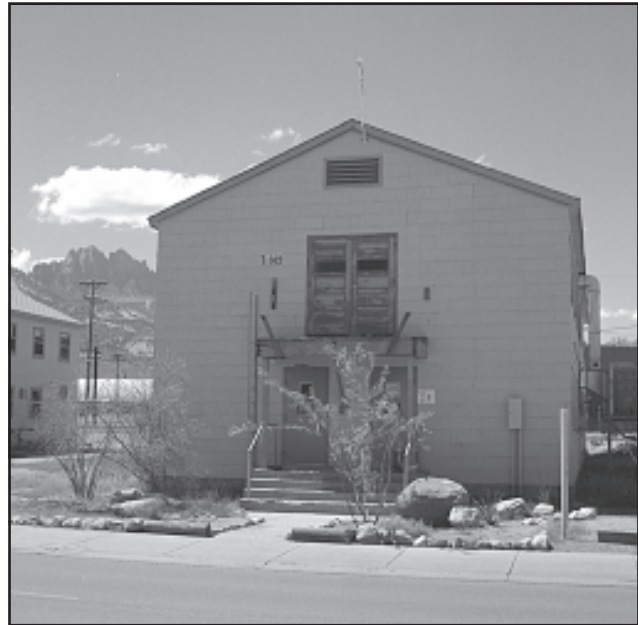
Figure 19. Building T-149 (repository 1), originally built during World War II as temporary barracks, presently houses offices of the Natural and Cultural Resources Division.
