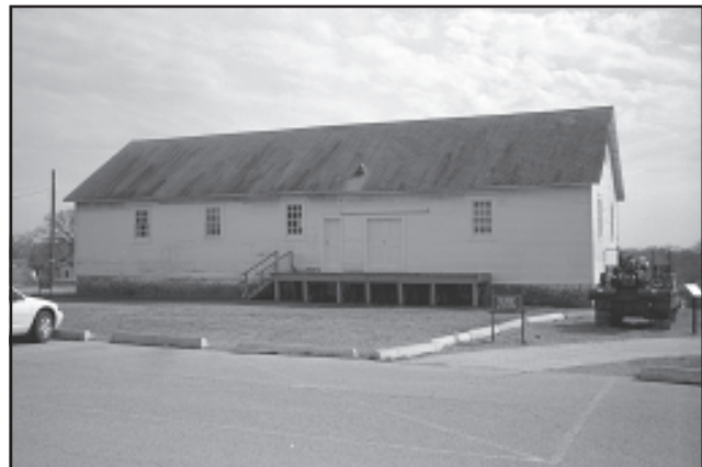
Figure 23. The Quartermaster Granary on Fort Sill has been converted to serve as an artifact repository.
