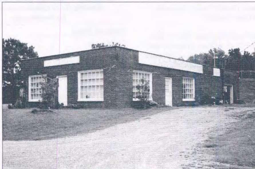
Figure 6. Exterior view of JRIA.
