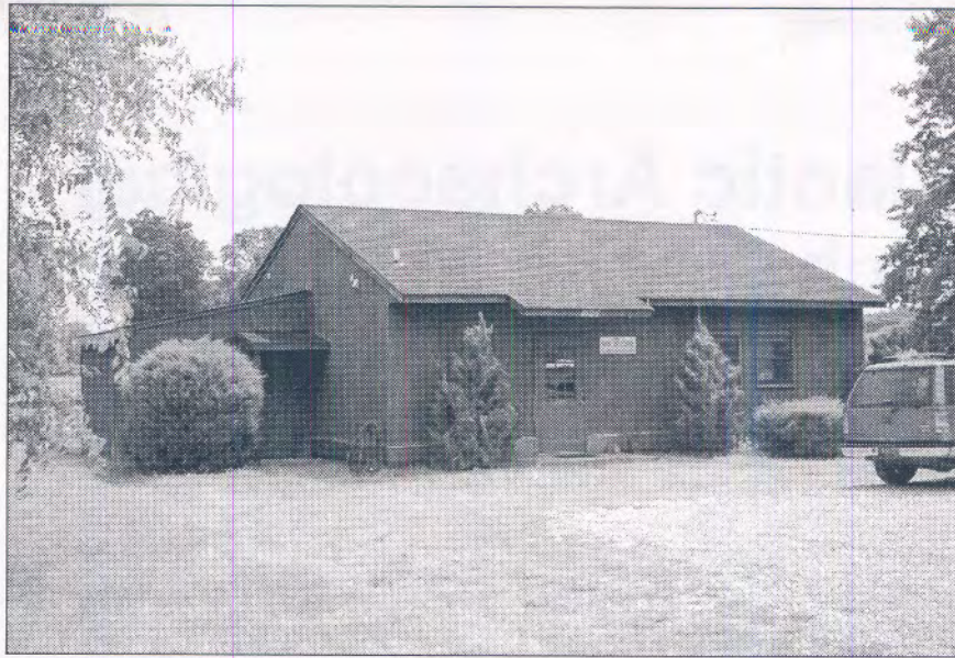
Figure 10. Exterior view of MAAR.
