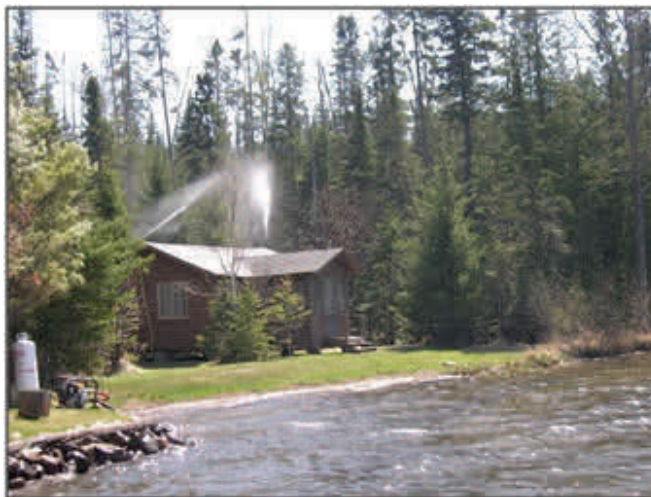
Private home sprinkler in Minnesota. Credit: Northeast Region
