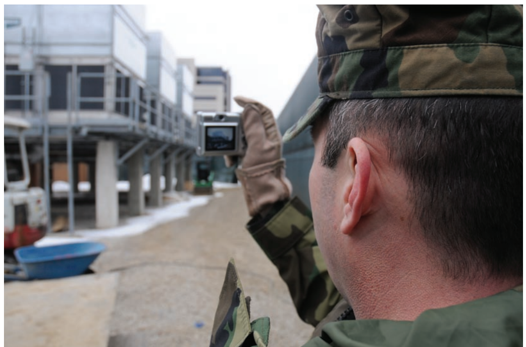
(left) JSIVA 4 during a recent mission in Iraq. (below) When Navy Lt. Cmdr. Max Sisson looks at an installation’s infrastructure, he looks at everything, including cooling systems.
