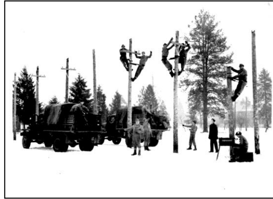
Wiring for communications security (training).
