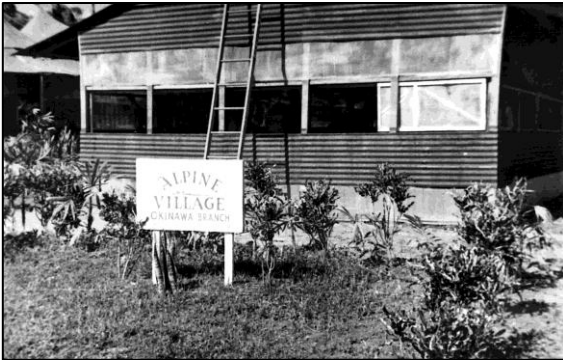
Alpine Village, Okinawa mess hall. Ladder was property of electricians, not permanent fixture.
