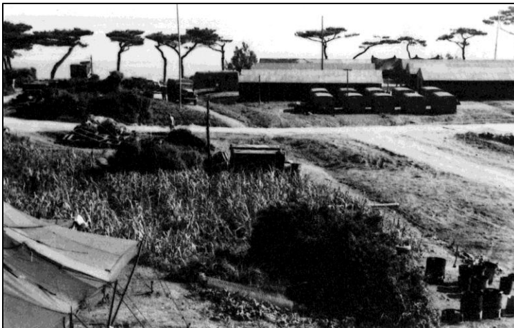
Operations Building and TC-8s, TC-9s.
