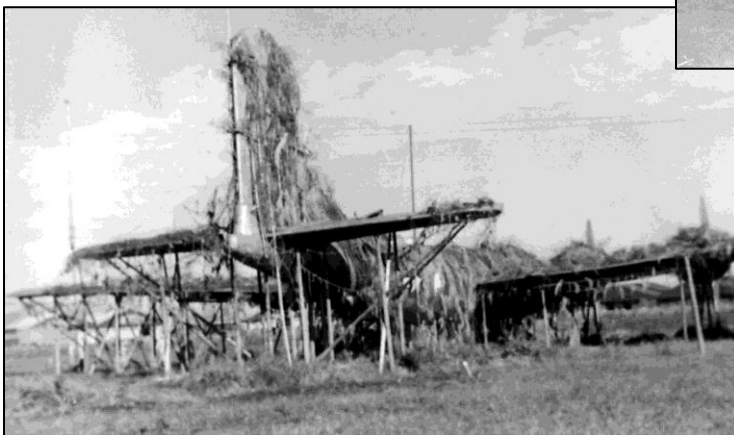
Fake B-29 Superfortress heavy bomber the Japanese had constructed, found in a field near our camp. It was complete with markings.
