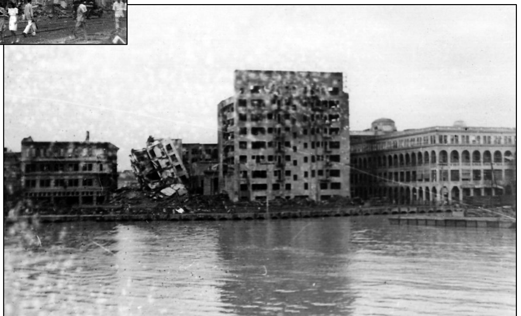
Destroyed and abandoned buildings in Manila.
