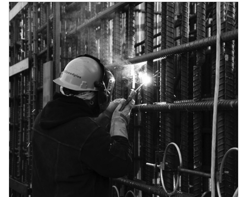
A worker welds rebar ties on the WTP pretreatment facility.
