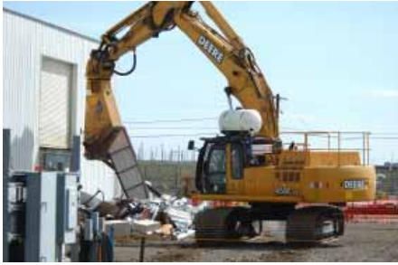
Demolishing the 241-Z Liquid Waste Facility.
