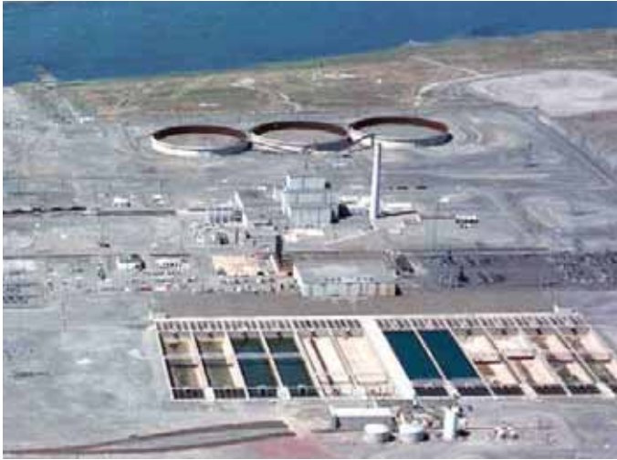
Aerial view of the K-Basins. Radioactive waste was removed from K East Basin in 2007.
