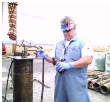
Left: Workers inject chemicals into the ground to form a mineral barrier that traps contamination in the soil before it reaches the Columbia River.
