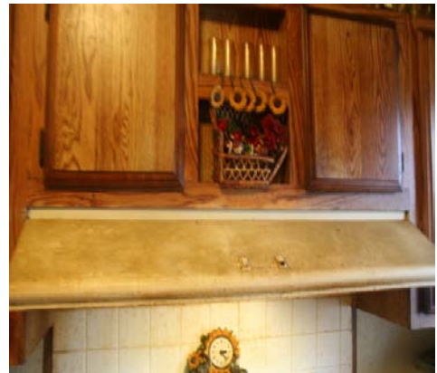
Excessive grease build-up on the stove hood and wall
