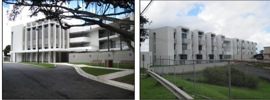
Partial views of the main entrance of the project and 27 housing units constructed
