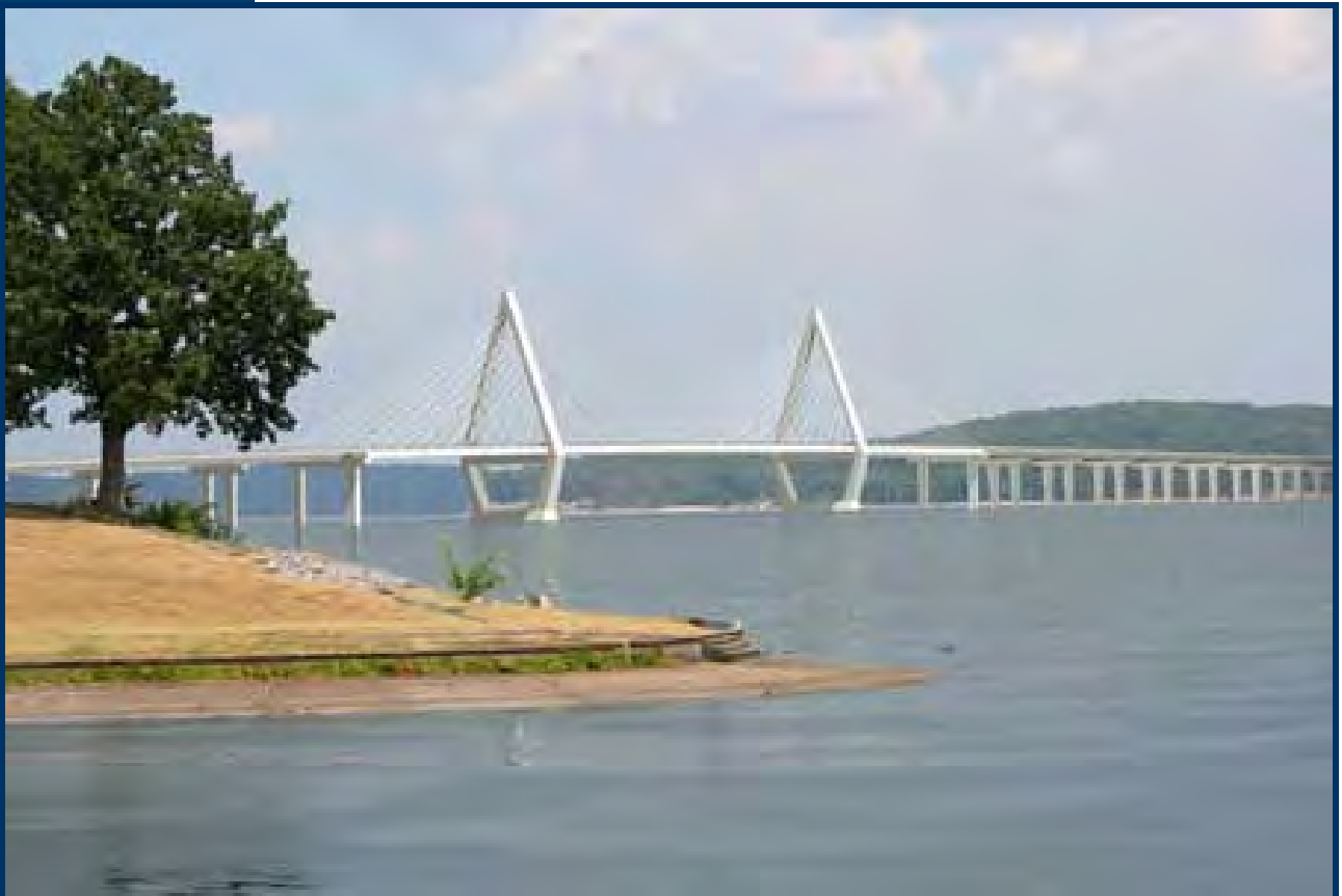
POTENTIAL TWO DIAMOND TOWER CABLE STAY BRIDGE DESIGN FOR US 68/80 LAKE BRIDGES
