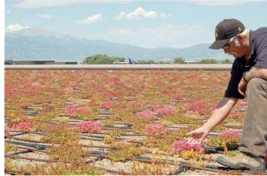
Phil Chase monitors Sedum plants on the vegetative rooftop of the 21st Space Wing headquarters building at Peterson Air Force Base, Colo. Heat is redirected through the plants instead of the rooftop, cooling the inside of the building. The building's roof is about 67 degrees cooler than the nearby 21st Mission Support Group building. Mr. Chase is the solid waste and hazardous materials program manager for the 21st Civil Engineer Squadron Asset Management Flight. (U.S. Air Force photo/Thea Skinner)
