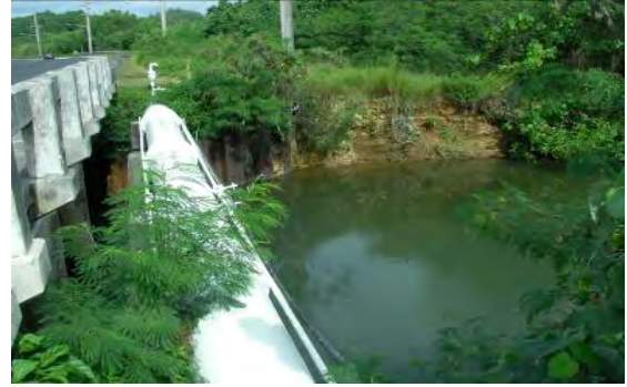
Figure F-4: Rte 1 at Atantano Bridge
