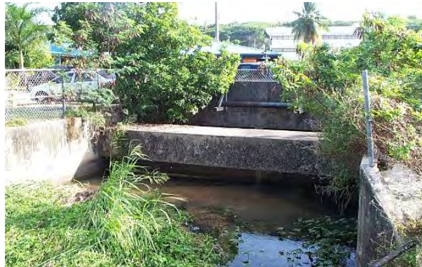
Figure 6 Tamuning Drainageway Outlet
