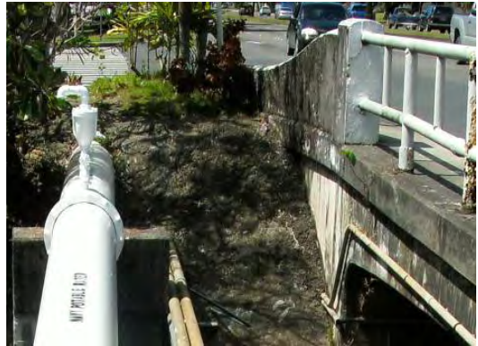
Figure F-1 Agana Bridge Upstream Embankment
