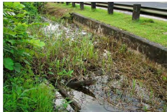
Figure F-3 Agueda Bridge Downstream Obstructions
