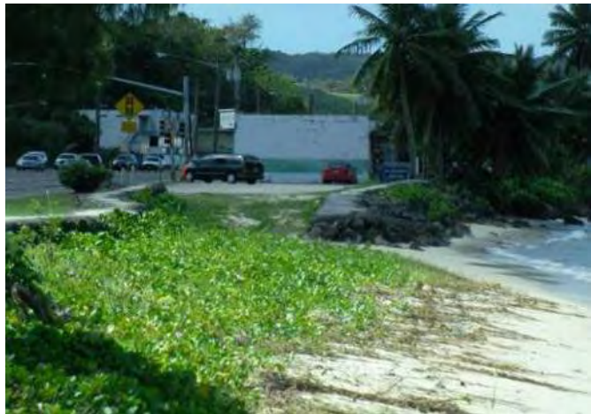
Figure 17: Coastal Erosion Protection along Rte 1
