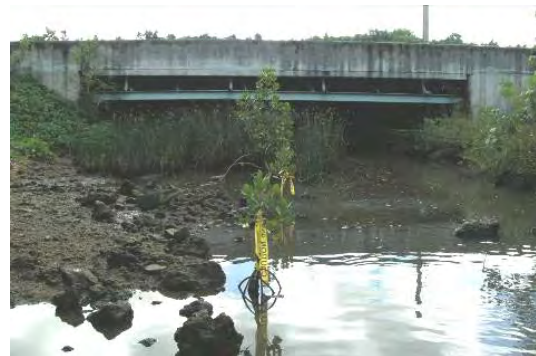
Figure F-2 Laguas Bridge Upstream Section
