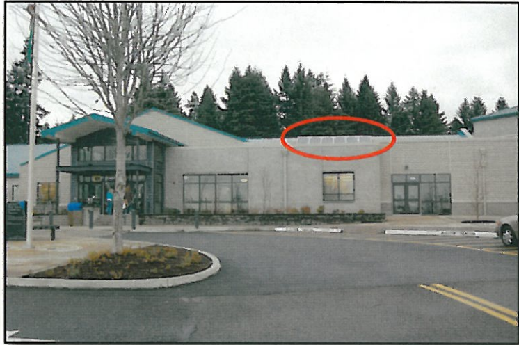
1.1 kW roof-mounted PV system at La Center High School
