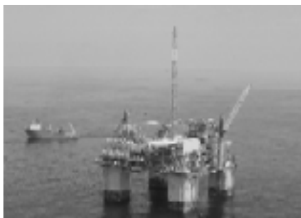
Figure 17: Na Kika, Floating Production Facility in the Gulf of Mexico Region
