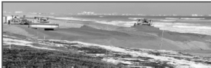
Figure 24: The picture to the left shows restoration efforts using OCS sand resources on Patrick Air Force Base near Coca Beach, Florida.
