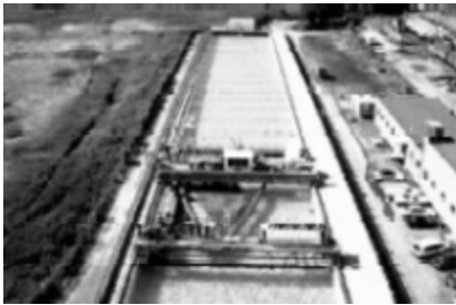
Figure 33: Ohmsett facility in New Jersey.
