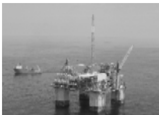
Figure 29: Na Kika – Gulf of Mexico Region Floating Production Facility
