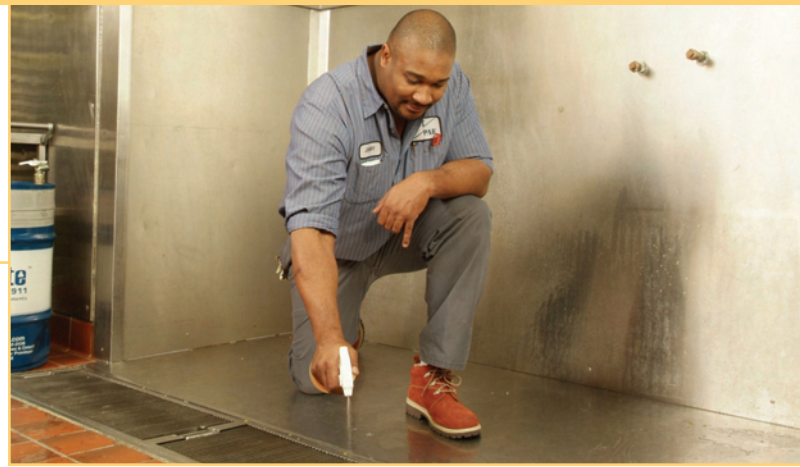
DRAIN CLEANING: Jim Nolan, a long-time employee of USDA’s maintenance contractor, Capitol Technology Services Inc., uses a soy biobased drain cleaner in a South Building cafeteria kitchen. “This product really works,” says Nolan. “It keeps the drain clear, cuts grease and eliminates slime while being biodegradable, non-acidic and non-caustic. Not bad when your major aim is to control the bugs that feed on food scraps.”
