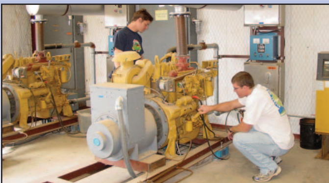
Southern Plains Area staffs have switched to cleaner burning biodiesel in diesel vehicles as well as power stationary engines used to generate electricity as part of the research on wind/hybrid power.
