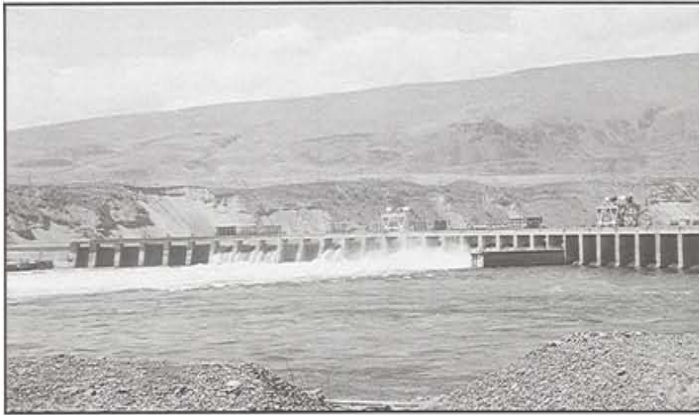
Rock Island Dam
