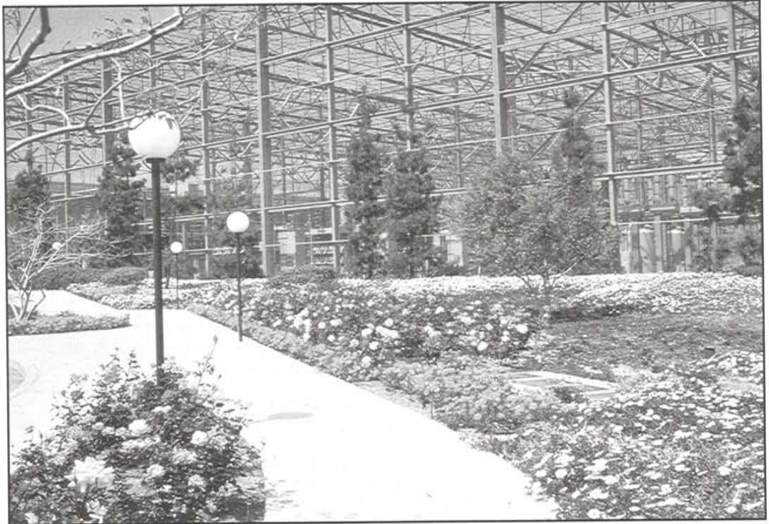
At Sylmar Substation, outside Los Angeles, California, power from the Northwest is often delivered to serve peak summer loads in the Southwest. During high Northwest load periods, power is delivered to Southwest utilities. This substation forms one end of the direct current (DC) intertie transmission link between the two regions.
