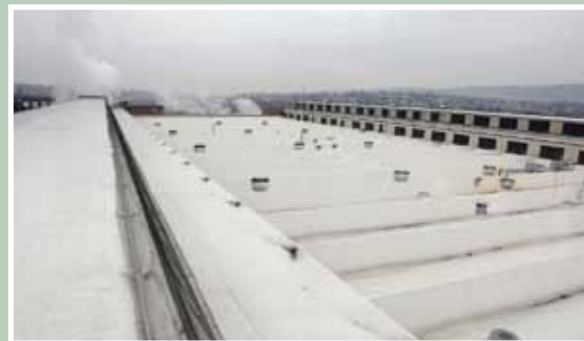
The Production Shop cooling towers provide water to cool equipment and maintain acceptable operating temperatures within SCAAP's production shop. In the past two years, rain water has provided all but 70,000 gallons of water required by the cooling system.
