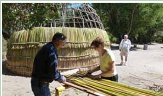
Volunteers working at the Mission La Purisima State Park built a Chumash tule hut with willow poles and tule reeds from the Pine Lakes recreation area on VAFB to clear and re-open multiple access points along the shoreline.
