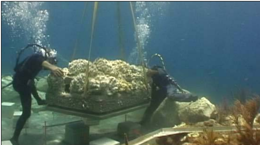
Figure 15 Habitat Replacement Module Deployment Requiring Commercial Dive Operations and Marine Operation Heavy Equipment
