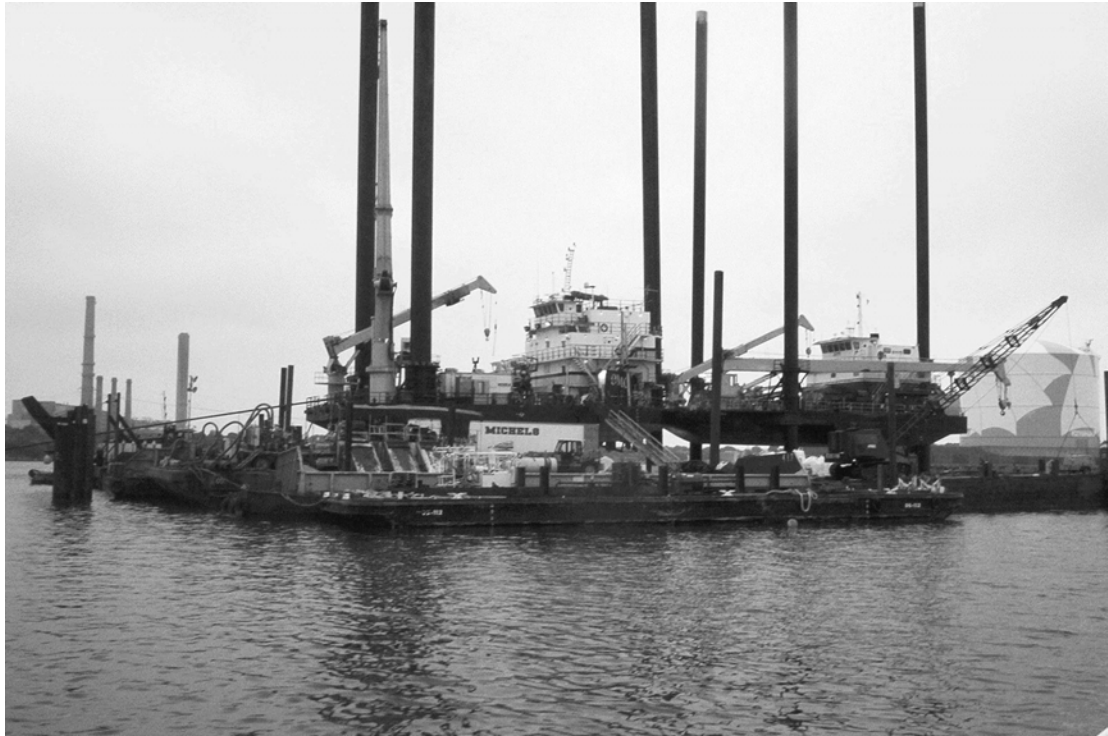
Figure 4 - Lift Boats Ready for Pull-back
