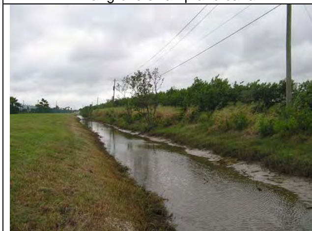
3. W-1: South conveyance ditch, facing east.
