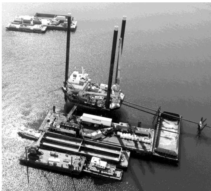
Figure 1 - Typical HDD Marine Spread
