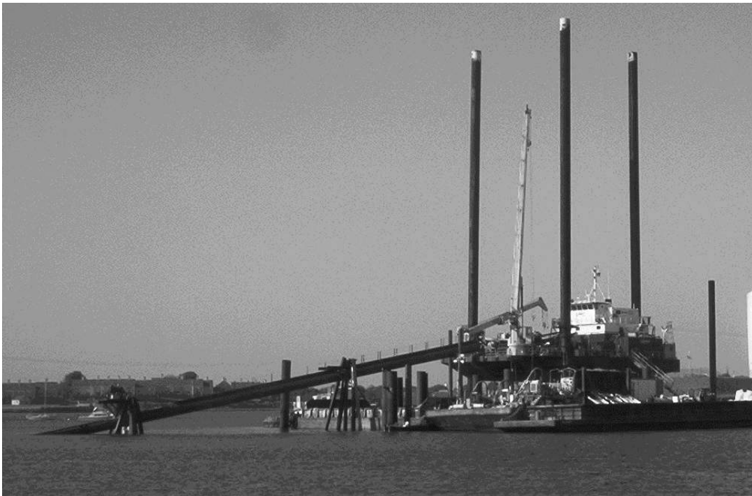
Figure 2 – Typical Marine Riser Structure
