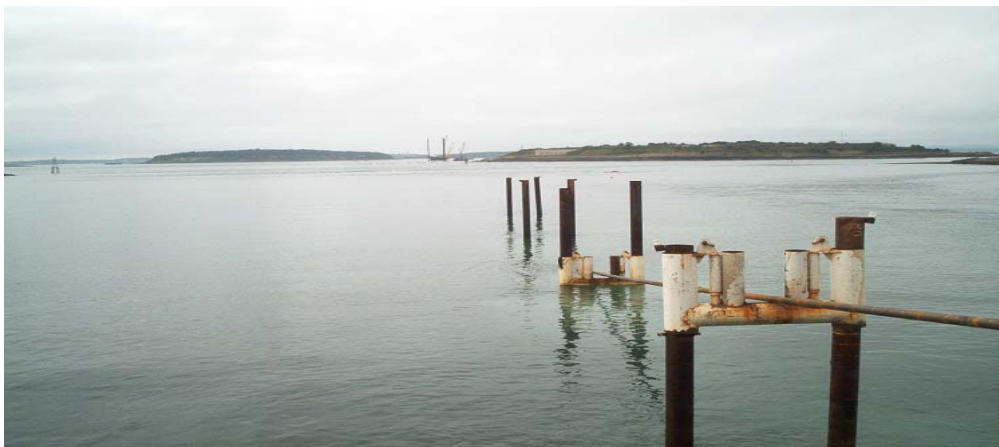
Figure 4 HDD Exit Side Operation – Riser Structure
