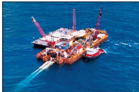
Figure 4-1 Typical Pipelay, Plowing, and Backfill Spread (courtesy of Horizon Offshore)
