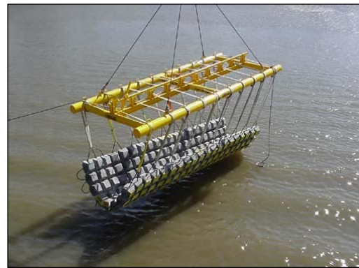
Figure 7 Concrete Mattress on Deployment Frame
