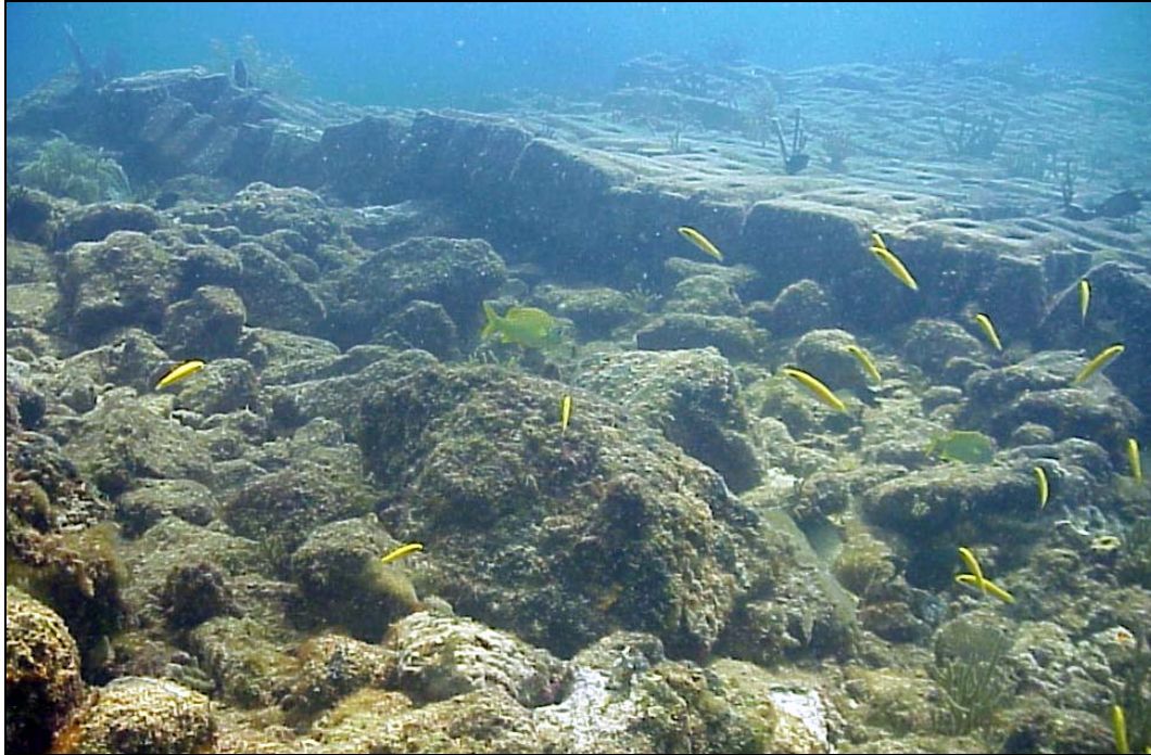
Figure 13 Articulating Mats Similar to Those Being Considered for Mitigation for the Port Dolphin Project for Use as Protective Structures
