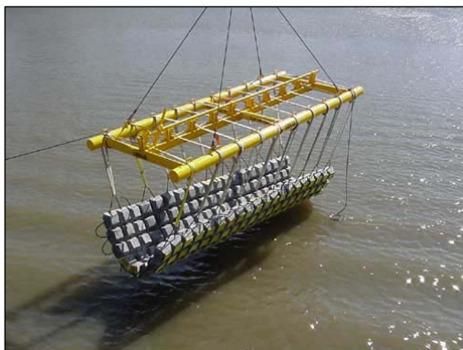
Figure 3-9 Concrete Mattress on Deployment Frame
