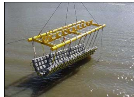
Figure 7 Concrete Mattress on Deployment Frame
