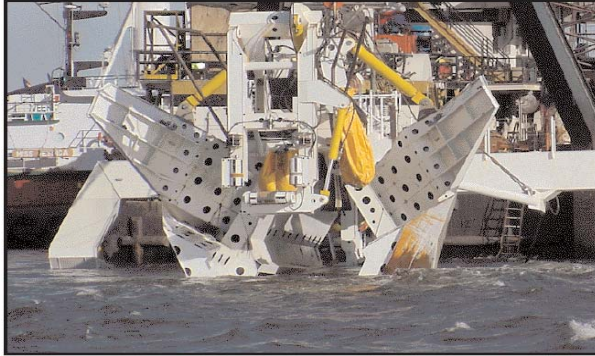
Figure 3-4 A Typical Pipeline Burial Plow (courtesy of Horizon Offshore)
