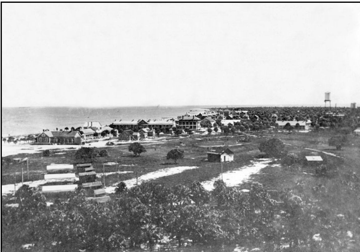
Figure 11. Fort Dade, Egmont Key ca. 1909 (University of South Florida 2002).
