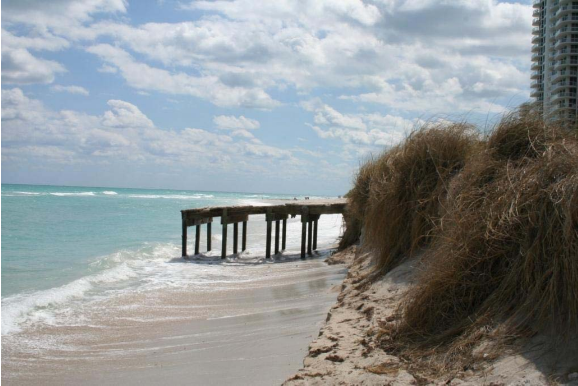
Figure 3 - R-Monument 45 Looking South in February 2009
