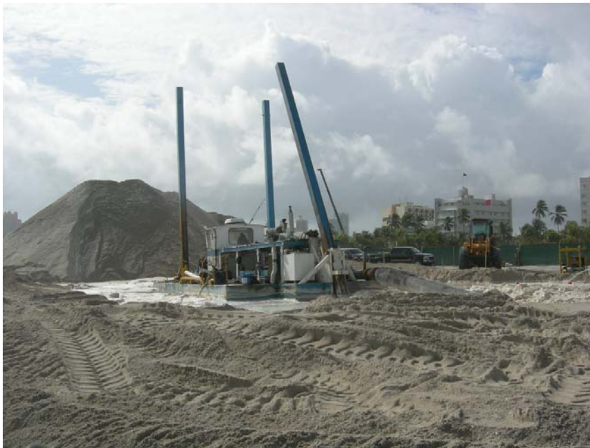
Figure 1.3 Example of Cutterhead Suction Dredge at Lumus Park (Source: COE 2009)
