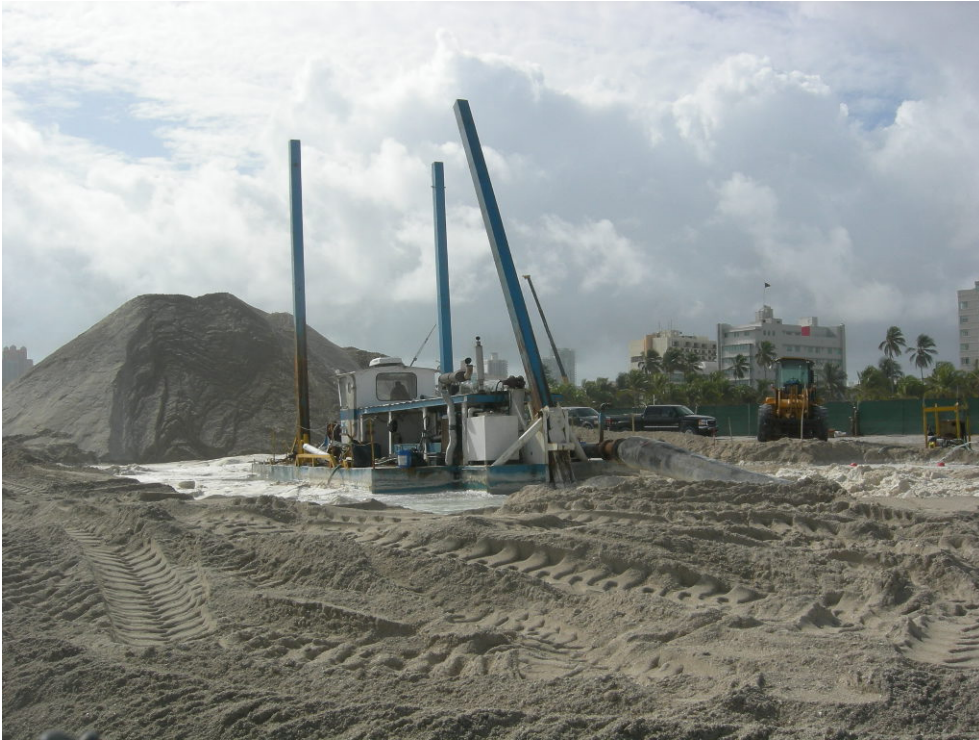
Figure 6 - Dredge on the Beach in Back-passing program at Lumus Park
