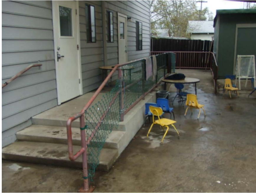
Photograph 3 – Taken at South Ukiah on 3/31/10 showing a chain-link fence on steps leading to the outdoor play area that was not properly fastened to the top railing.
