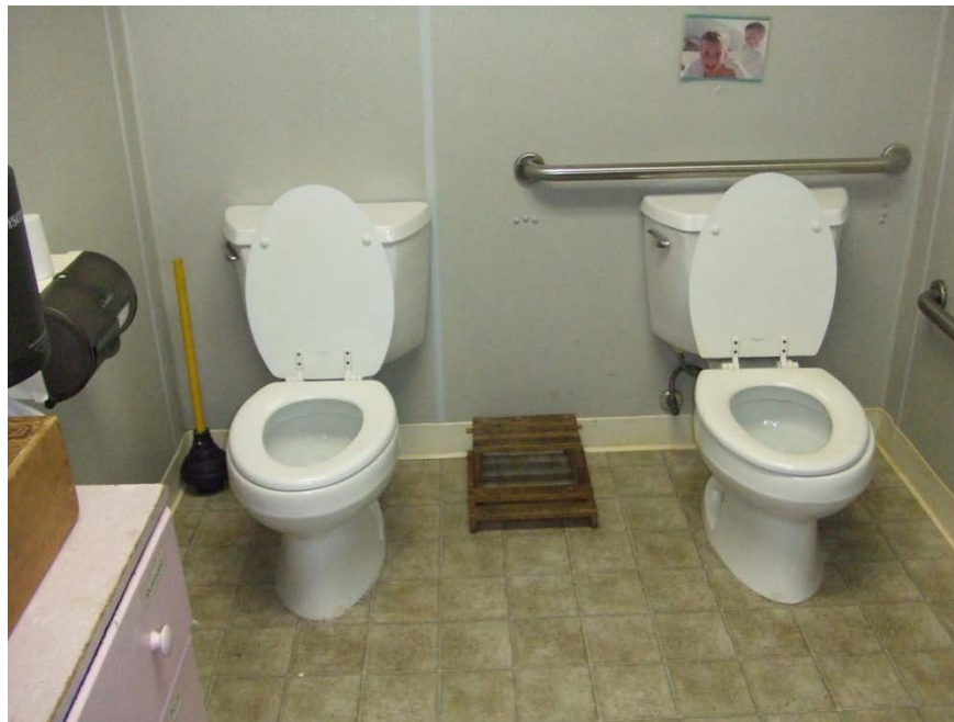
Photograph 16 – Taken at Fort Bragg on 4/1/10 showing adult-sized toilets in the children’s bathroom that did not have child-sized toilet seat adapters.
