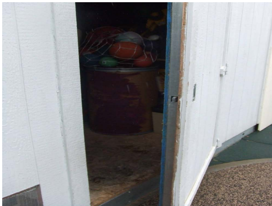
Photograph 25 – Taken at Low Gap on 4/2/10 showing an unlocked storage shed on the playground.
