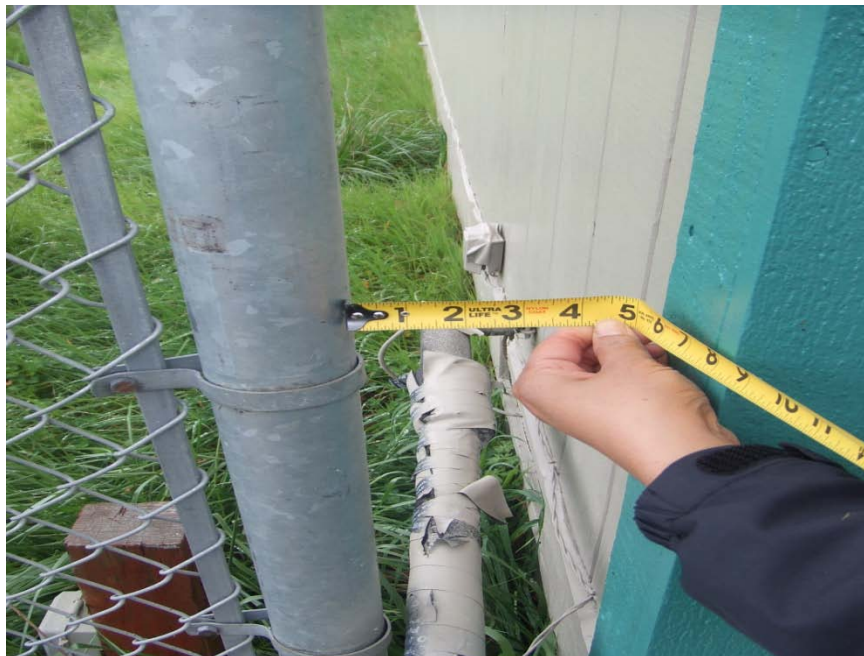
Photograph 8 – Taken at Willits Head Start on 4/1/10 showing a 5-inch gap next to the improperly secured gate shown in Photograph 7.
