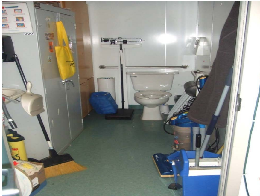
Photograph 6 – Taken at Willits Head Start on 4/1/10 showing an unlocked adult bathroom, which allowed children access to unsanitary and potentially hazardous materials and equipment (e.g., a vacuum, mop, and bucket containing dirty water).
