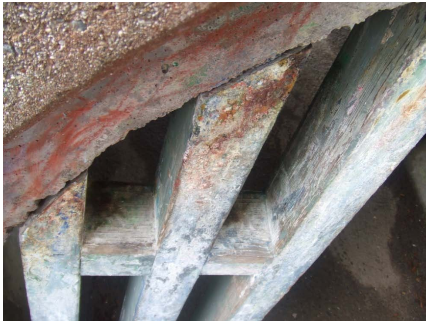
Photograph 12 – Taken at Willits Head Start on 4/1/10 showing mold and peeling paint on the wooden portion of a concrete play tunnel on the playground.
