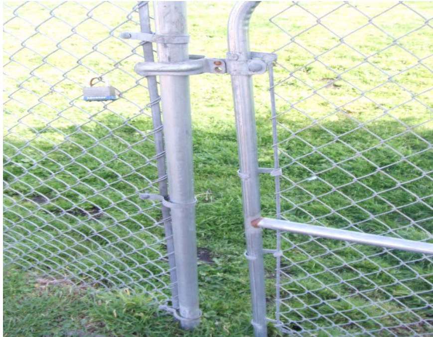
Photograph 21 – Taken at Fort Bragg on 4/1/10 showing an unlocked gate on the playground, which led to an unsupervised field. The gate latch was within children’s reach. The gate also had a 6-inch gap that a child could fit through.
