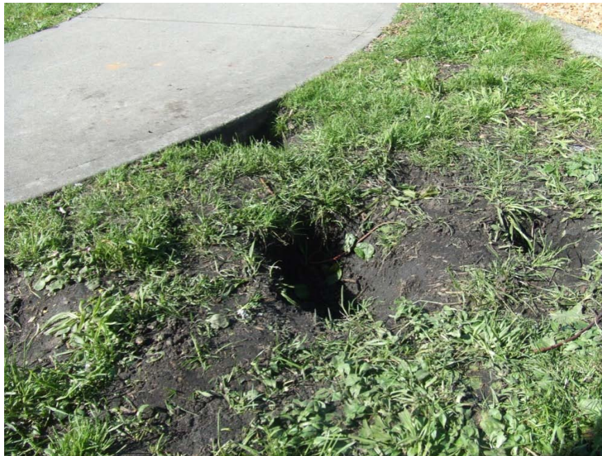
Photograph 22 – Taken at Fort Bragg on 4/1/10 showing deep holes on the playground, which were tripping hazards.
