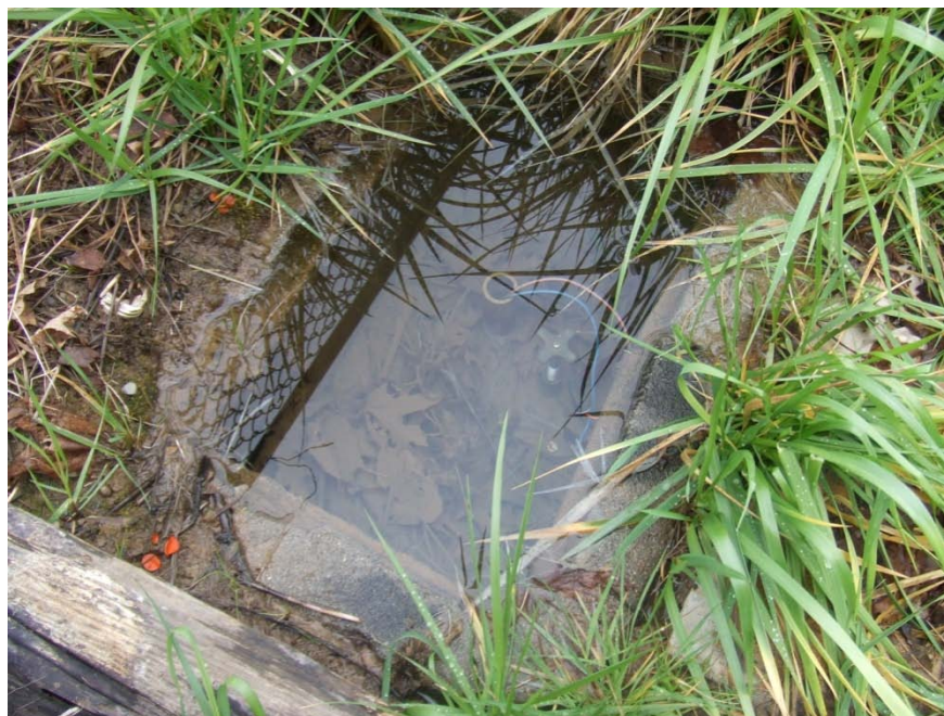
Photograph 9 – Taken at Willits Head Start on 4/1/10 showing a 16-inch-deep water-filled hole, which was a tripping hazard. The hole was located in an area accessible to children, approximately 10 feet beyond the improperly secured gate shown in Photograph 7.
