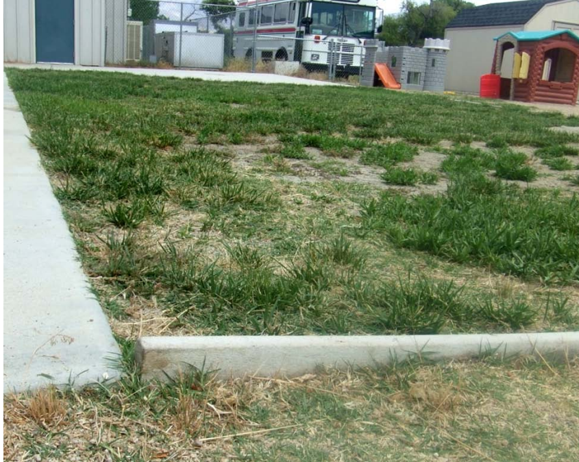
Photograph 3 – Taken at Little Promises on 6/3/09 showing one of two landscaping dividers on the playground protruding approximately 2 inches from the ground.
